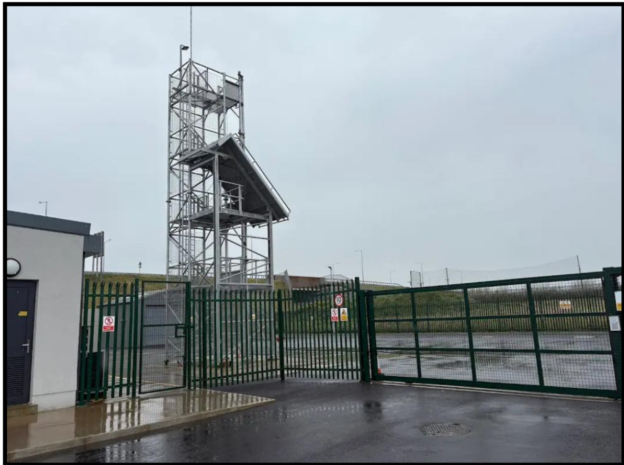
Plate 6.10 Looking Northwest from the South of the site area at existing infrastructure to the rear of the Fire Station
