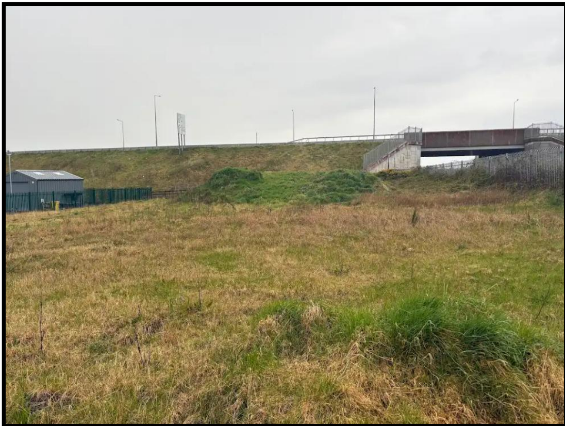
Plate 6.6 Looking West from the East of the site
