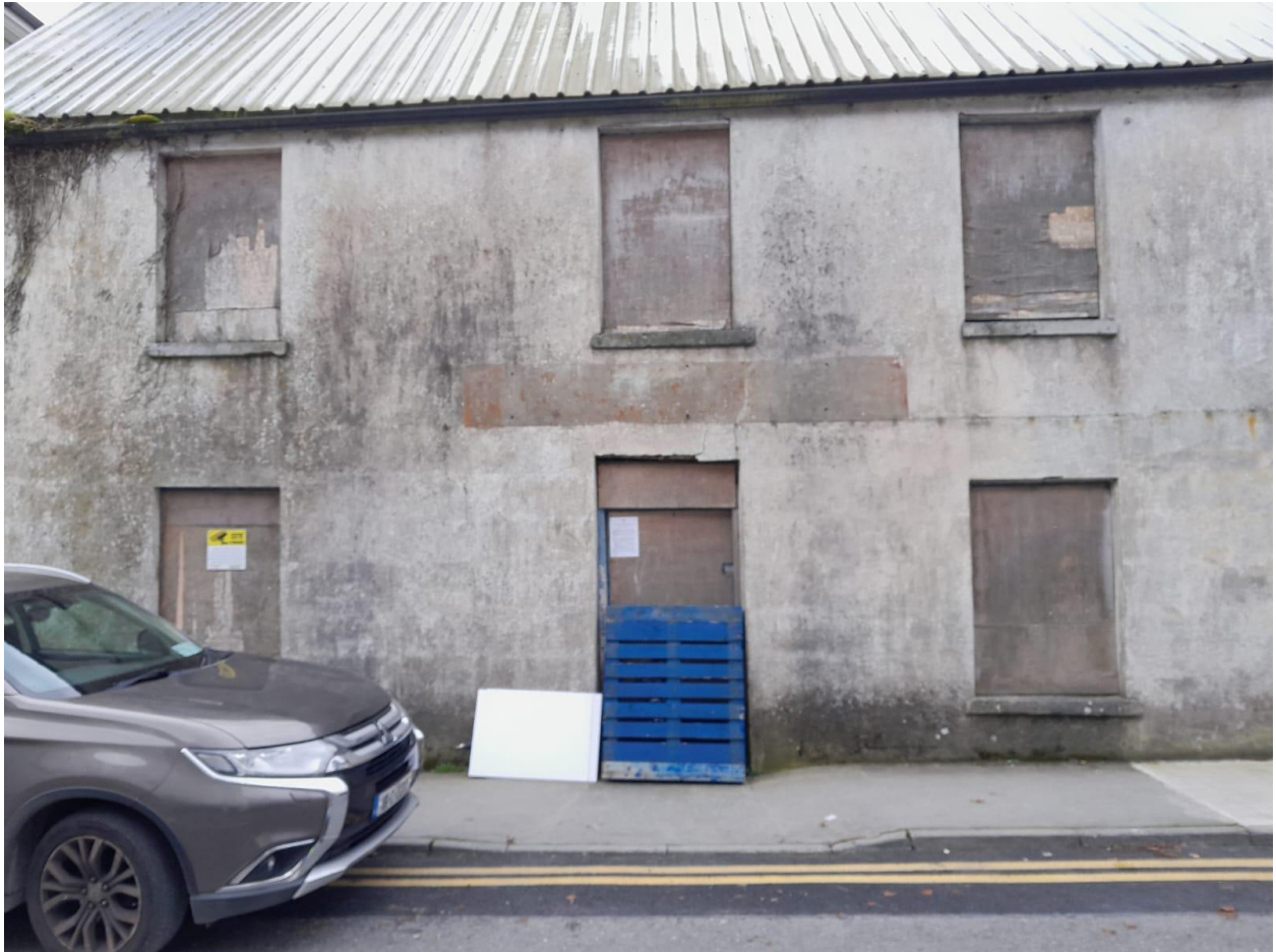
Photograph 2: Site notice in position on front entrance
