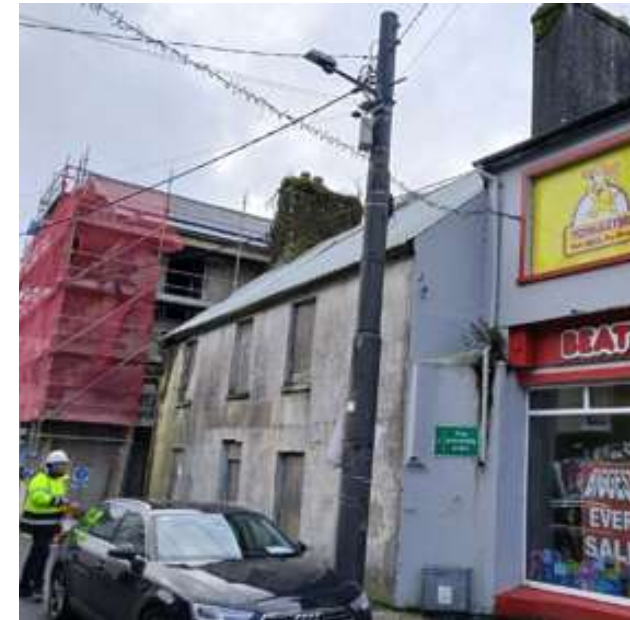
Fig.17: View from Church Street
