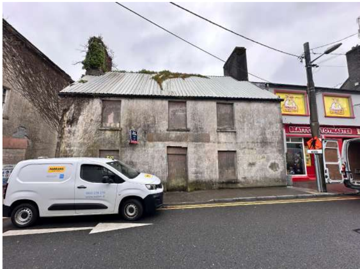
Fig.3: View from Church Street
