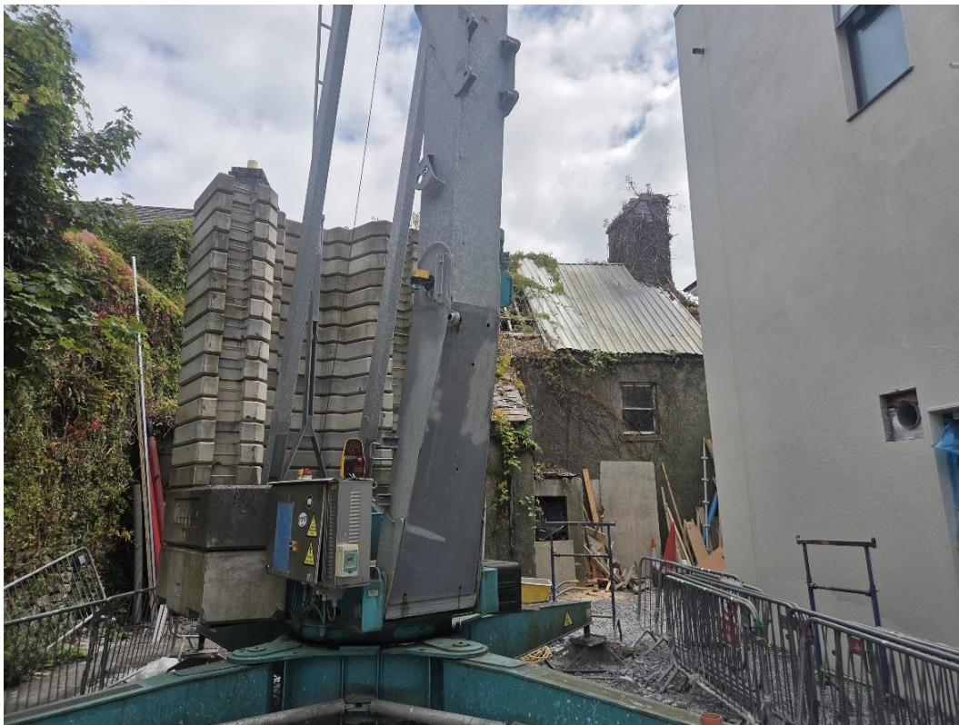
Plate 3-3: Rear of building
