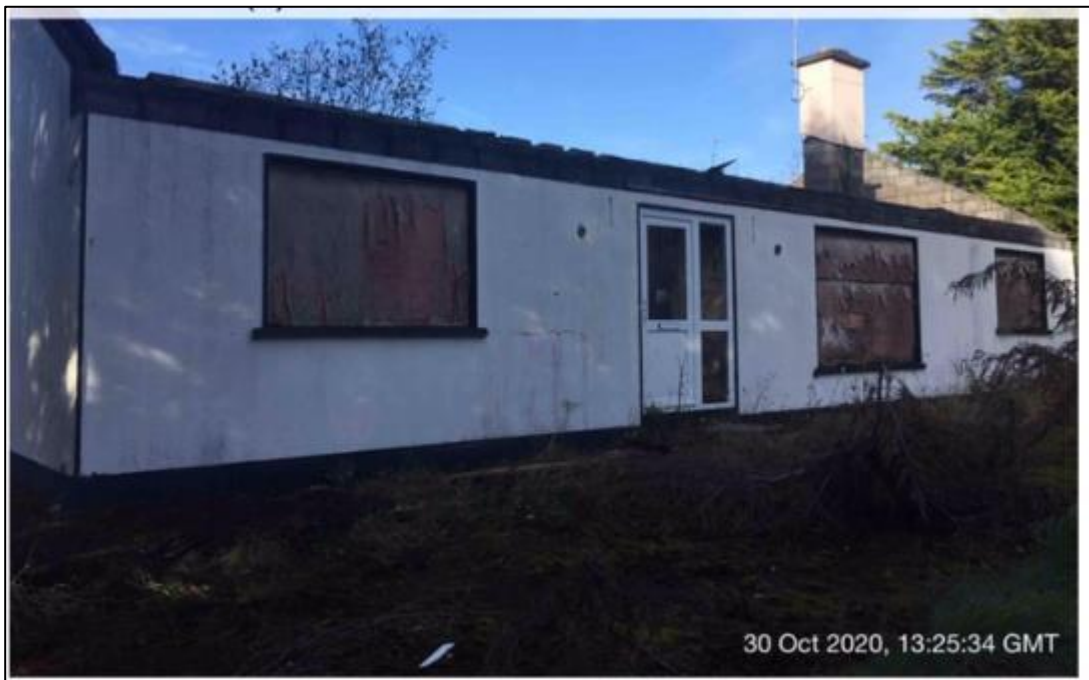
Photograph 2: Front Elevation of The Existing Dwelling taken from within the site
