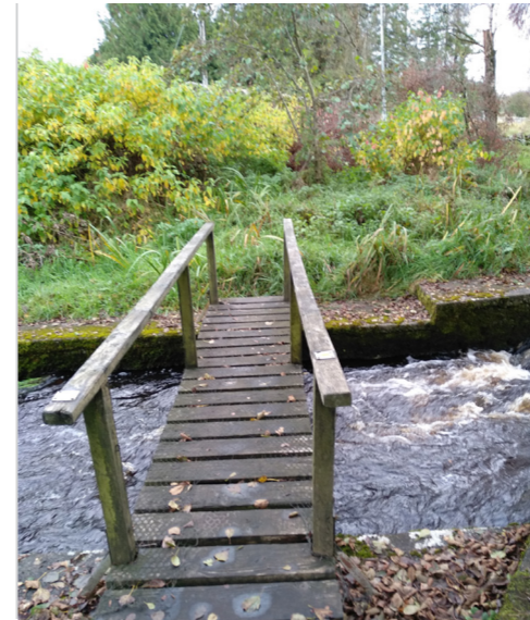
BRIDGE CROSSING THE DERRYHIPPO RIVER IN CREGGS WILDLIFE PARK.
