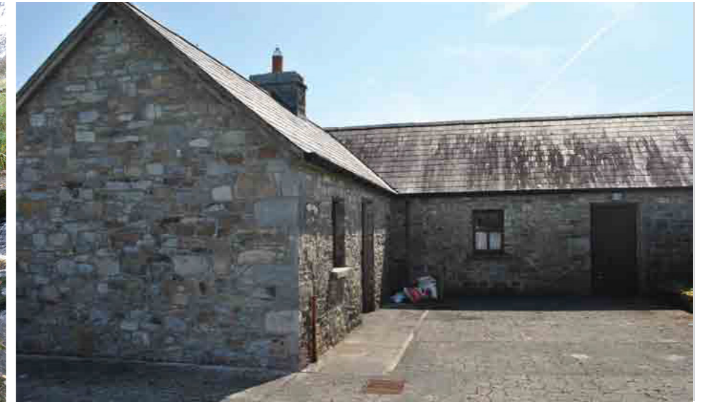
CHARLES STUART PARNELL HERITAGE CENTRE LOCATED ALONG THE MAIN STREET OF CREGGS VILLAGE.
