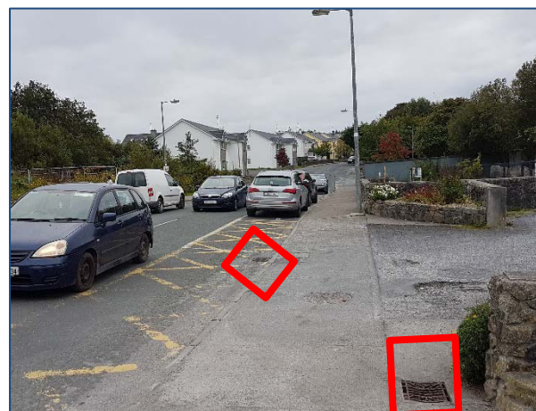
Plate 2-4 L1320 Existing Drainage
