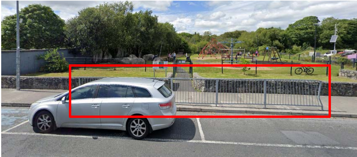
Plate 2-5 L1320 Pedestrian Guardrail adjacent to Playground
