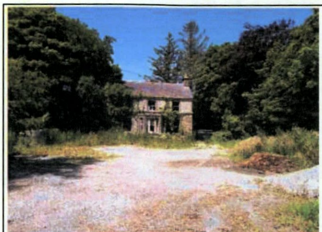
Photograph 2: Front Elevation of The Existing Dwelling taken from within the site
