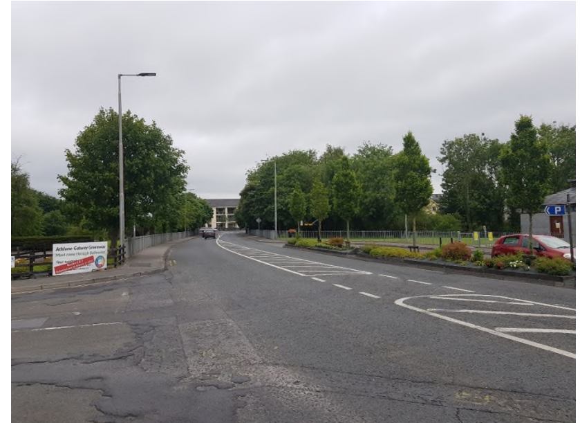
Figure 33. R446 (Marina) Facing North
