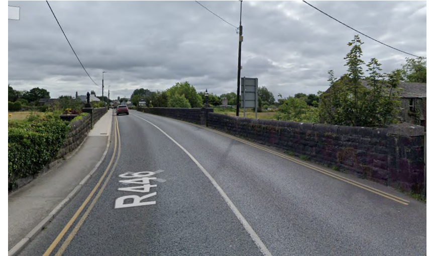
Figure 36. Bridge Street (Facing East)
