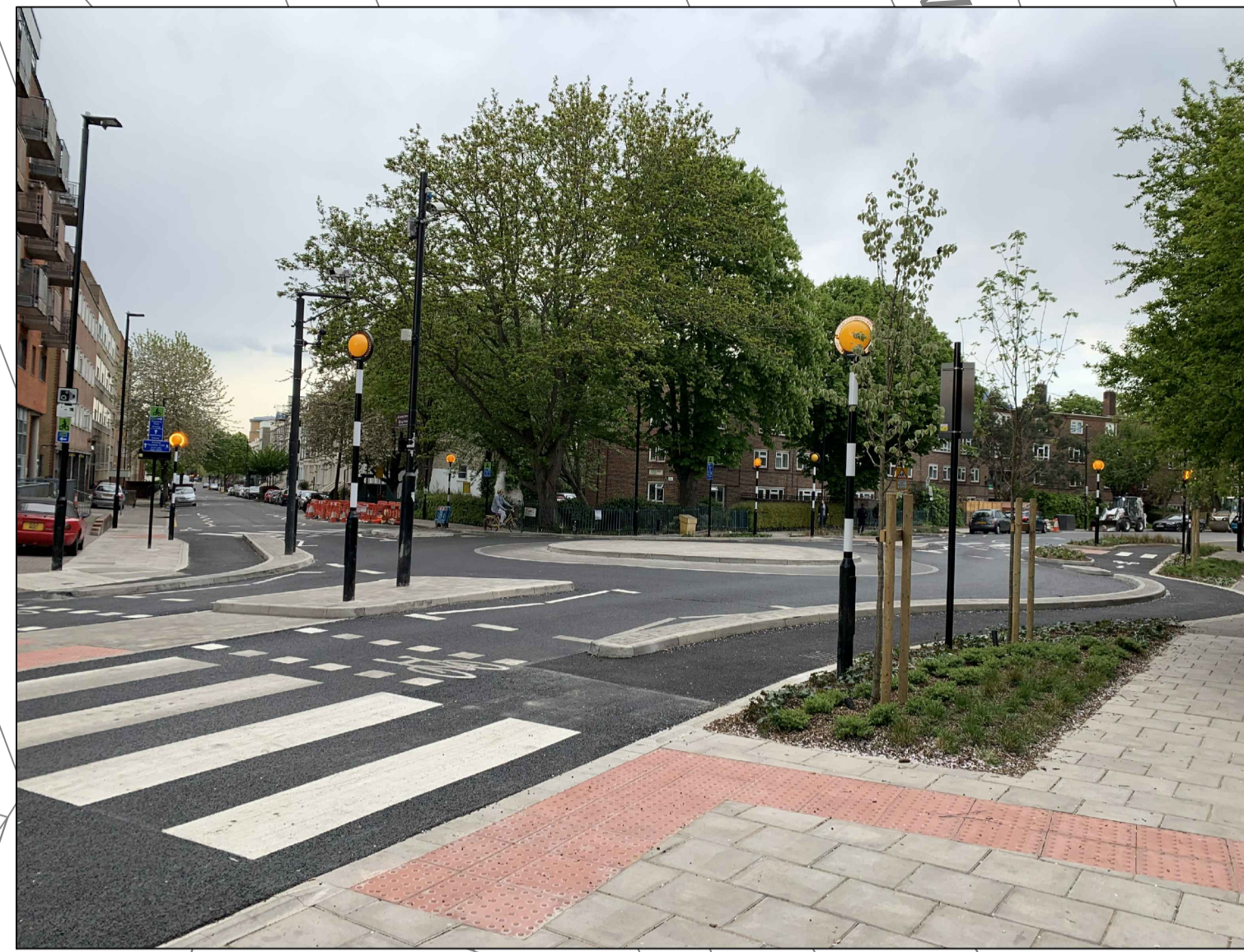
Benwell Roundabout, Islington, London - Flush crossing and raised table
