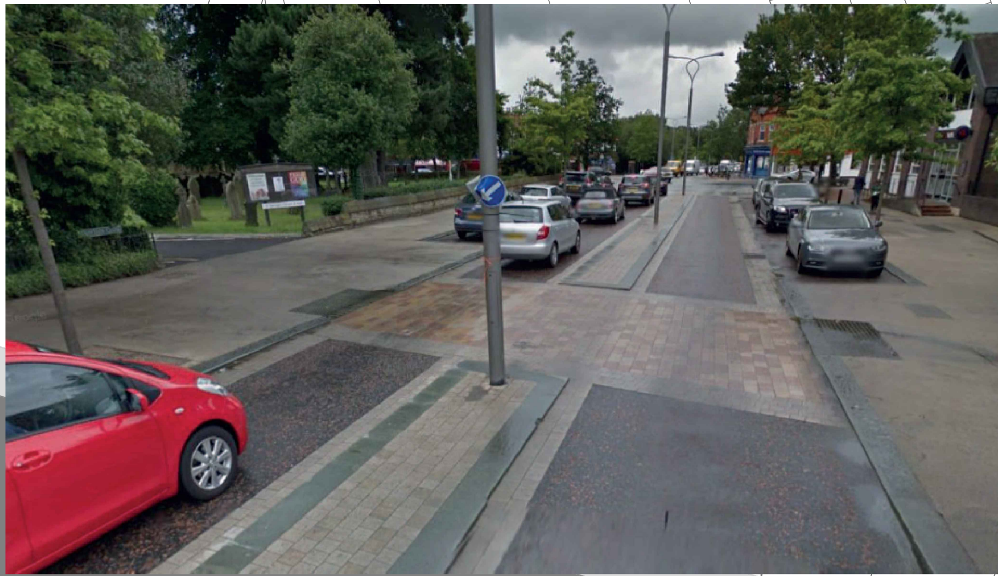
Poyton, cheshire - Informal pedestrian crossing point
