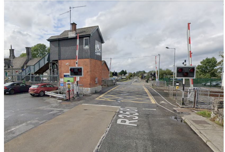
Figure 38. Ballinasloe Station (Facing North)
