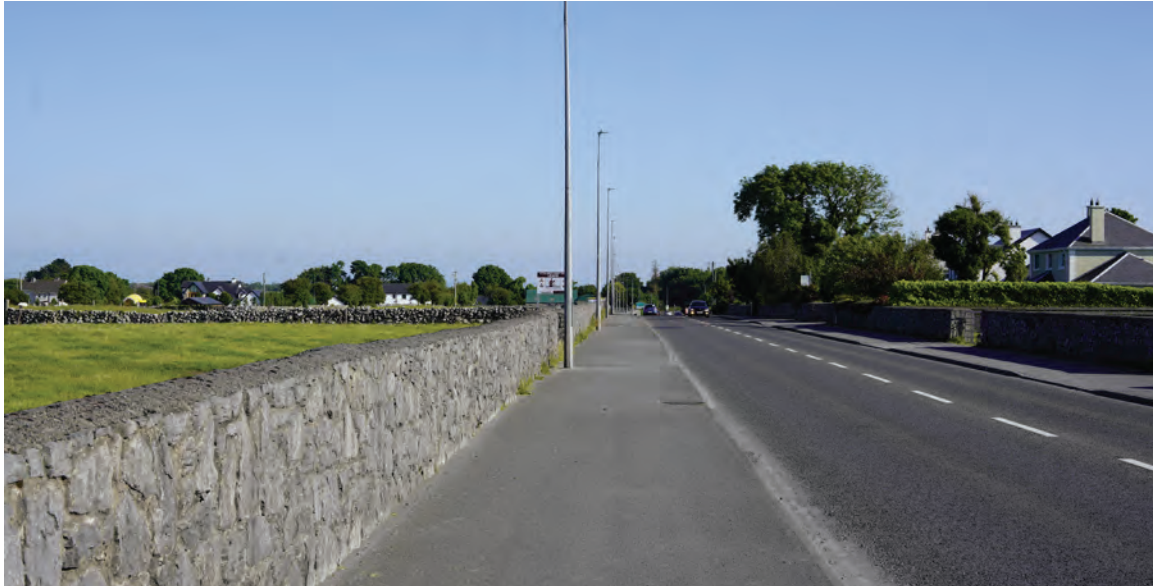
Parkmore Rd looking south
