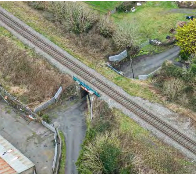
Stone bridge at L71051
