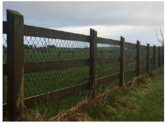
Picture of the post and rail fence proposed for use where noted on the drawing.
