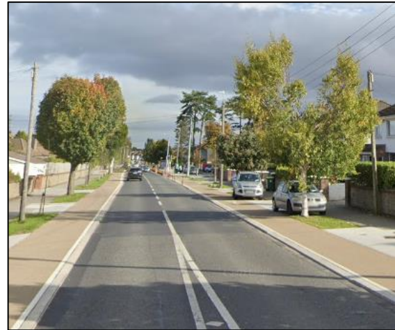
Figure 5-2: Example of a Segregated Cycle Track
