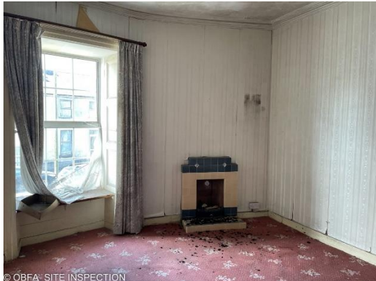
Existing timber shutters, skirtings, fireplace, cornices
