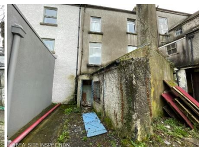
Extensions to rear of 3 storey structure
