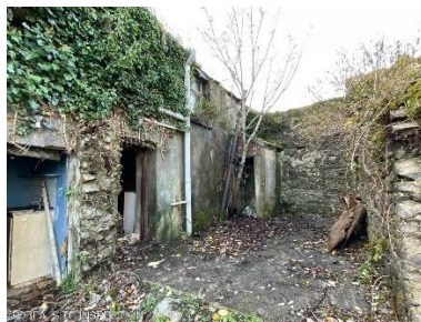
2 storey terrace facing west
