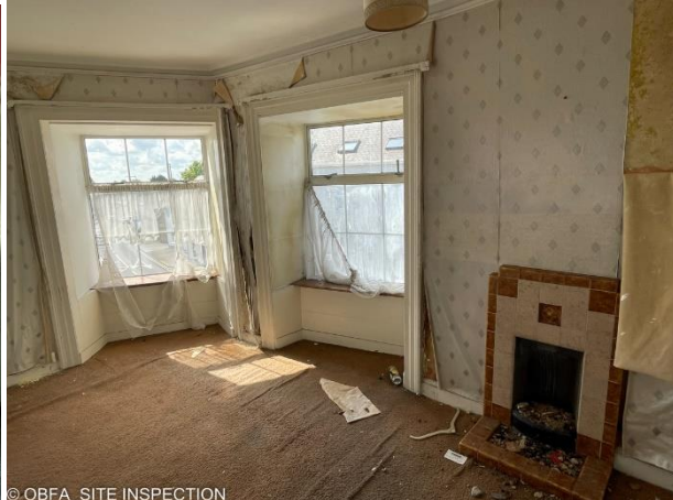
Existing timber shutters, skirtings, fireplace, cornices
