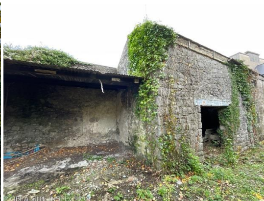
Existing stone shed
