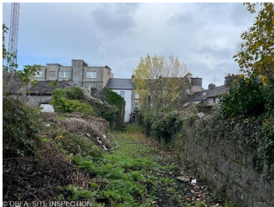
Existing stone wall sub-dividing site
