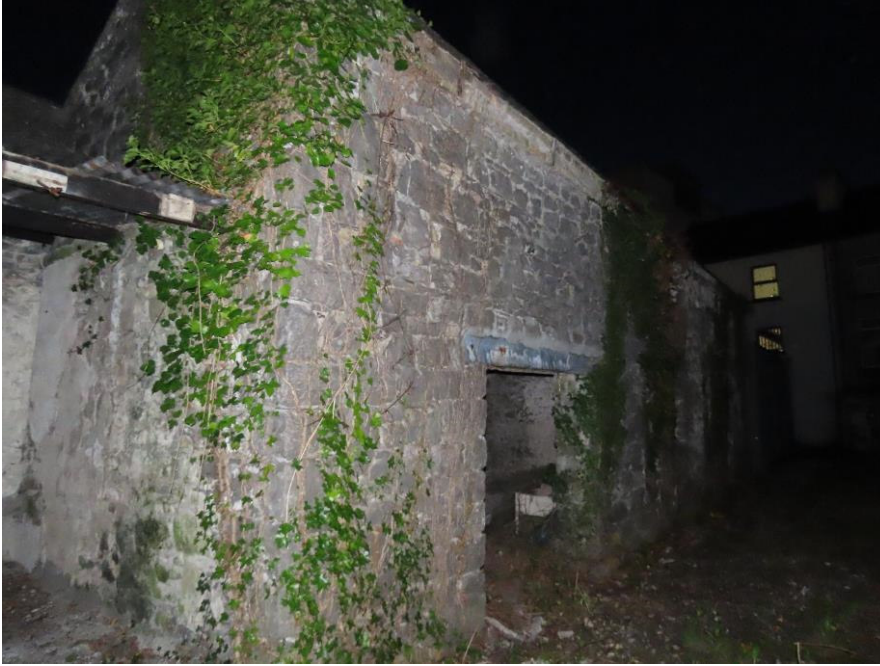
Photo 67 – dusk survey conducted at stone outbuildings to rear of Property 9
