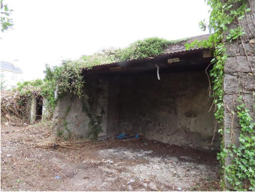
Photo 63 – lean-to building attached to stone outbuilding
