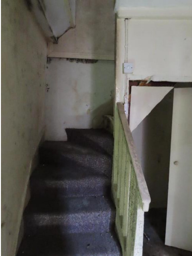
Photo 35 – stairs in Property No 6
