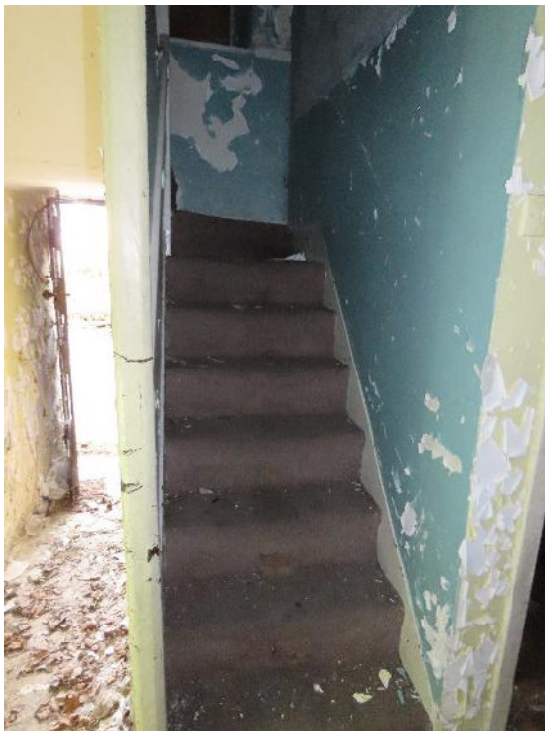
Photo 31 – stairs in Property 4
