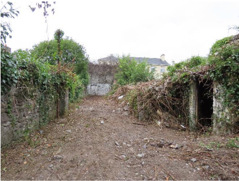
Photo 64 – looking west towards rear boundary wall
