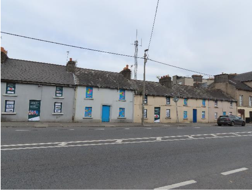
Photo 3 - Properties 3 - 7 in Dunlo Hill terrace – front elevation
