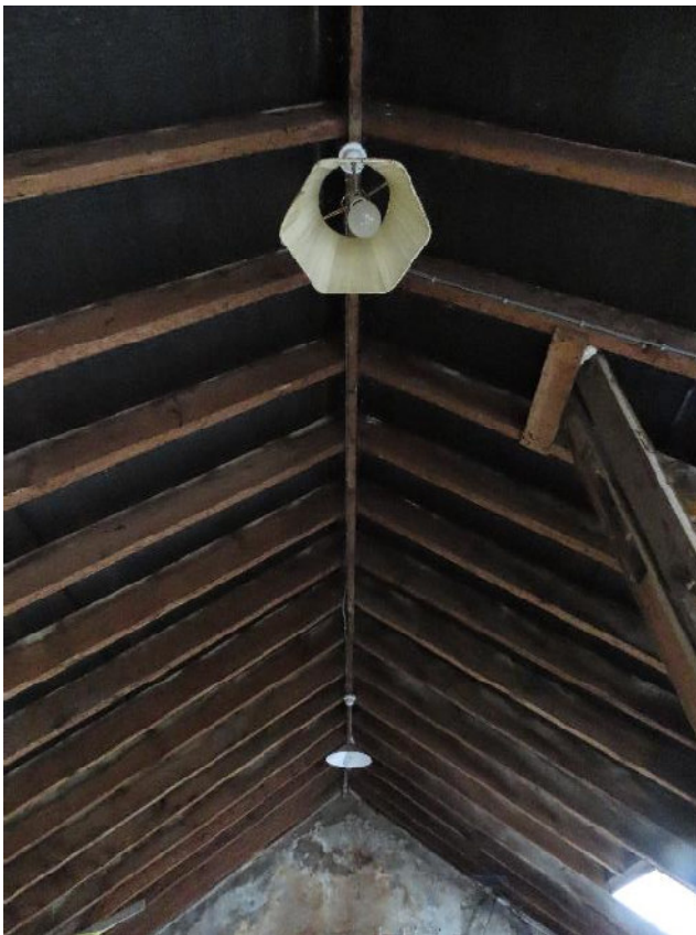
Photo 60 – exposed timbers in attic space – no evidence of bats
