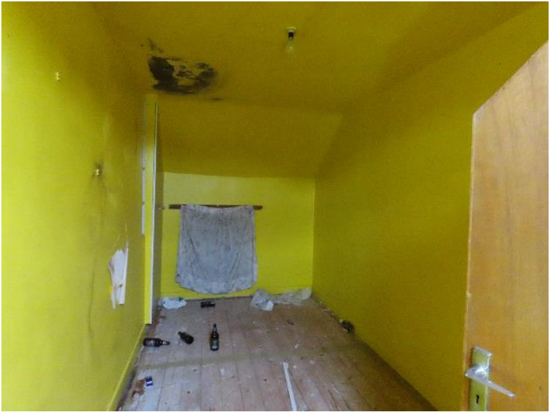
Photo 26 - Upstairs bedroom in property 3
