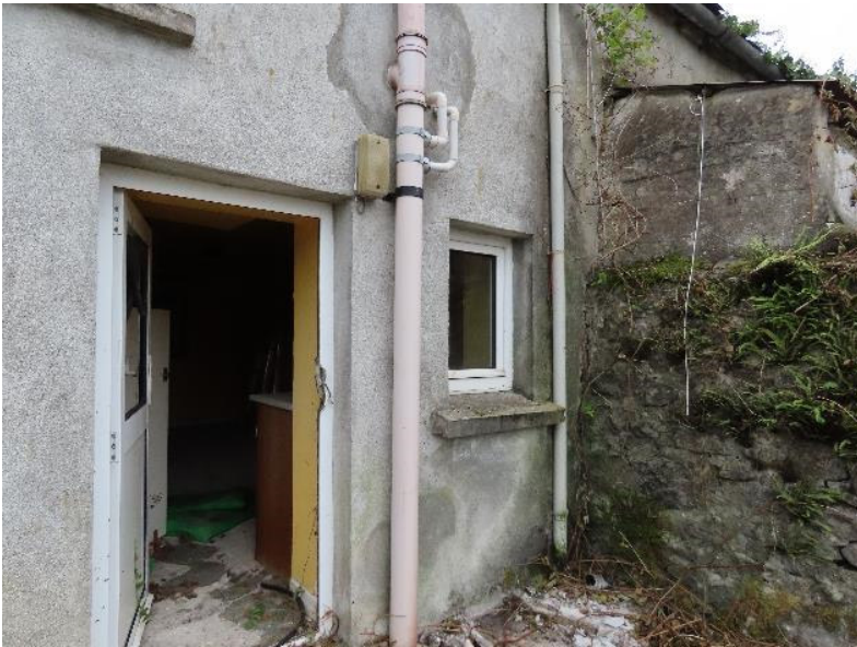
Photo 25 - Rear door of Property 3
