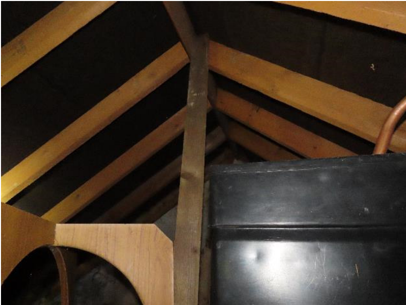
Photo 28 - Attic space of Property 3 showing bitumen lining on inside of slates
