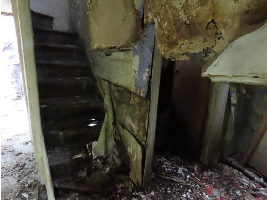
Photo 41 - Stairs in Property 7
