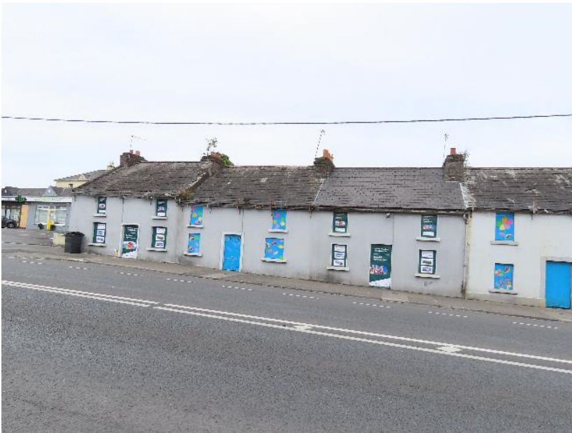
Photo 2 - Properties 1- 4 at western end of Dunlo Hill terrace
