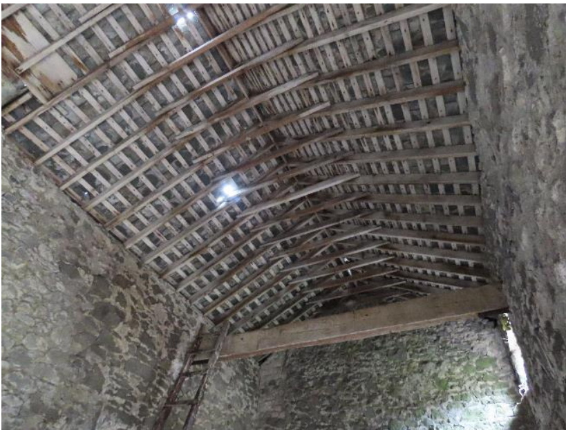
Photo 62 – exposed roof timbers in outbuilding
