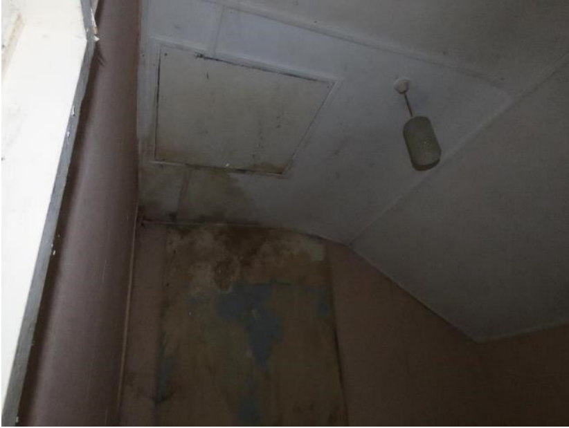
Photo 37 – trap door to attic of Property 6
