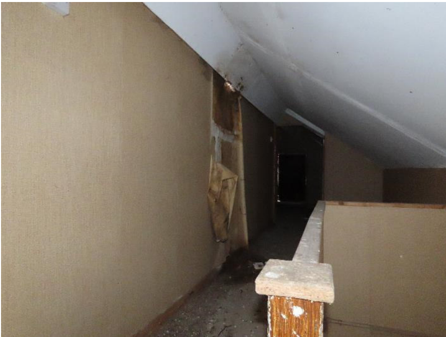
Photo 46 – upstairs landing of rear section of building
