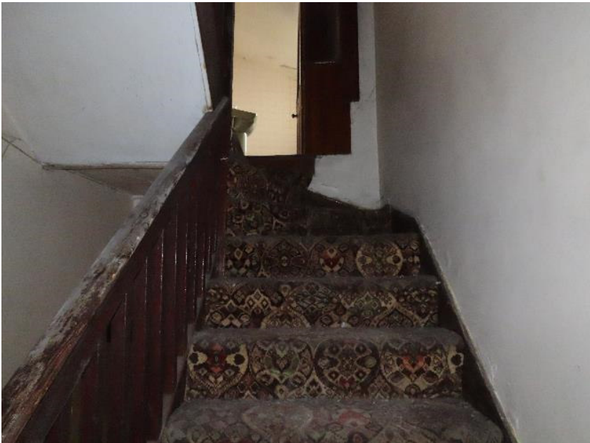
Photo 48 – stairs to attic rooms
