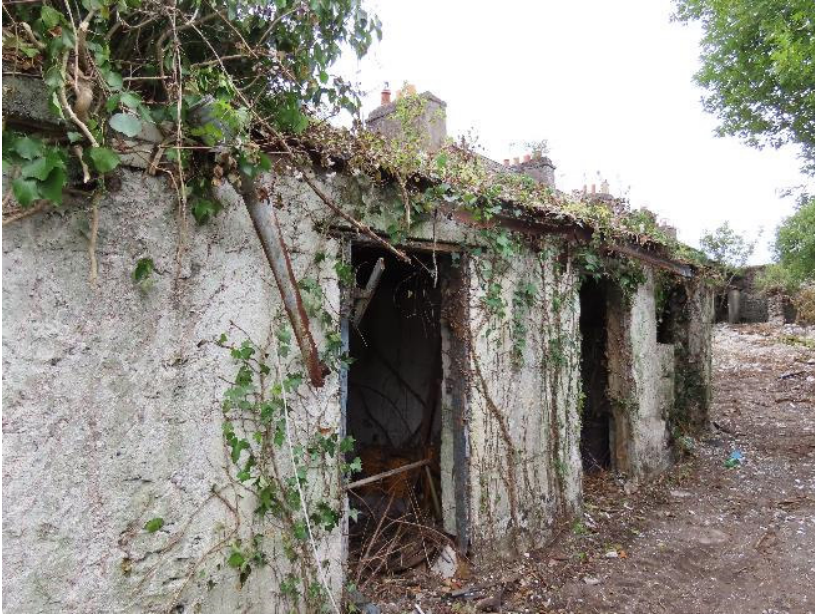
Photo 12 - Stone outbuildings to rear of Dooley's pub
