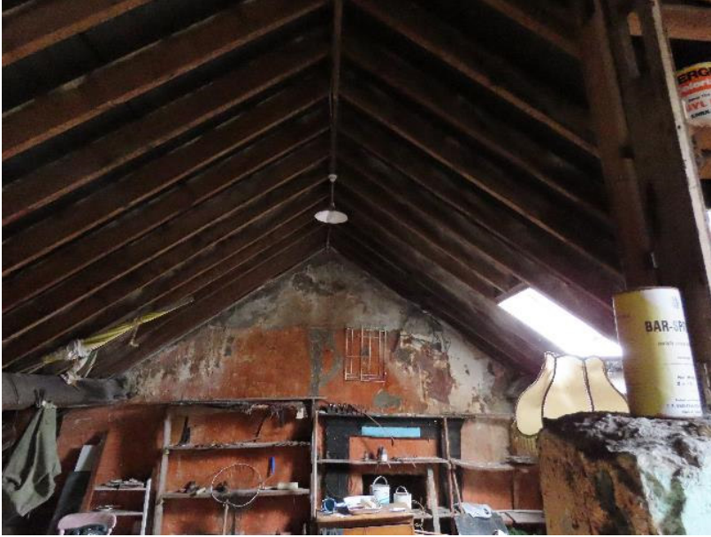
Photo 59 – attic space being used as work space/ storage space
