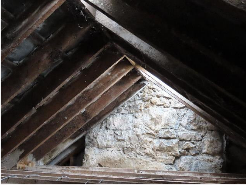
Photo 22 - Attic space of Property 1
