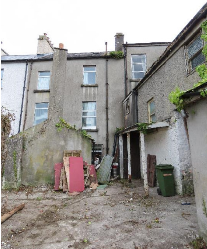
Photo 10 - Rear of Dooley's Pub and Property No. 9
