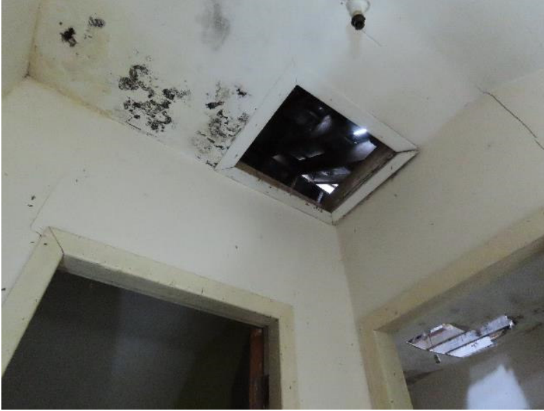
Photo 20 - Access to attic space of Property 1 via trapdoor in upstairs ceiling
