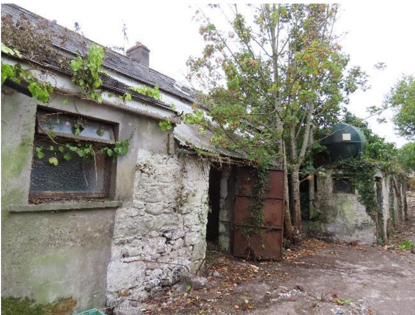
Photo 11 - Stone outbuildings to rear of Dooley's pub
