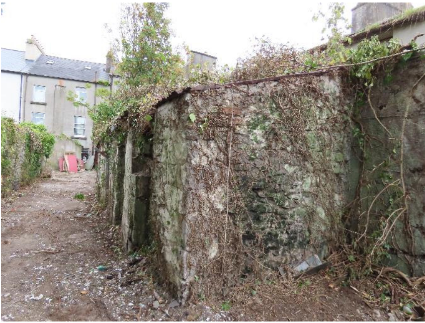
Photo 42 - Sheds to rear of Property 5, 6 & 7
