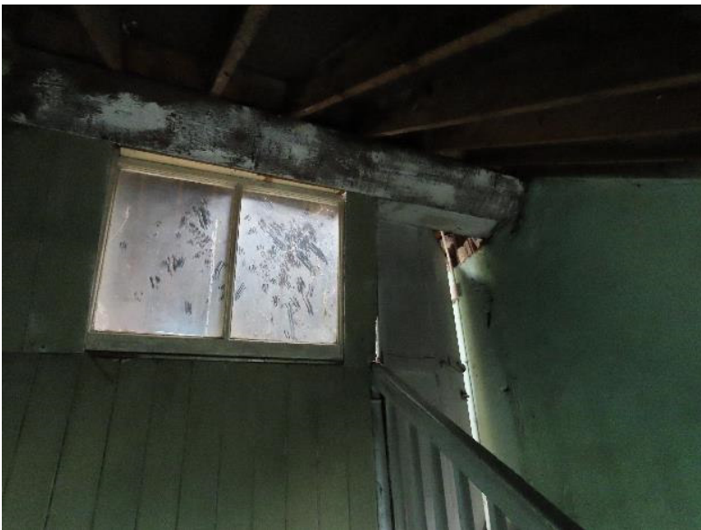
Photo 58 – stairs to attic space
