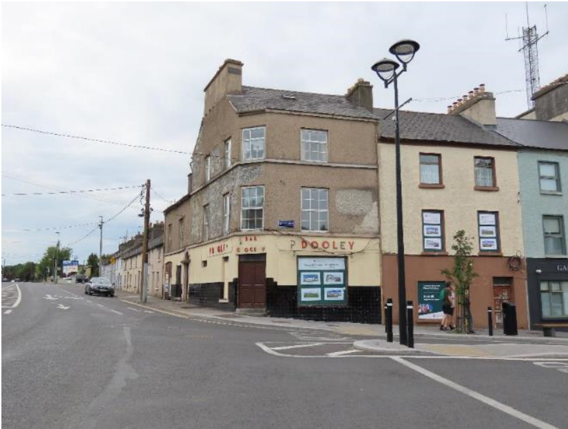
Photo 8 - Dunlo terrace to rear of Dooleys Pub, Dooley's Pub and Adjoining 3 storey building
