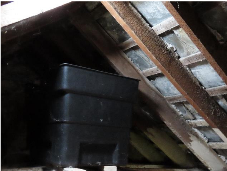
Photo 23 - Attic space of Property 1 showing original slates
