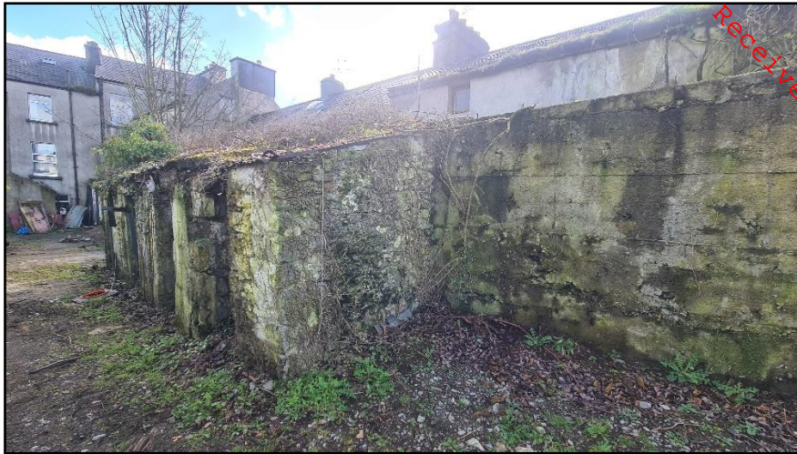
Plate 15 Facing E showing extensions to rear of terraced dwellings
