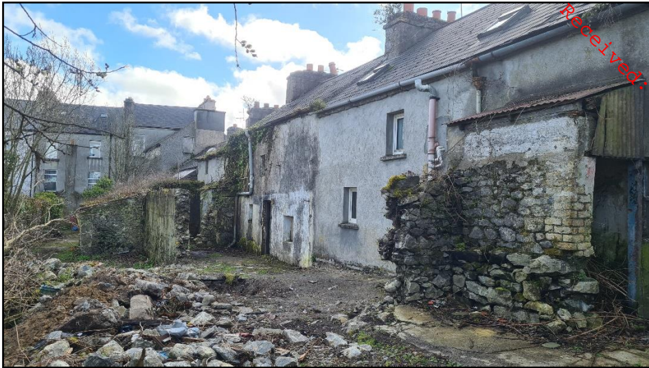
Plate 12 Facing SE showing rear of terraced dwellings
