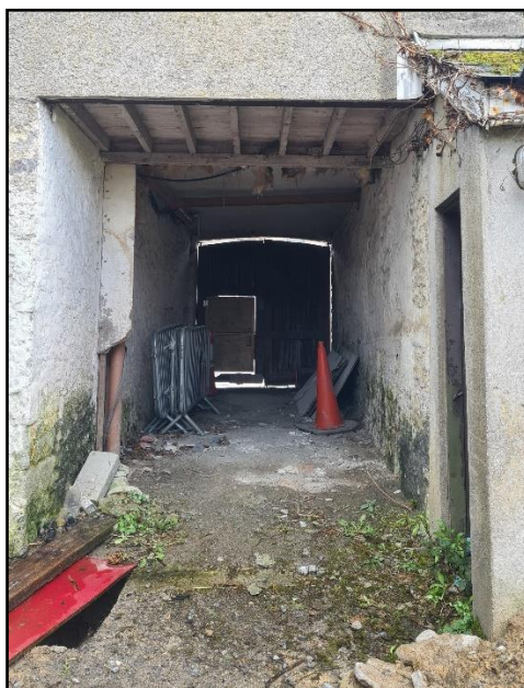
Plate 17 Facing N showing archway in the SE extent of site
