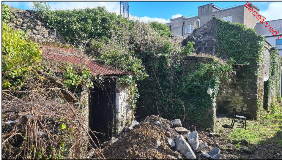
Plate 6 Facing E showing outbuildings abutting N boundary wall
