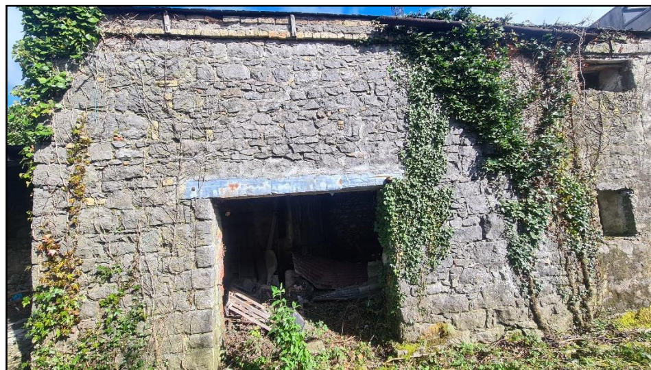
Plate 8 Facing N showing stone outbuilding abutting N boundary wall
