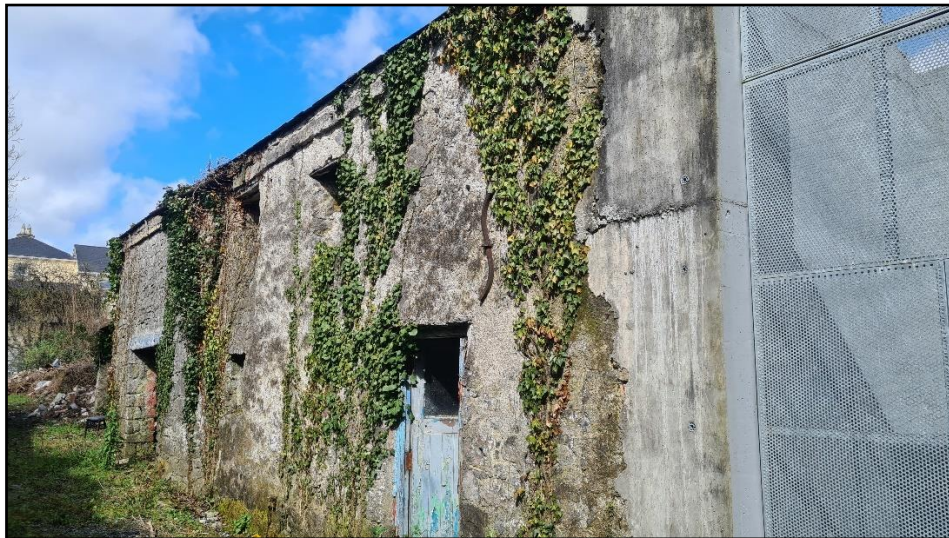
Plate 7 Facing W showing outbuildings abutting N boundary wall
