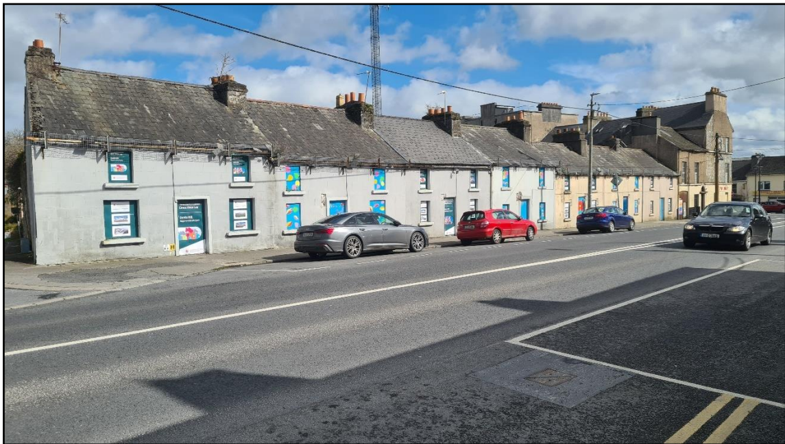
Plate 2 Facing NW showing development site façade at Dunlo Hill
