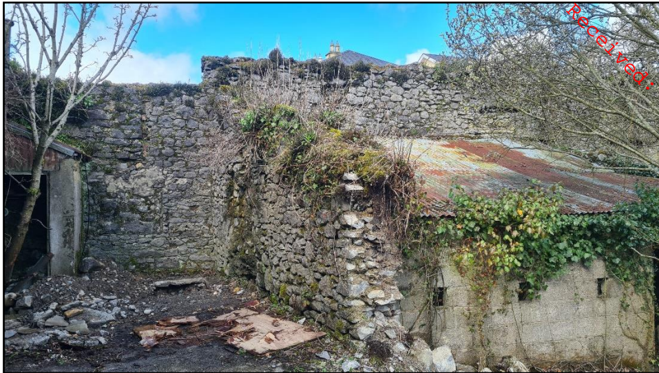
Plate 9 Facing W showing outbuilding abutting W boundary wall
