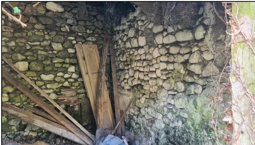
Plate 16 Interior of extension (seen in plate 15) showing rubble-built walls
