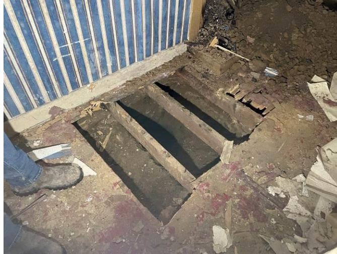
Photograph 30: Example of suspended timber floor within one of the residential units
