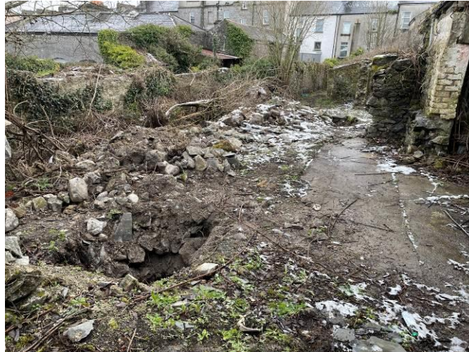
Photograph 1: Locations of trial holes at rear right side of the site
