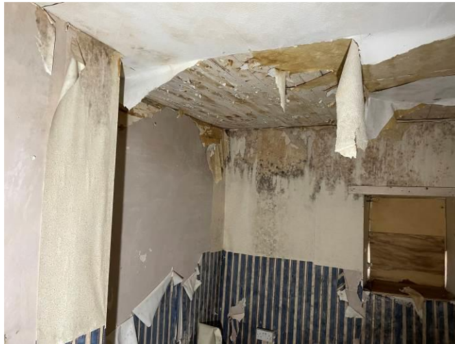
Photograph 24: Typical condition of the ceilings within the residential properties
