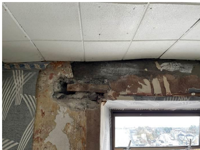
Photograph 12: Timber lintel within the public house part of the property
