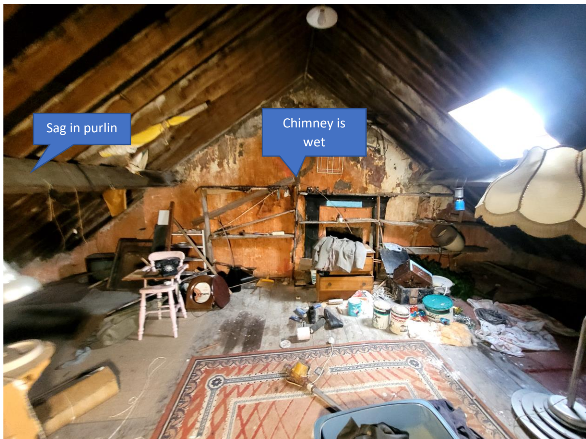
Figure 6. Shows a broad view of the attic space.
