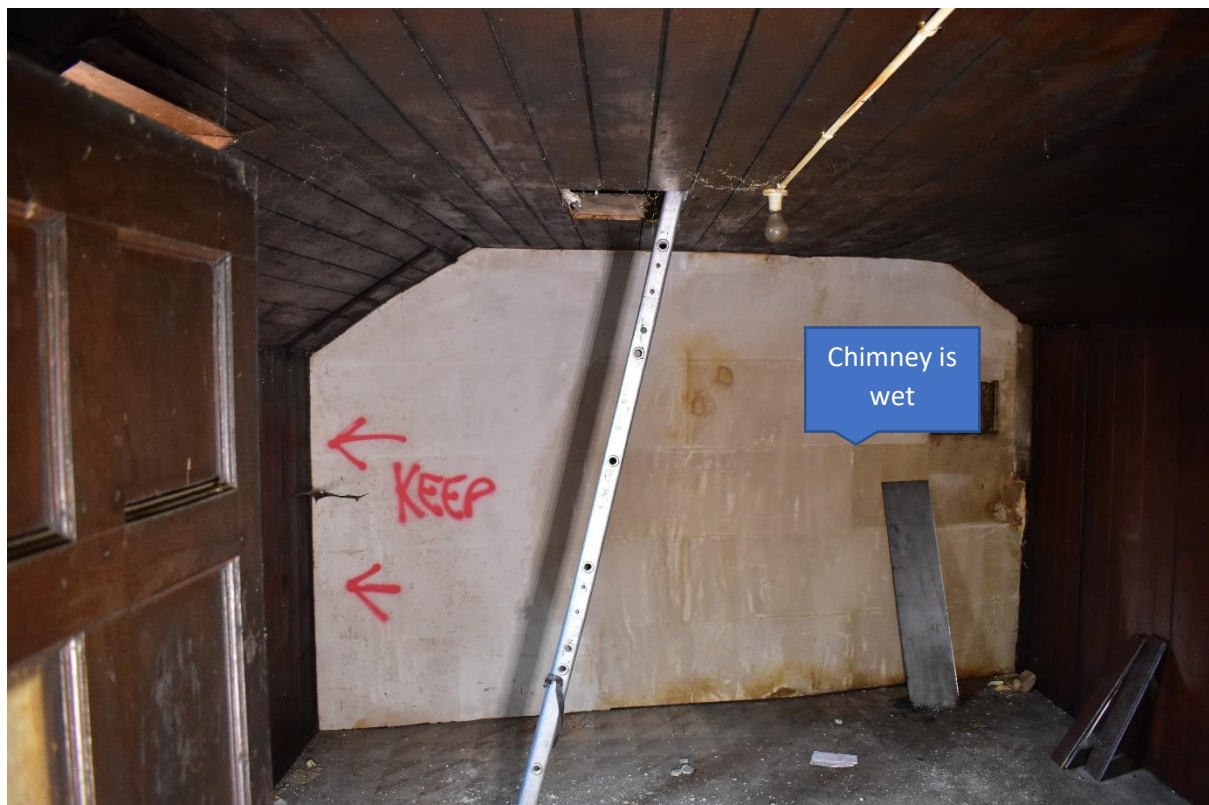
Figure 16. Shows the broad view of the attic room in Dooley's Pub.
