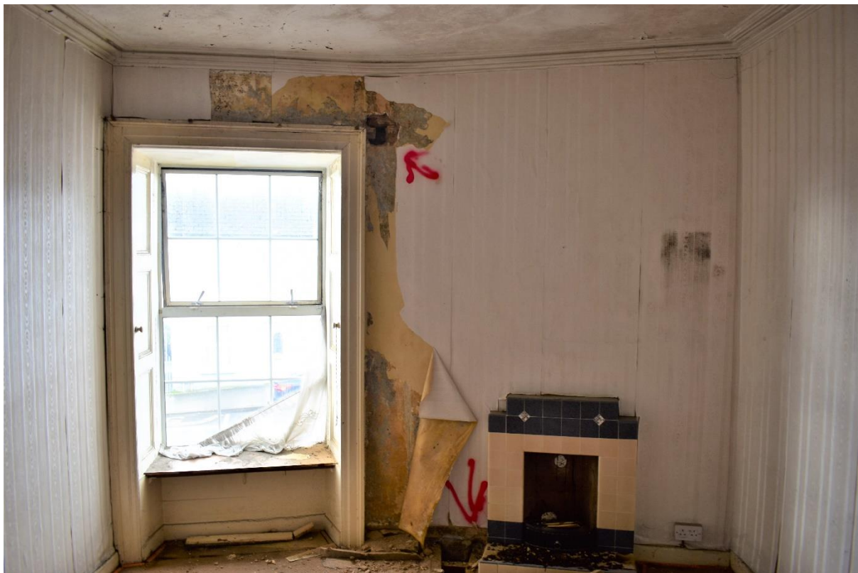
Figure 14. Shows pockets exposed on the Dunlo Hill elevation.
