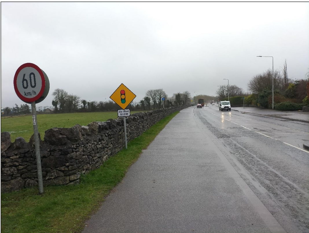
Plate 5-8 R381 located west of the site.
