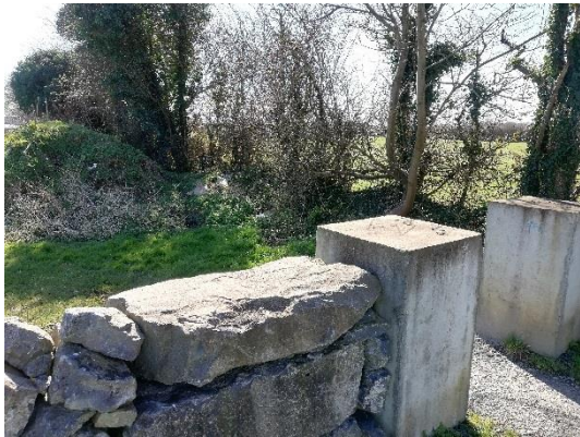
Eastern site boundary with GAA; access shown is from Cuairt Na hAbhainn to GAA
