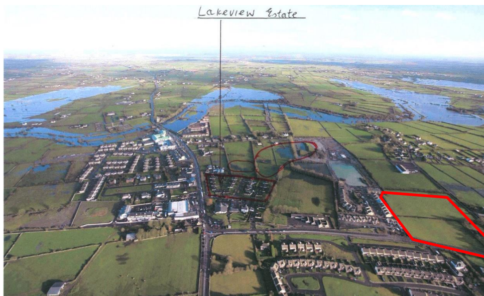
Figure 3-2 Lakeview flooding December 2006
