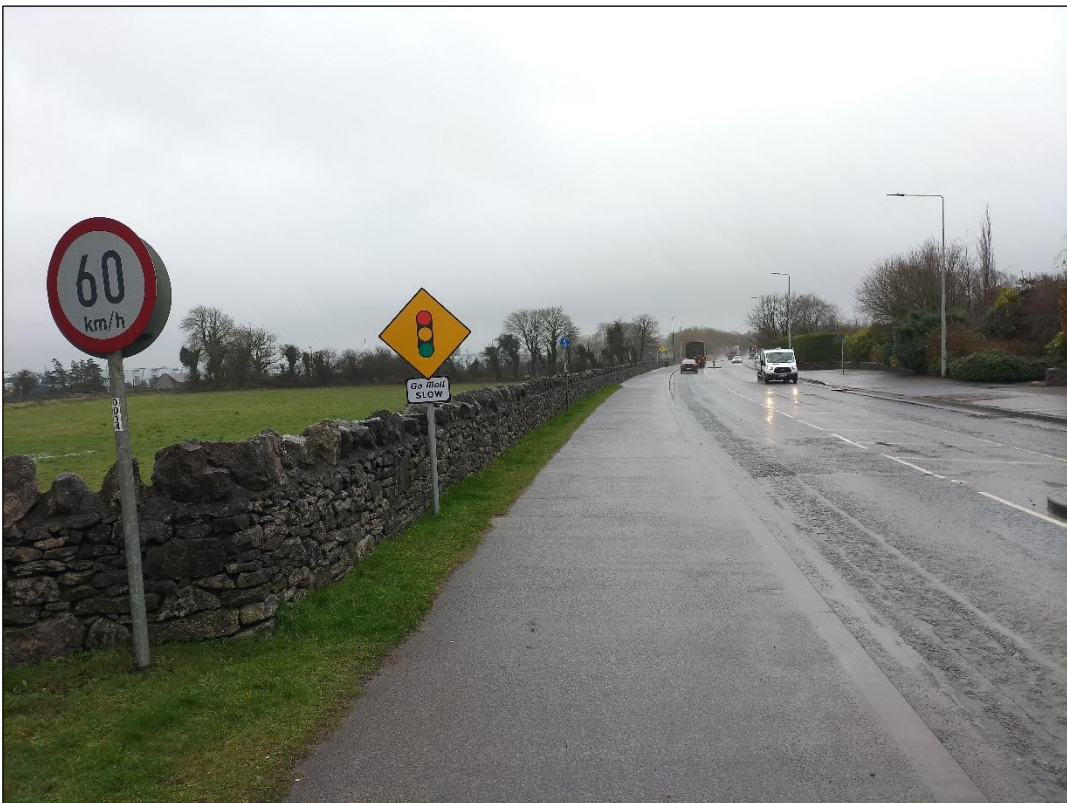
Plate 2-9 R381 located west of the site.
