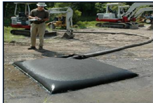
Plate 3-2 Silt Bag under inspection
