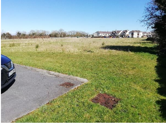
Looking north-east along route of culverted pipe in Cuairt Na hAbhainn
