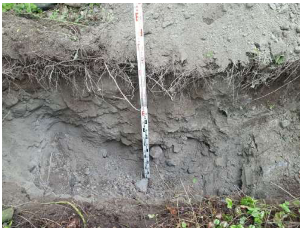
Trial Pit dug to 1.5m deep 02-07-2020, water ingress noted at base of Trial Hole.
