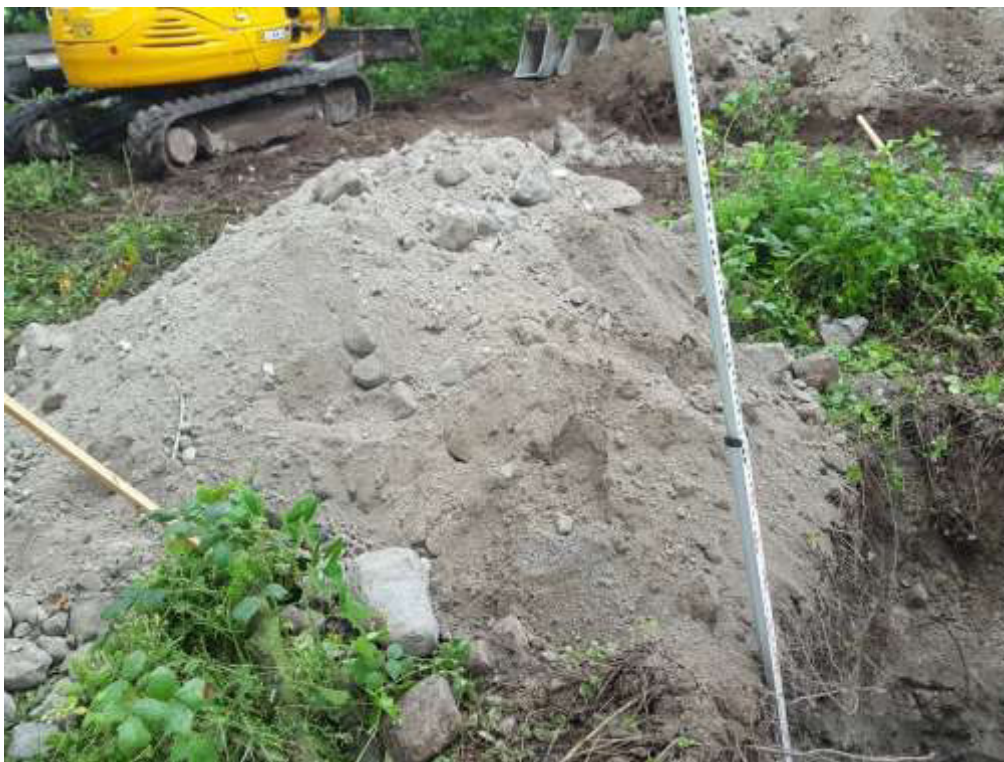
Trial Pit spoil dug to 1.5m deep 02-07-2020.
