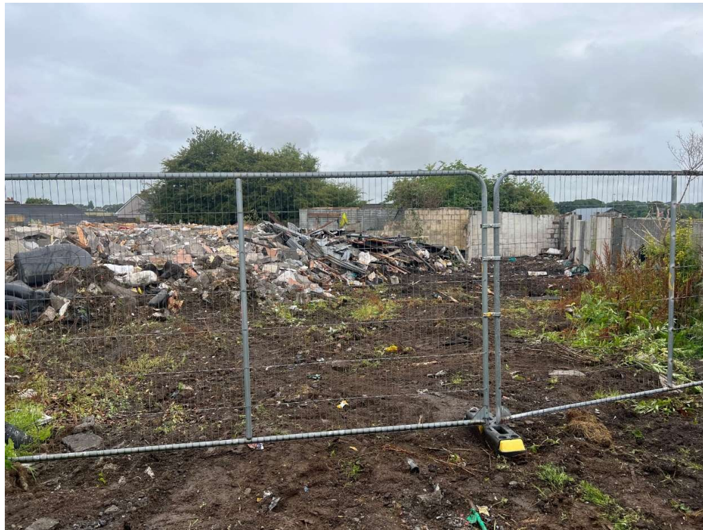
Figure 9 - Site following demolition of dwellings.
