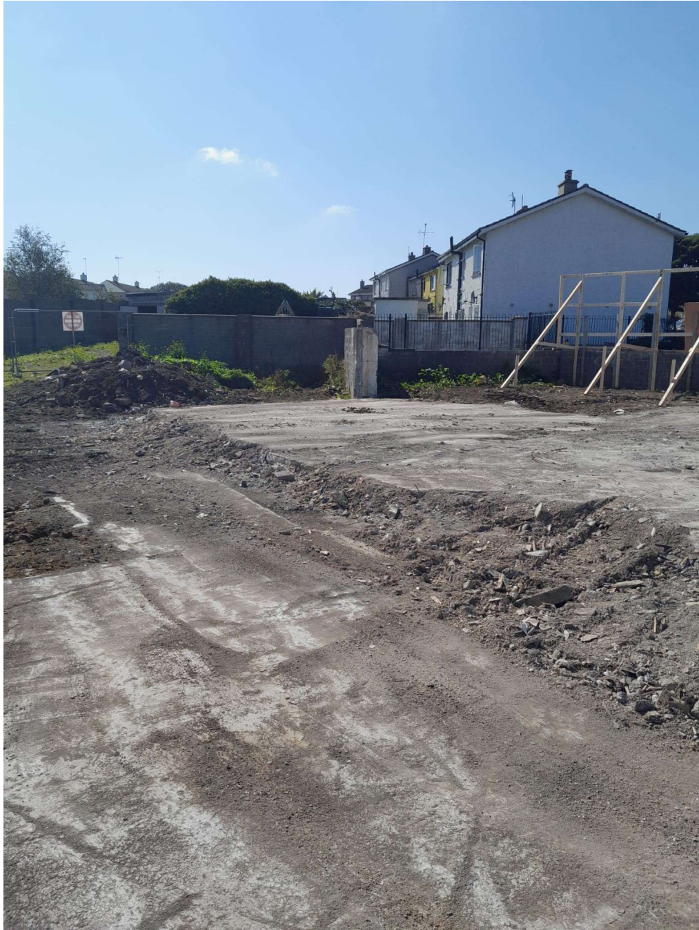
Figure 10 - Site cleared looking towards South West
