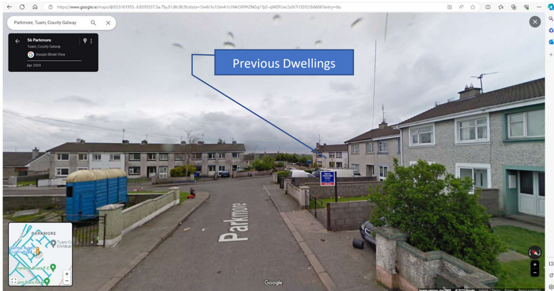
Figure 8 - South Approach to Site showing 2 no. previous dwellings.
