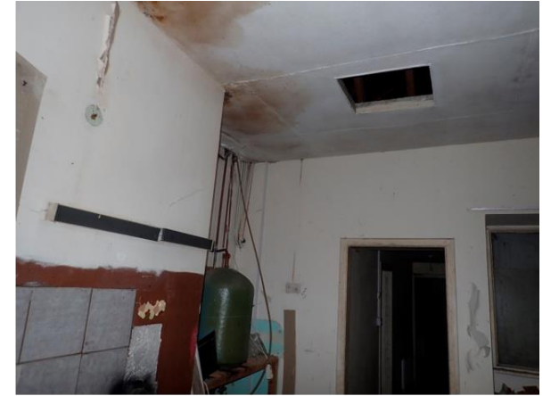
Plate 7: View of loft hatch during March 2024 survey
