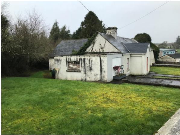
Plate 1: View of dwelling looking north
