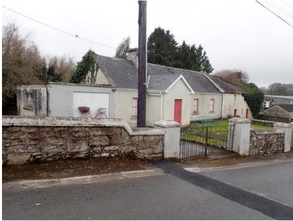
Plate 7: View of dwelling during March 2024 inspection survey
