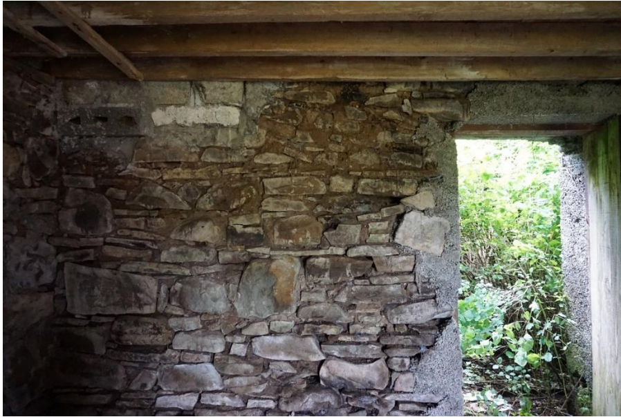
Photograph 11 - Outbuilding Rear Interior Sandstone Wall
