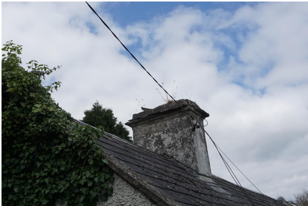
Photograph 2 - Chimney from Southern Side
