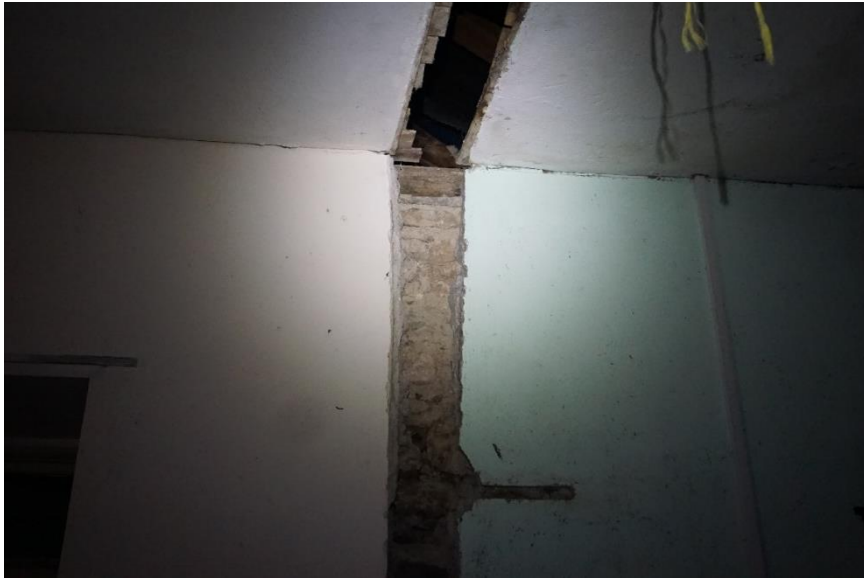
Photograph 5 - Cementitious Render on Original Stone Wall in Living Room
