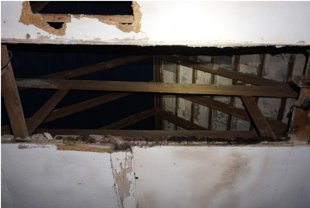
Photograph 7 - Modern Plaster Board Ceiling in Living Room
