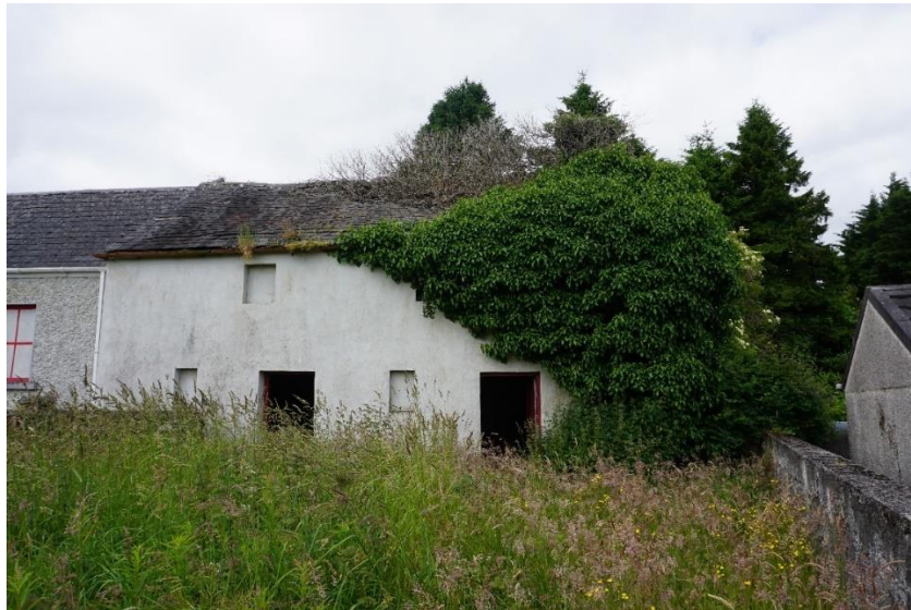
Photograph 9 - Front Elevation of Outbuilding Showing Roof and Obscured Chimney
