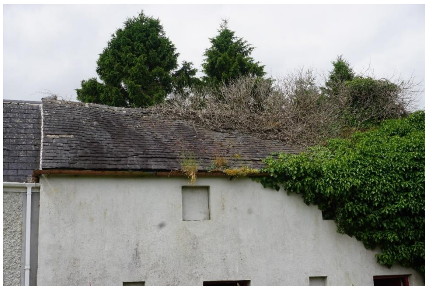
Photograph 10 - Galvanised Steel Rainwater Goods on Outbuilding Front Exterior
