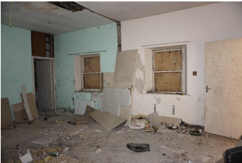
Photograph 8 - Main Living Room with Concrete Floor
