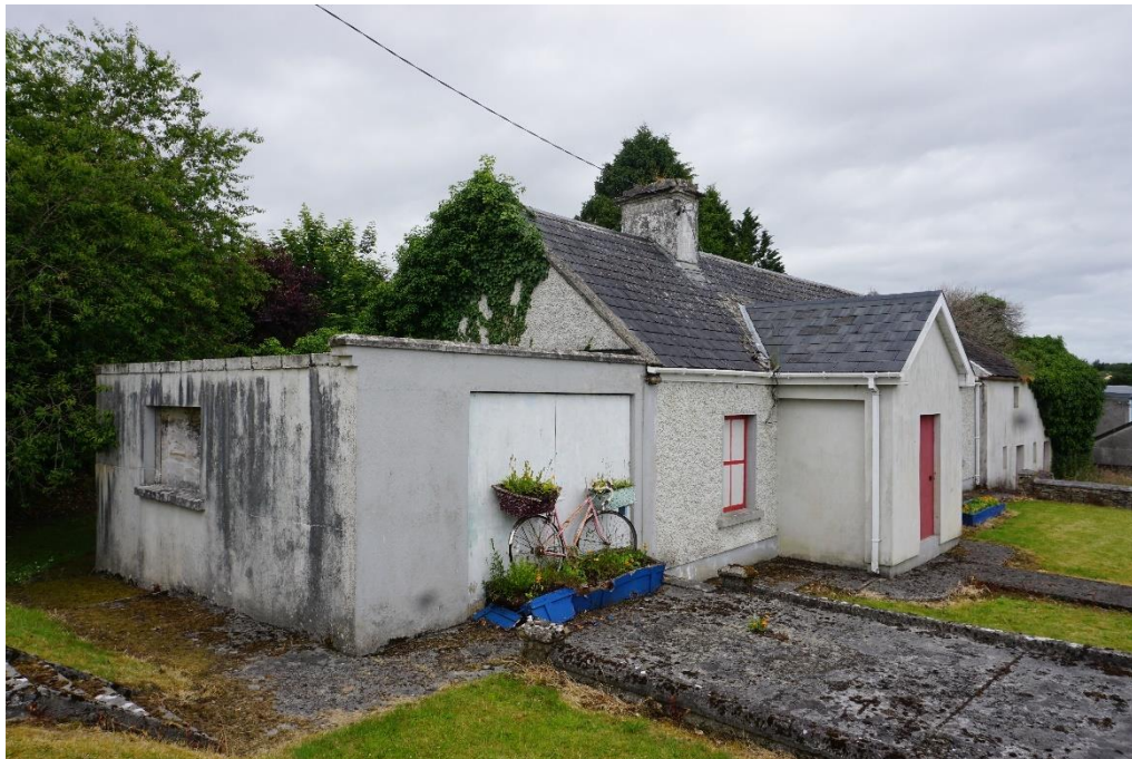
Photograph 13 – Exterior Surfaces Around Dwelling
