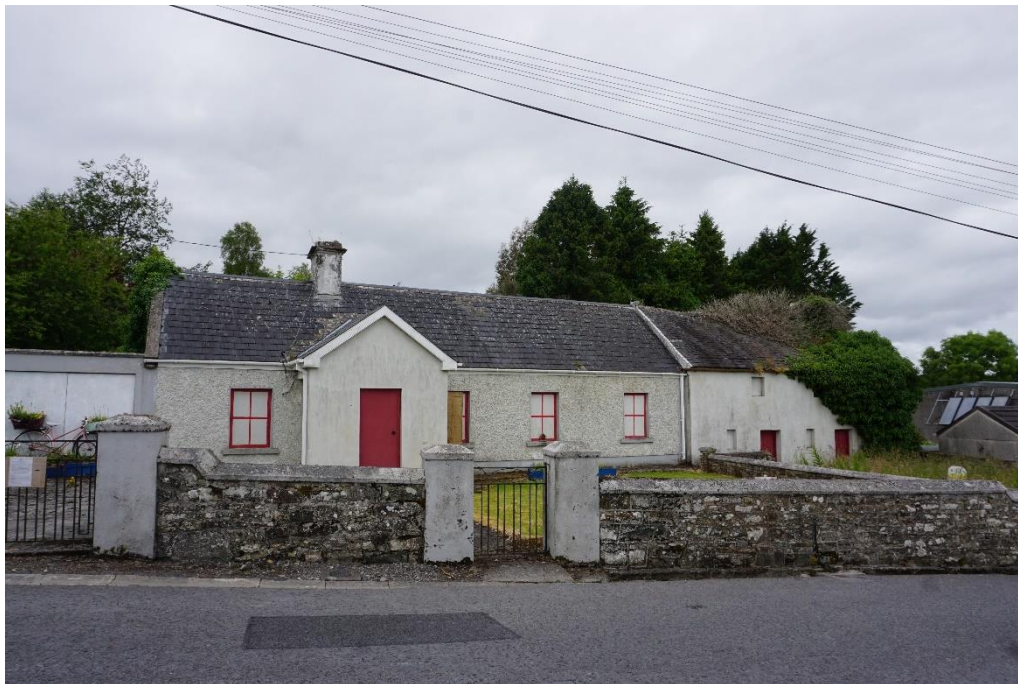
Photograph 12 – Stone Boundary Wall and Modern Gate on Eastern Side of Site
