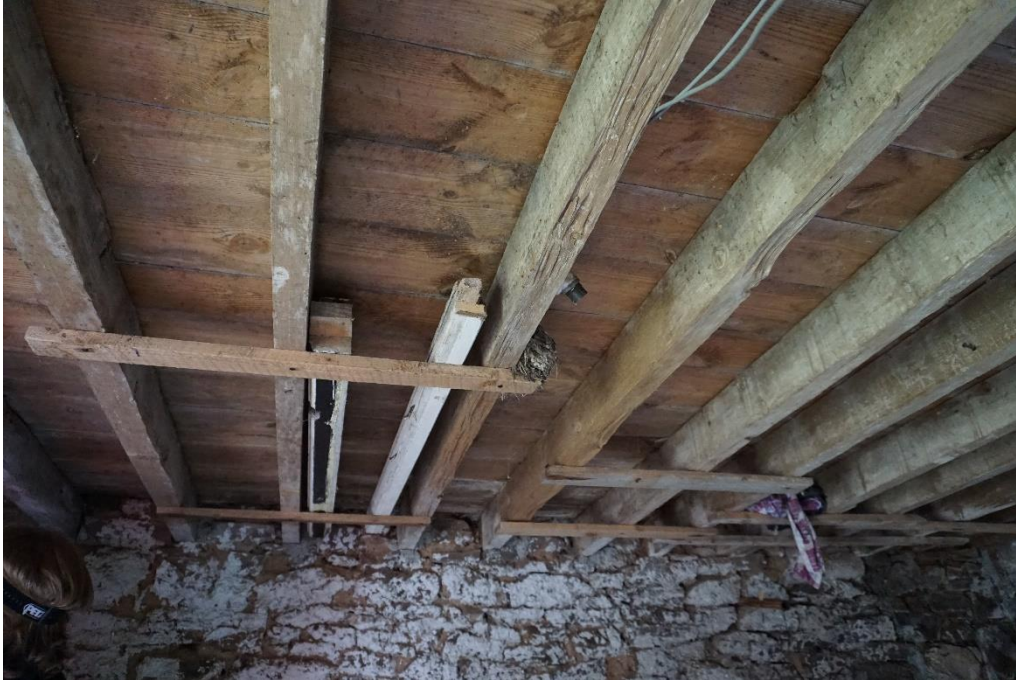
Photograph 12 - Underside of Timber Suspended Loft Floor
