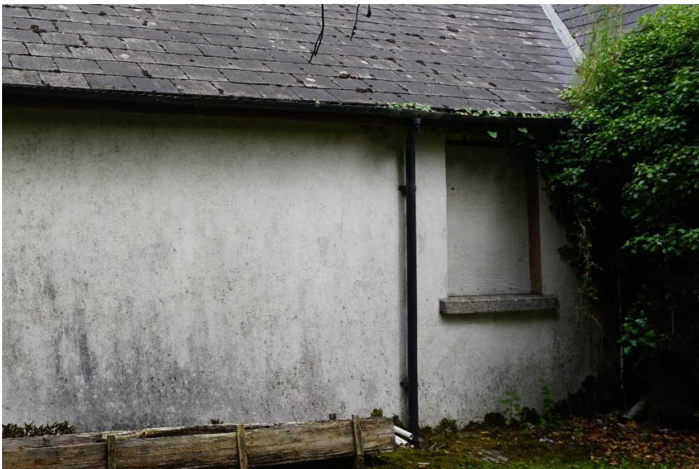
Photograph 4 - Galvanised Steel Rainwater Goods on South Elevation of Modern Extension
