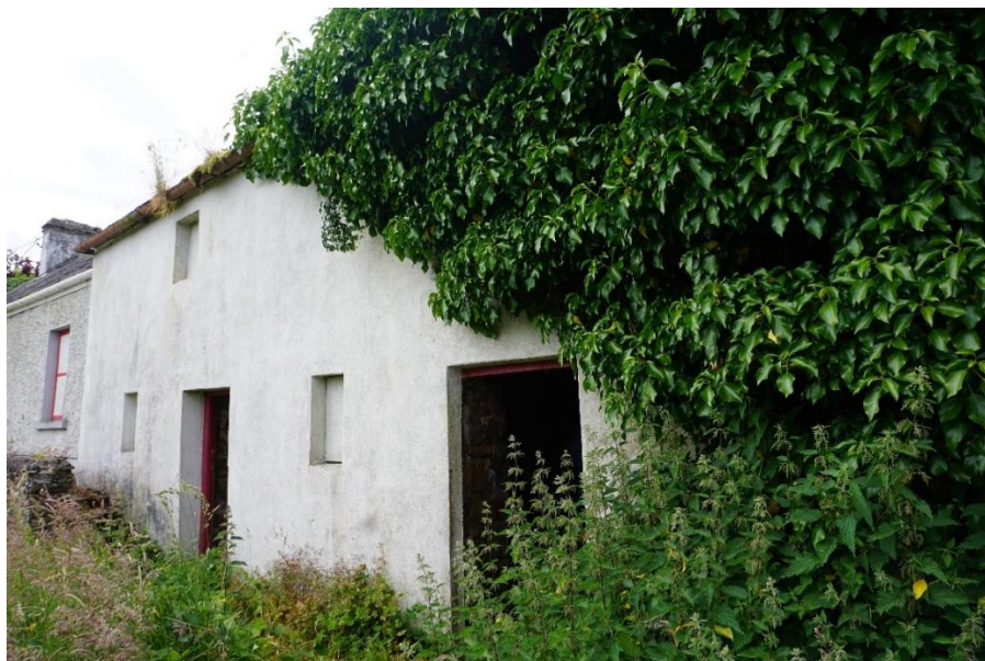
Photograph 10 – Exterior Outbuilding Traditional Timber Plank Doors
