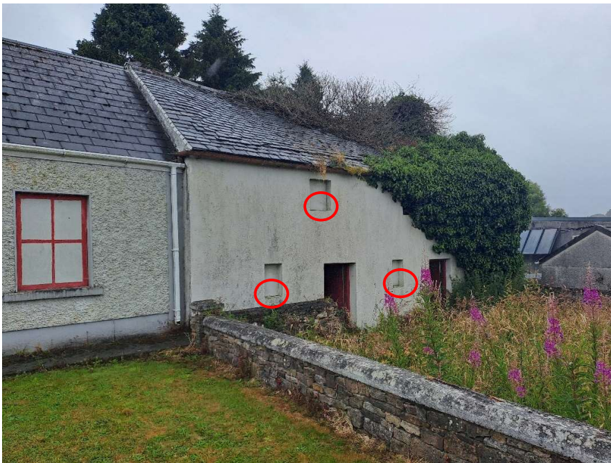
Figure 12- No existing external cills to window opes
