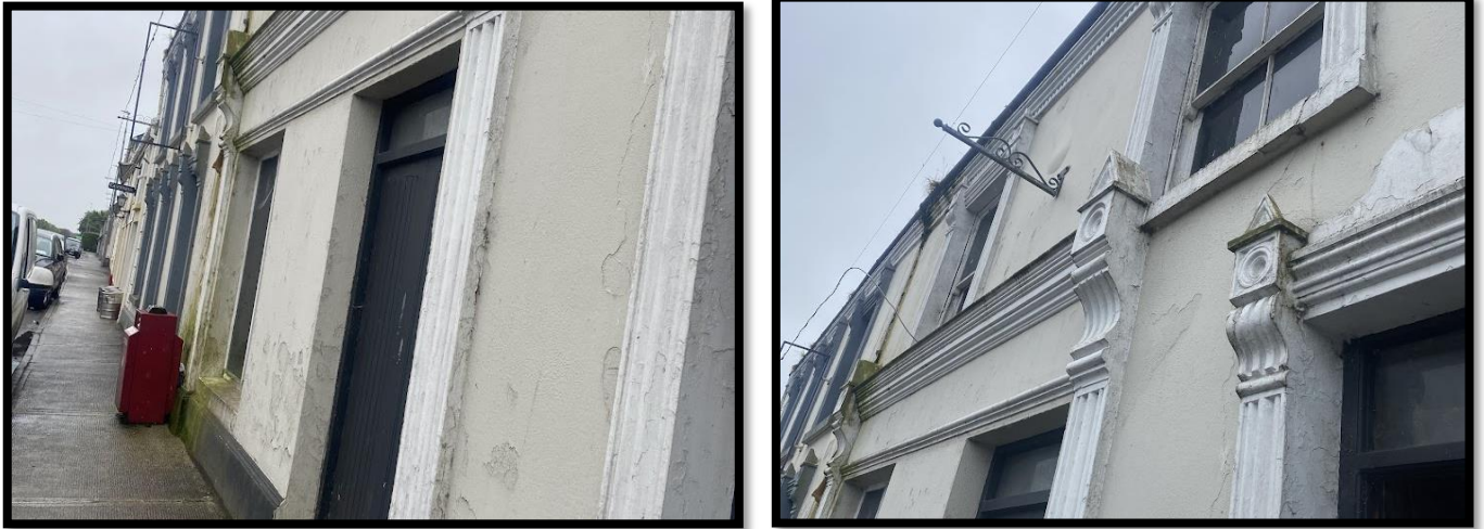
Figure 6.3- Exterior of Building 2
