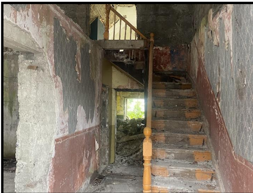
Figure 6.5- Interior of Building 2
