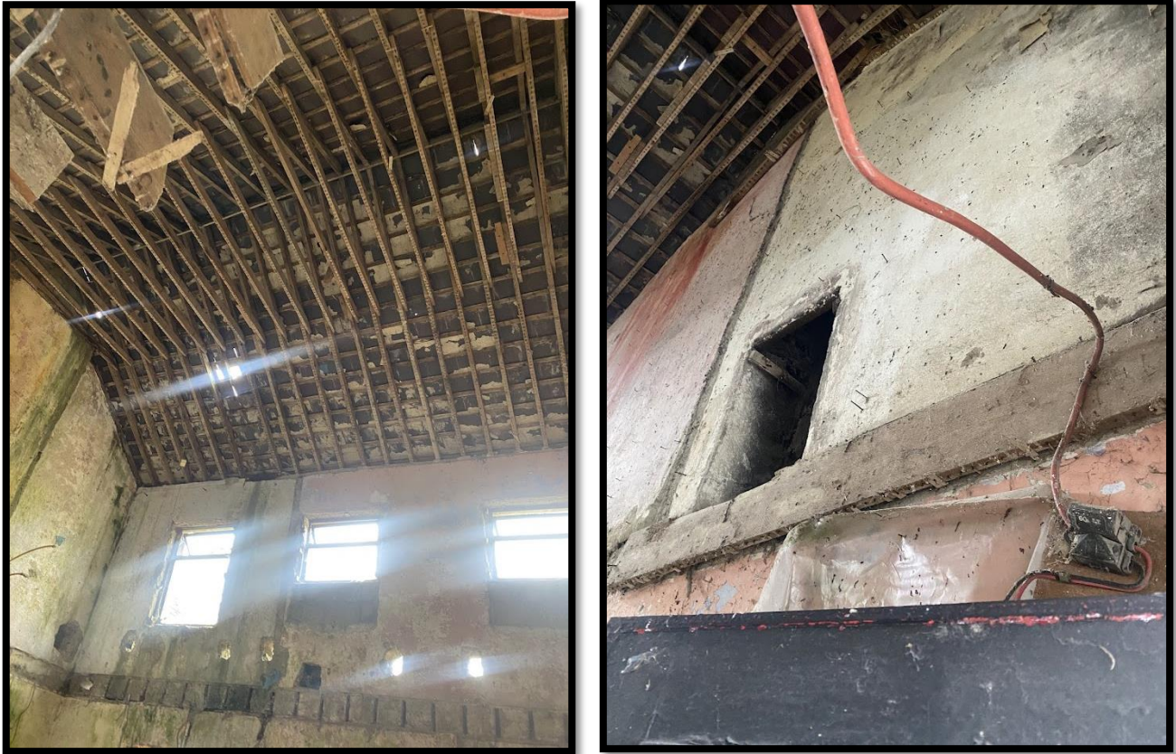
Figure 6.10- Interior of Building 3
