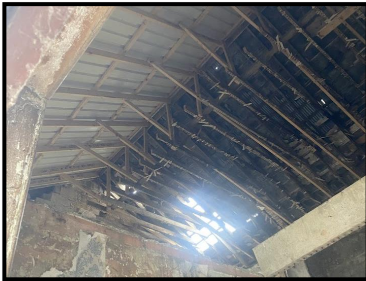
Figure 6.4- Roof of Building 2
