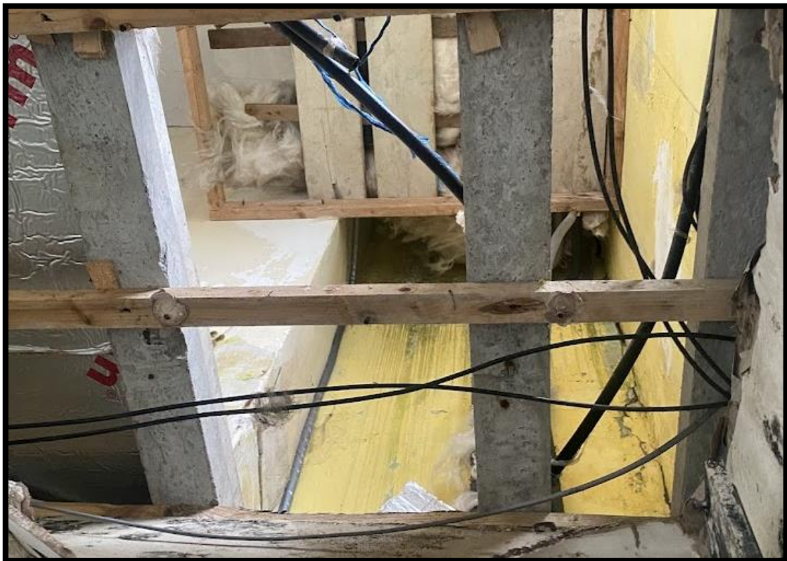
Figure 6.2- Interior of Building 1
