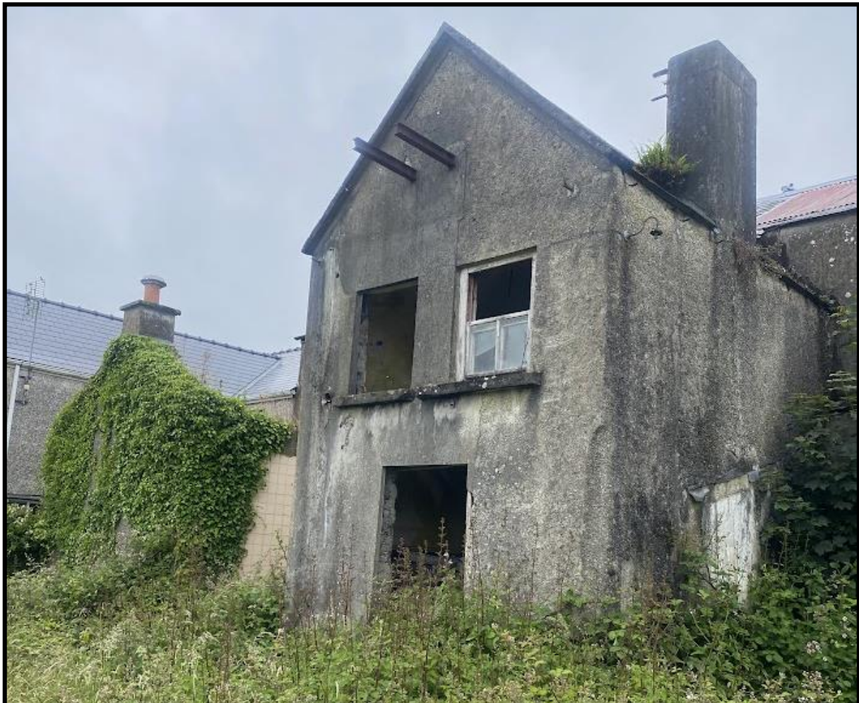
Figure 6.15- Rear of Buildings
