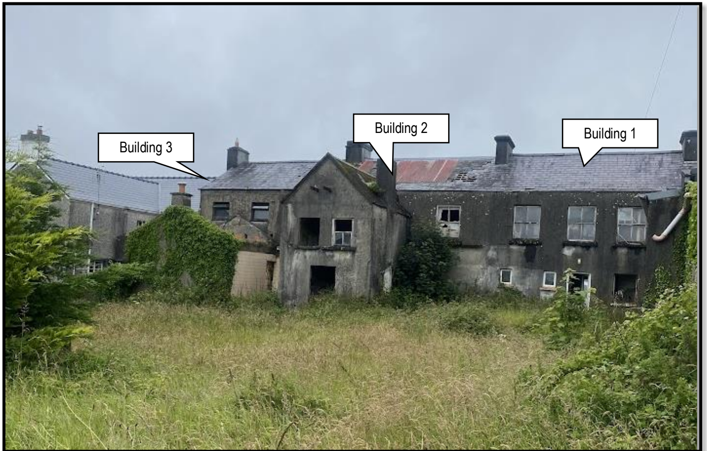
Figure 6.13- Rear of Buildings
