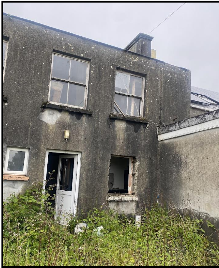
Figure 6.16- Rear of Buildings
