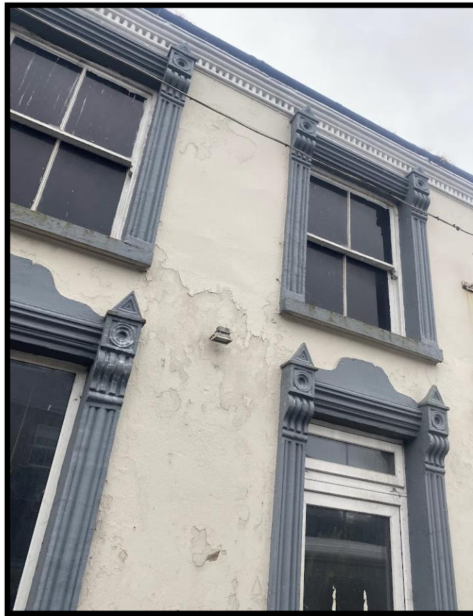
Figure 6.1- Front of Building 1
