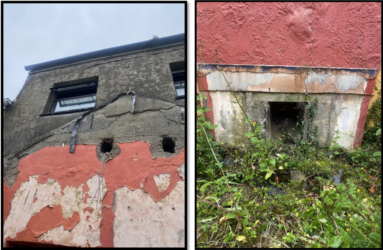
Figure 6.12- Rear of Building 3
