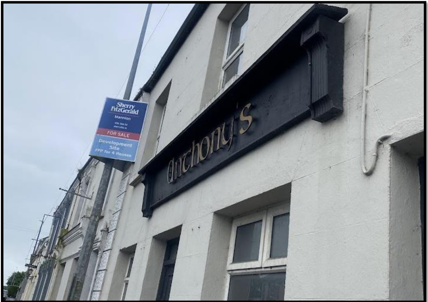
Figure 6.9- Exterior of Building 3
