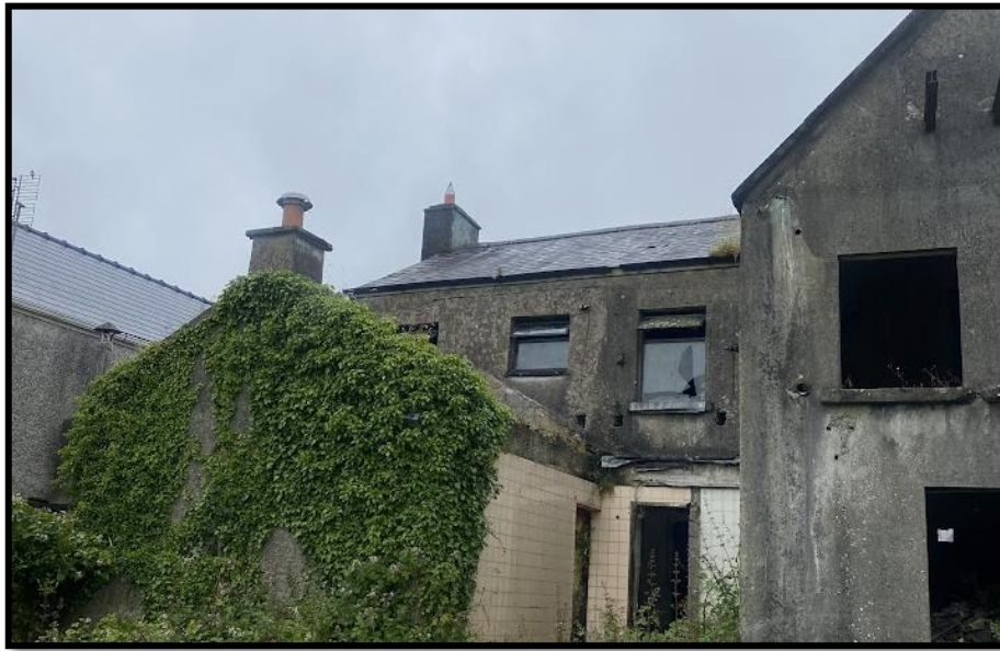
Figure 6.14- Rear of Buildings
