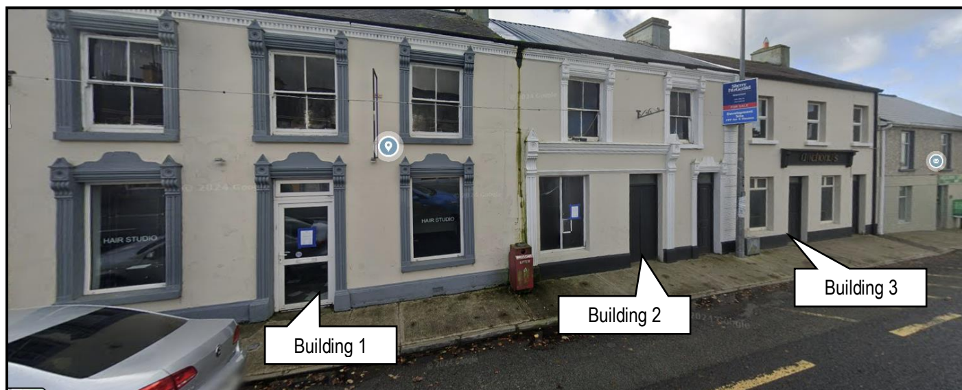
Figure 6.0- 3 no. Buildings on site
