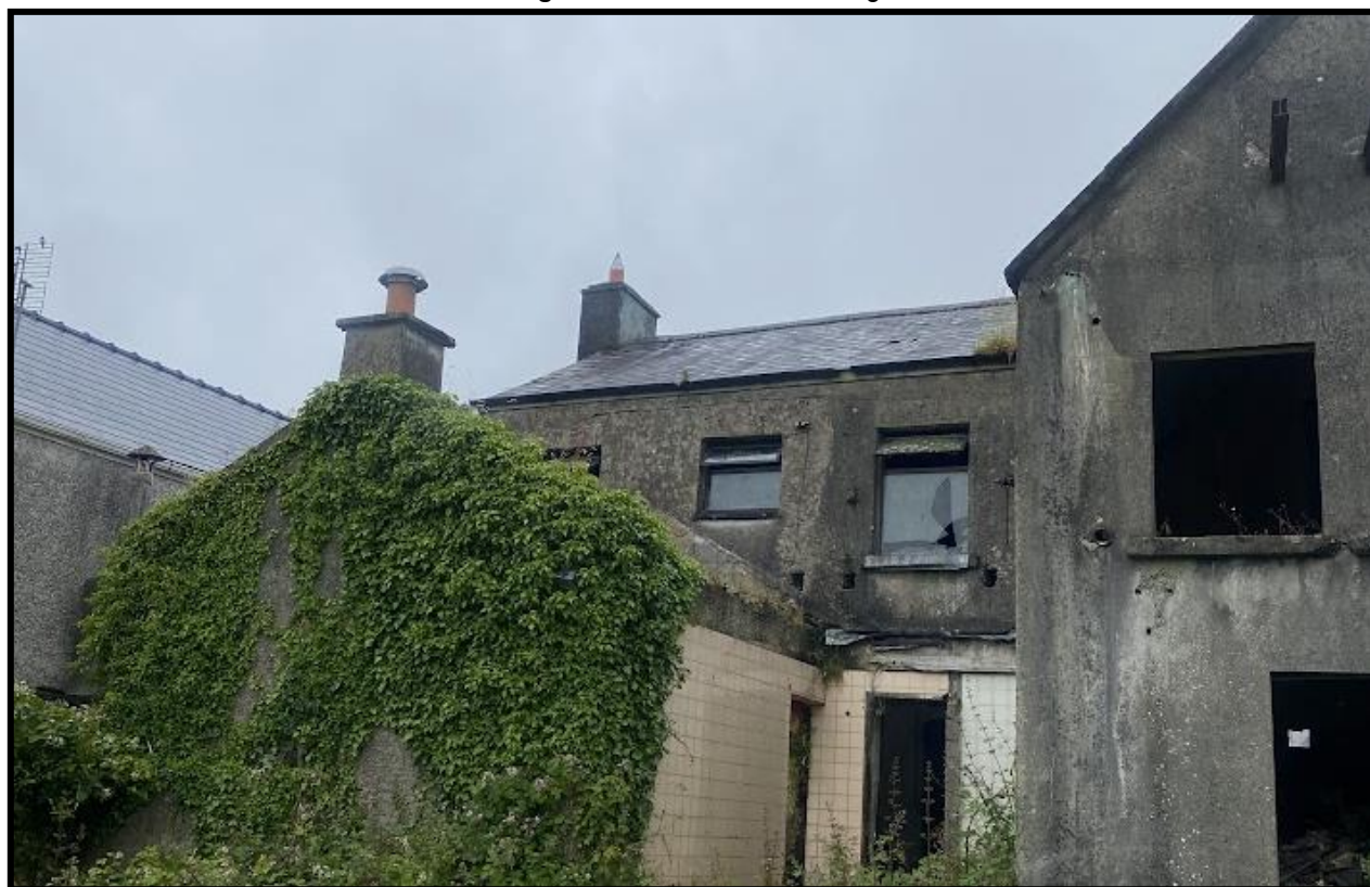
Figure 2.16- Rear of Buildings
