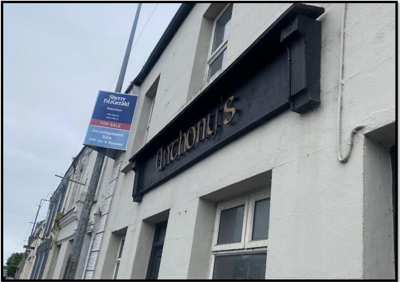
Figure 2.11- Exterior of Building 3
