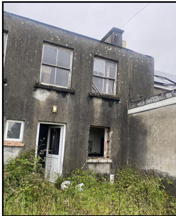
Figure 2.18- Rear of Buildings
