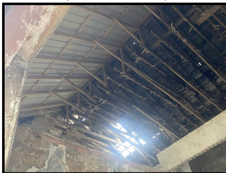
Figure 2.6- Roof of Building 2
