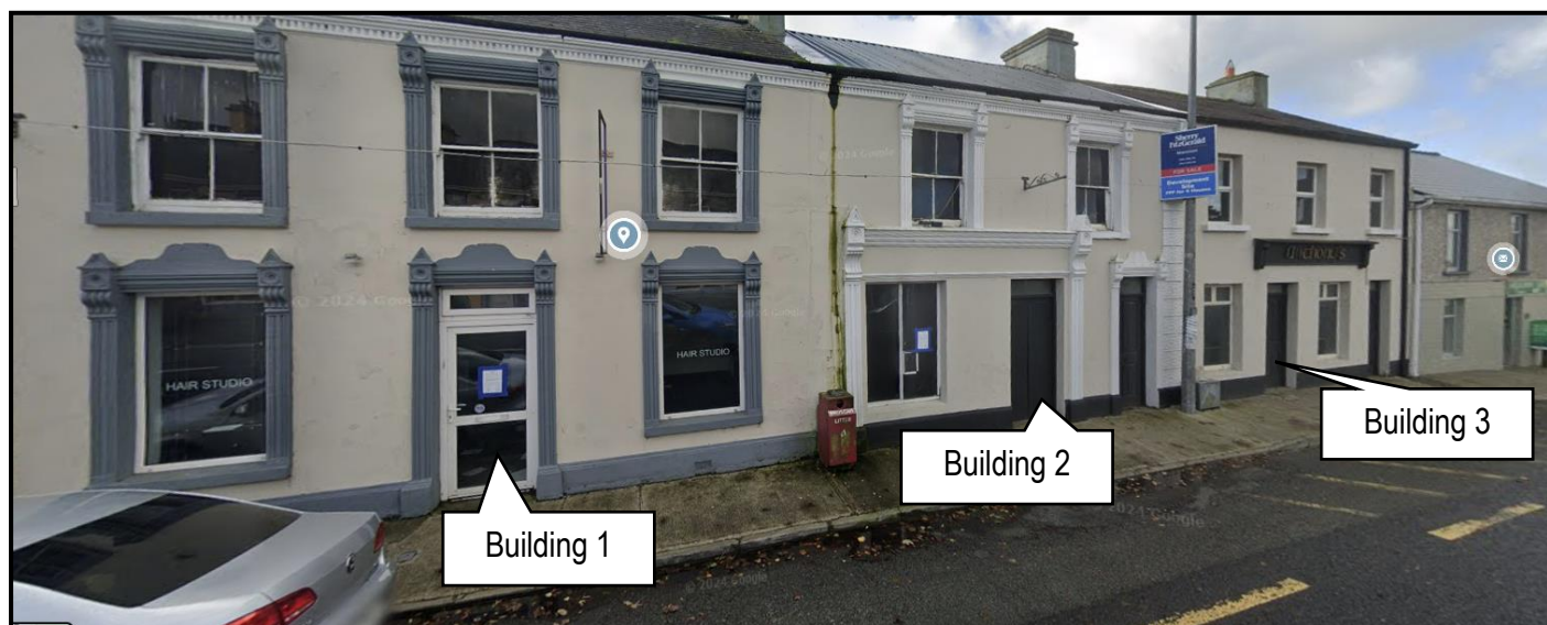
Figure 2.2- 3 no. Buildings on site
