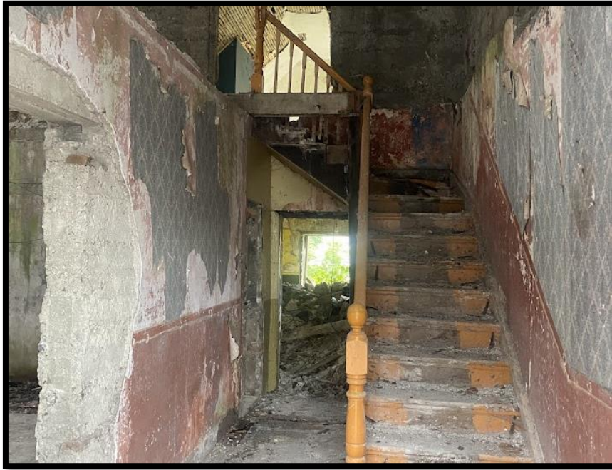
Figure 2.7- Interior of Building 2
