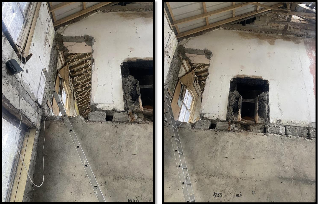
Figure 2.9- Looking to at Chimney (Building 2) and First floor of Building 1
