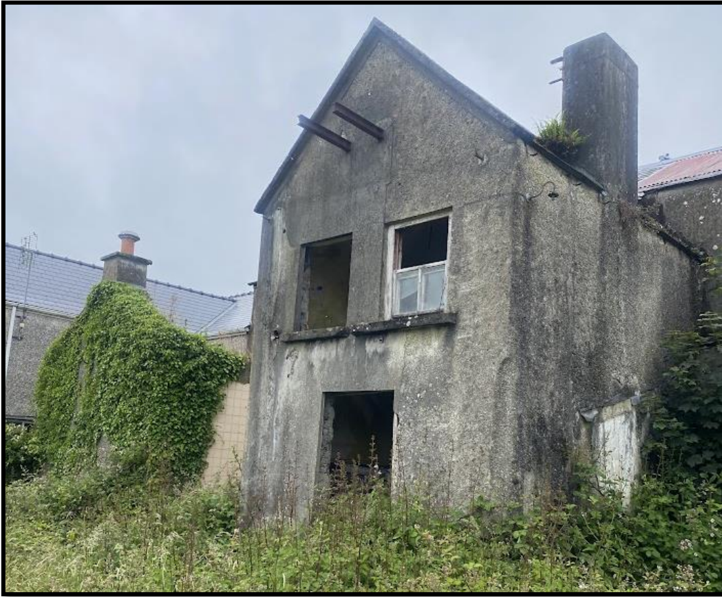
Figure 2.17- Rear of Buildings
