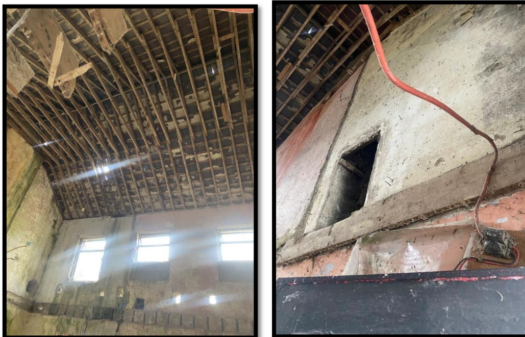
Figure 2.12- Interior of Building 3
