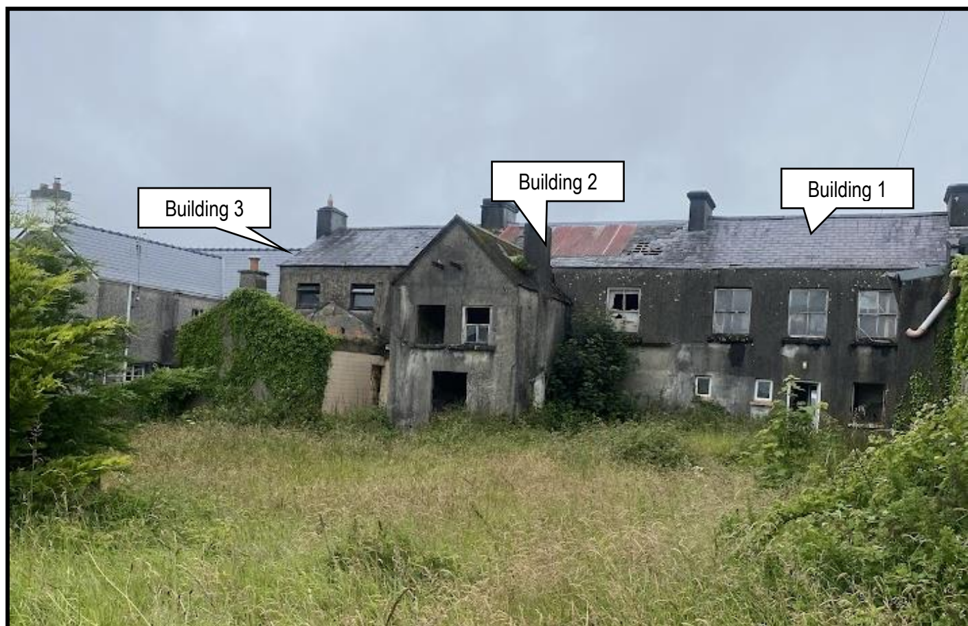
Figure 2.15- Rear of Buildings
