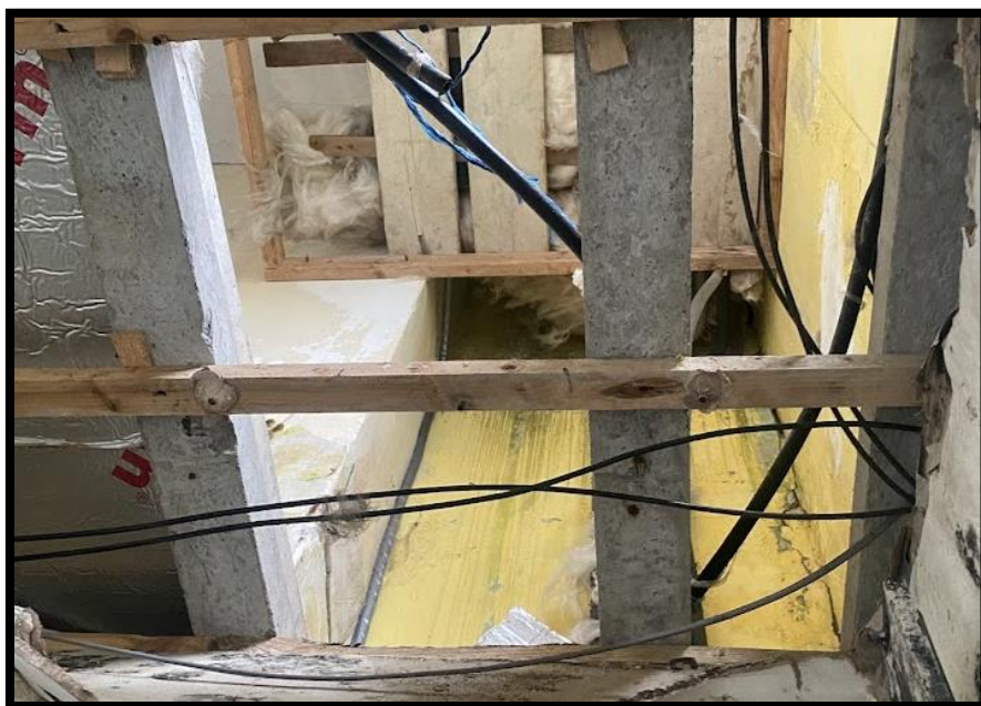
Figure 2.4- Interior of Building 1
