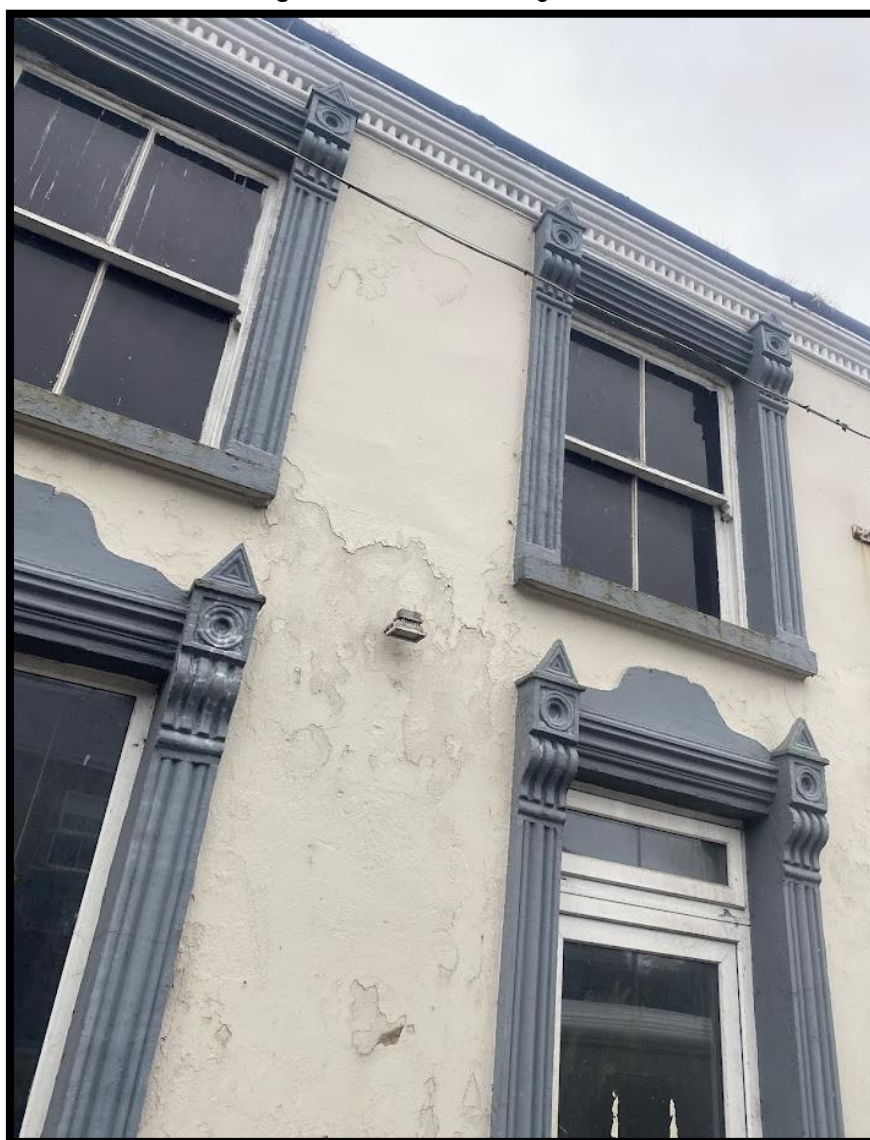
Figure 2.3- Front of Building 1
