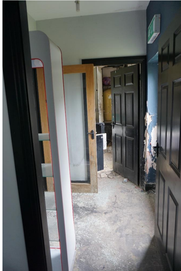
Photograph 3 Interior view of “Shelly’s”.
