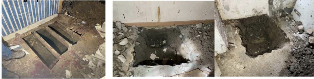
McKennas photos of existing floors- worker' cottage (timber), townhouse (solid) & Dolley's basement (solid)
