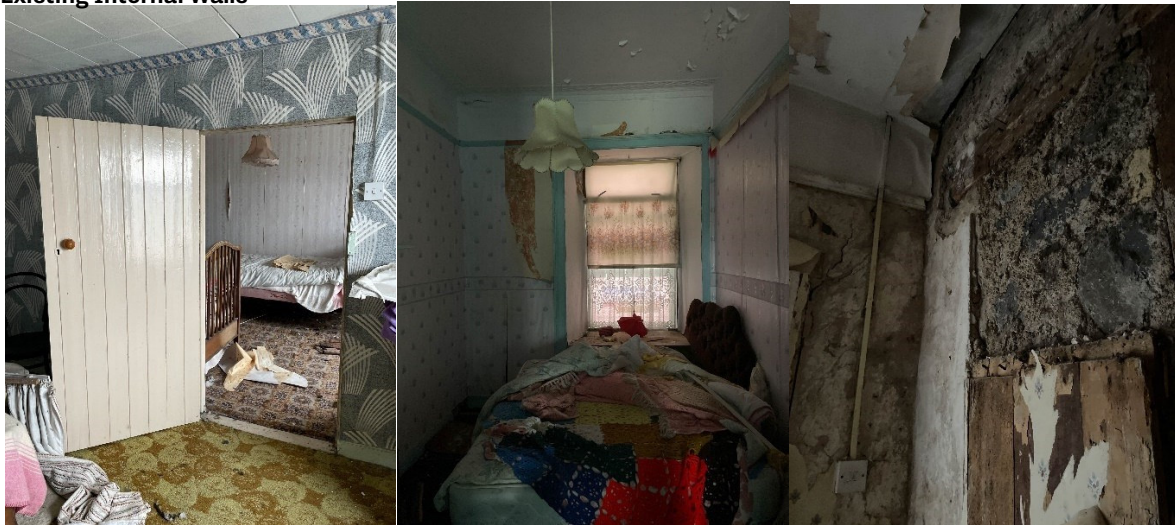
OBFA photos of existing internal walls within three-storey townhouse
