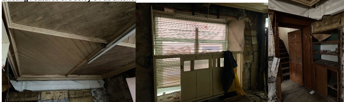
OBFA photos of existing interior elements within Dooley's Pub at ground floor level
