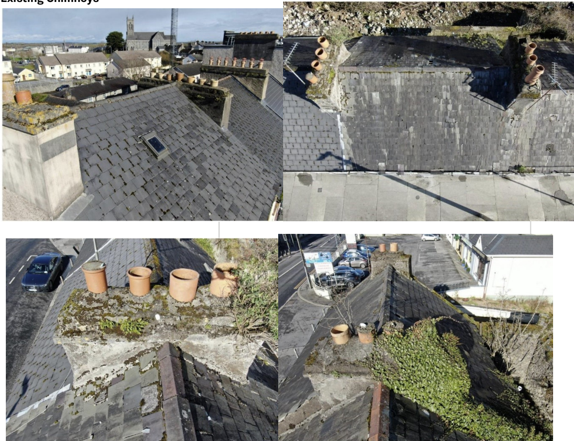
Photos of existing external Chimneys courtesy of “PJ Barrett & Co.”
