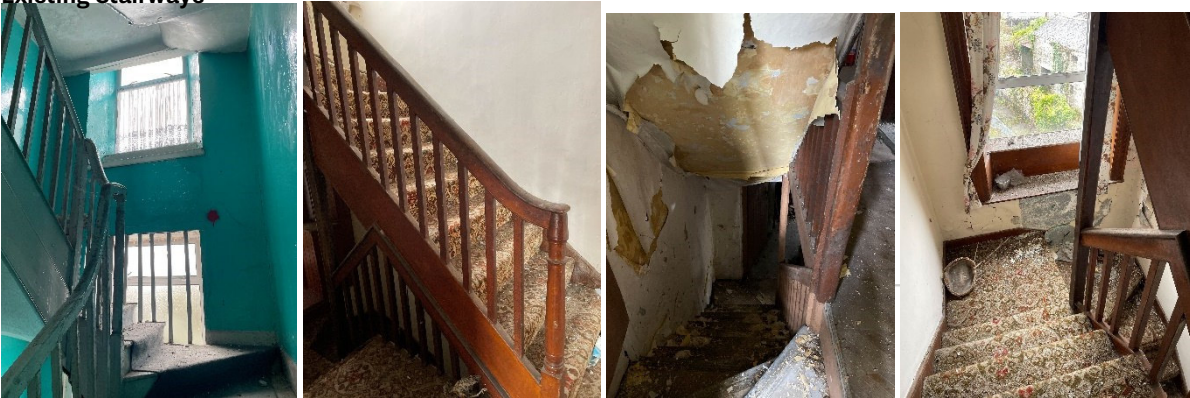
OBFA photos of existing stairways in Dooley's and adjacent townhouse
