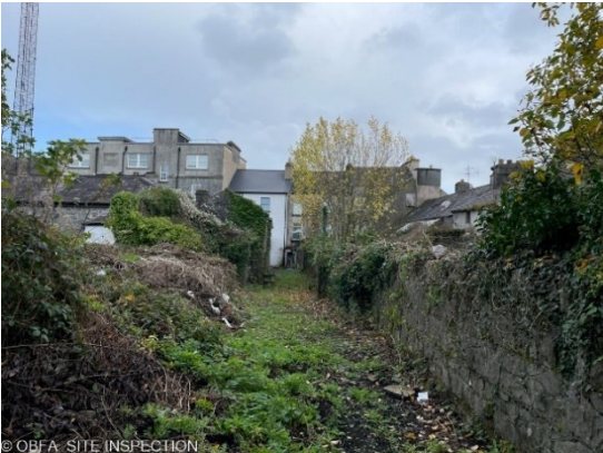
Existing stone wall sub-dividing site
