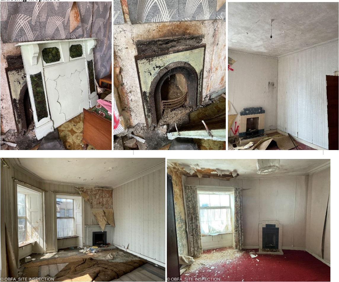
OBFA photos of existing fireplaces in Dooleys and the adjacent townhouse at Dunlo Hill.
