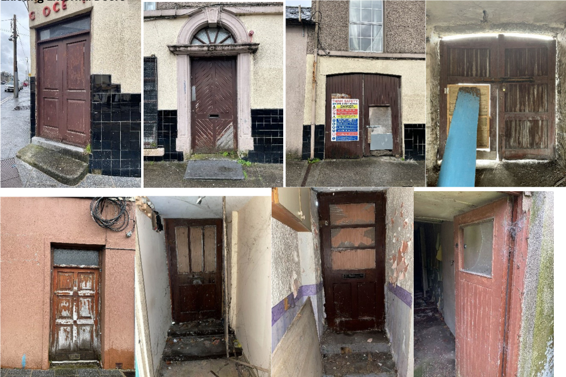
OBFA photos of existing external doorways from Dunlo Hill
