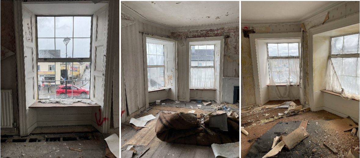
OBFA photos of existing window internal shutters, paneling & frames
