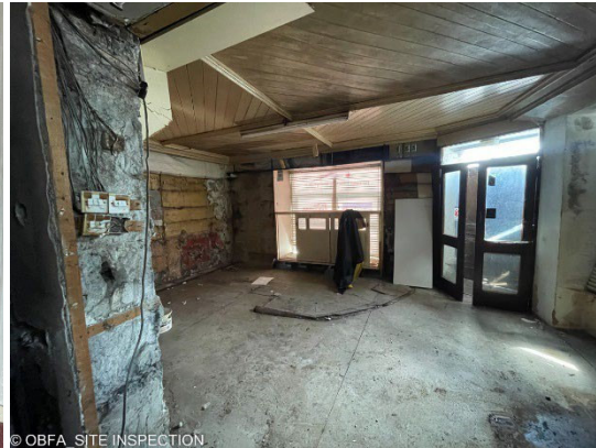
Existing timber ceiling of pub
