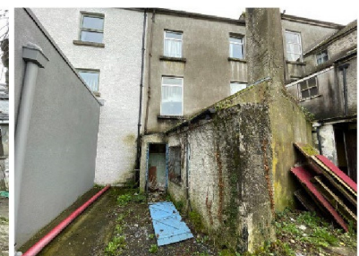
Extensions to rear of 3 storey structure
