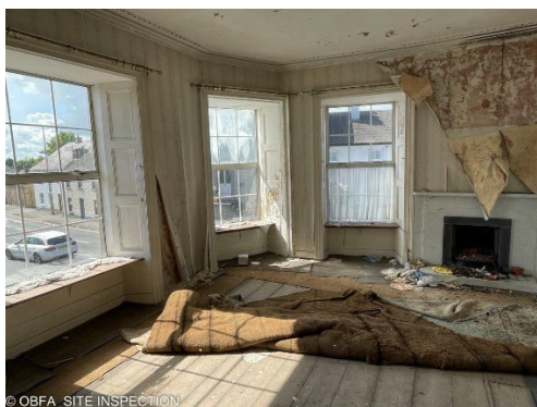
Existing shutters, skirtings, fireplace, cornices
