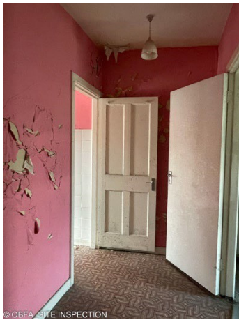
Existing timber panelled door
