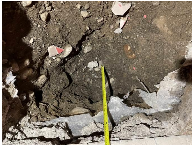
Photograph 4: Shallow depth of bearing stones under external / party walls of the existing dwellings (Unit 01). Typically, formation level is at 700mm below existing FFL
