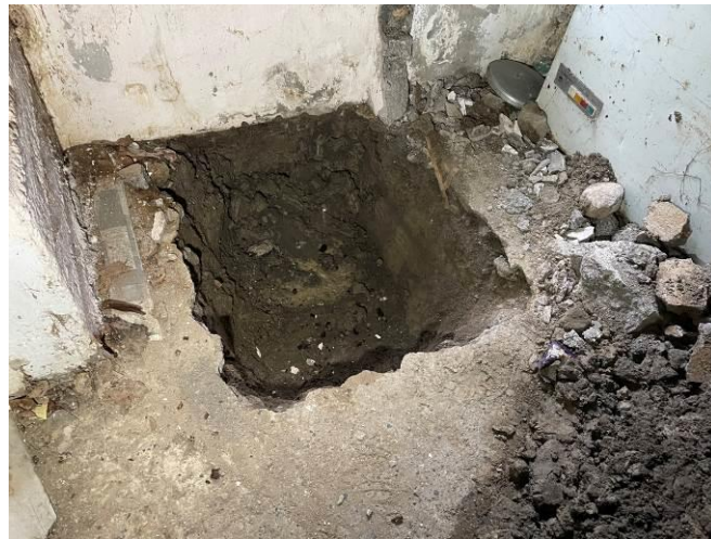
Photograph 7: Shallow depth of bearing stones under external walls of the Basement Area. Formation at 600mm below FFL
