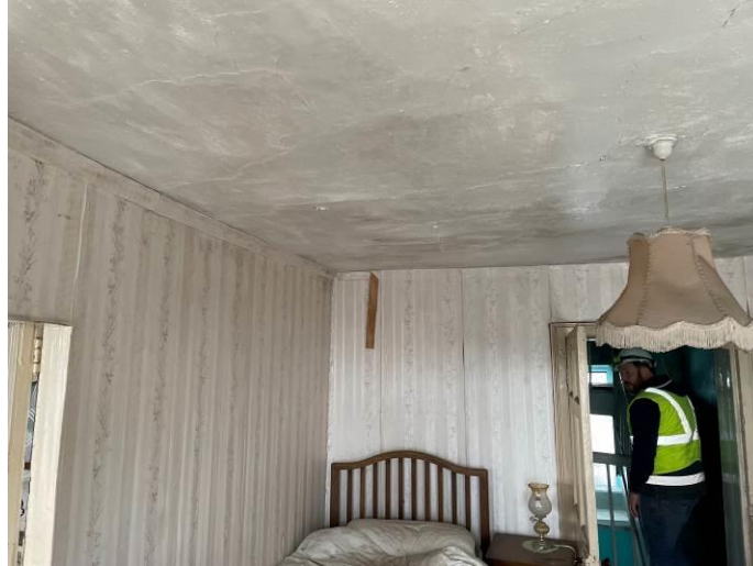
Photograph 26: Cracked and dilapidated nature of the ceilings within the public house area
