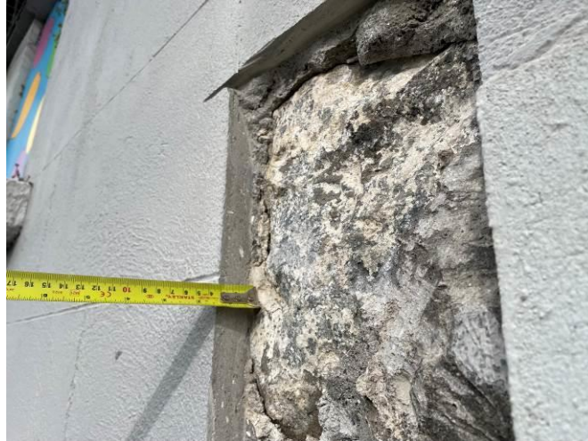
Photograph 19: Nature of the render and substrate in explorative hole at the front left side. The render is 30mm on average in thickness and well bonded to the stone
