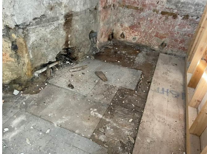
Photograph 35: Dilapidated condition of the timber floors and floor joists on the ground floor of the public house area
