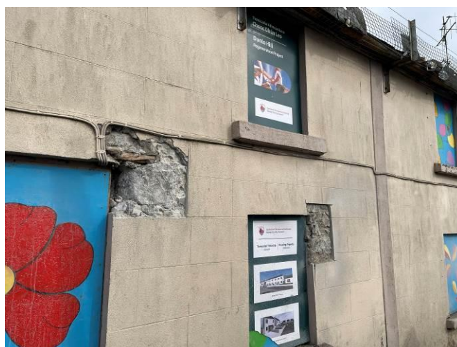
Photograph 21: Examples of the explorative holes in the render on the front elevations of the residential properties
