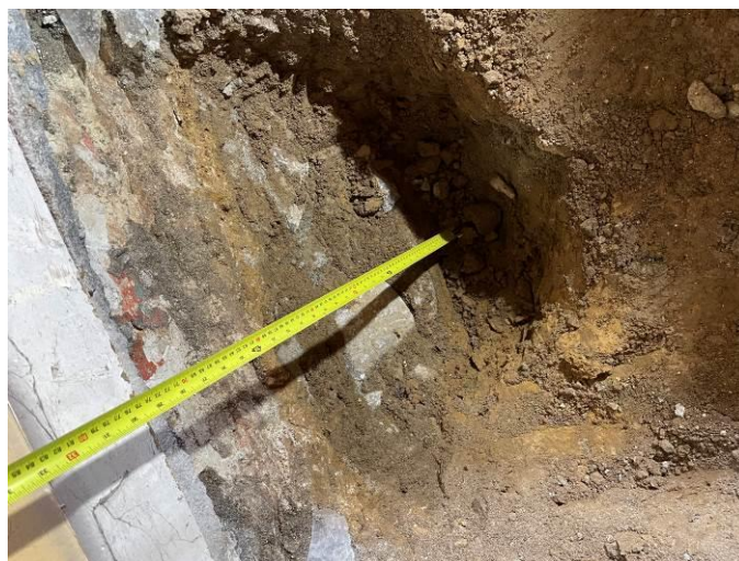
Photograph 5: Shallow depth of bearing stones under external / party walls of the existing dwellings (Unit 02)
