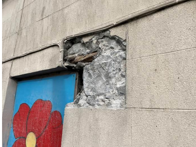
Photograph 22: Example of well bonded render and dilapidated timber lintel
