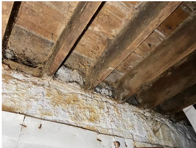
Photograph 39: Dilapidated condition of the timber floors and floor joists on the ground floor of the public house area
