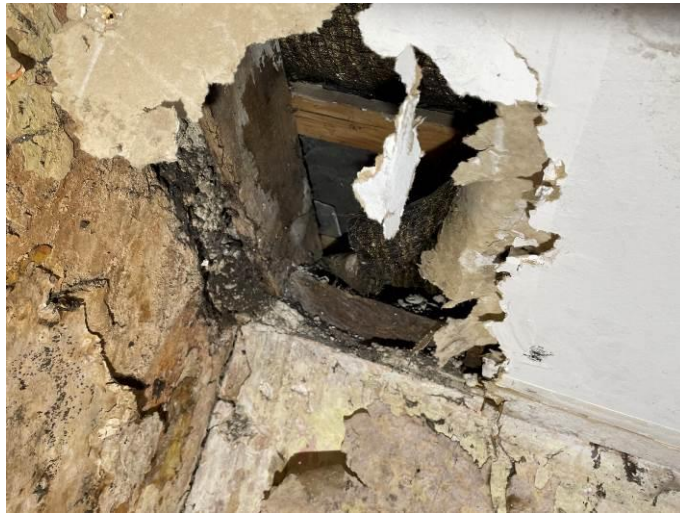
Photograph 46: Dilapidated and water damaged timber rafters in the residential property adjacent to the public house, left side
