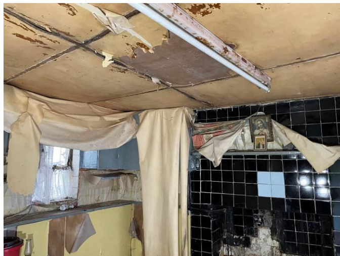
Photograph 28: Dilapidated nature of the walls and ceilings within the public house area
