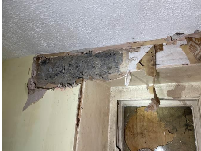
Photograph 10: Concrete & stone lintels were also noted in places within the residential properties
