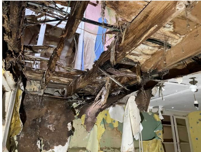
Photograph 32: First floor joists were found to be in this dilapidated condition within a number of the residential units
