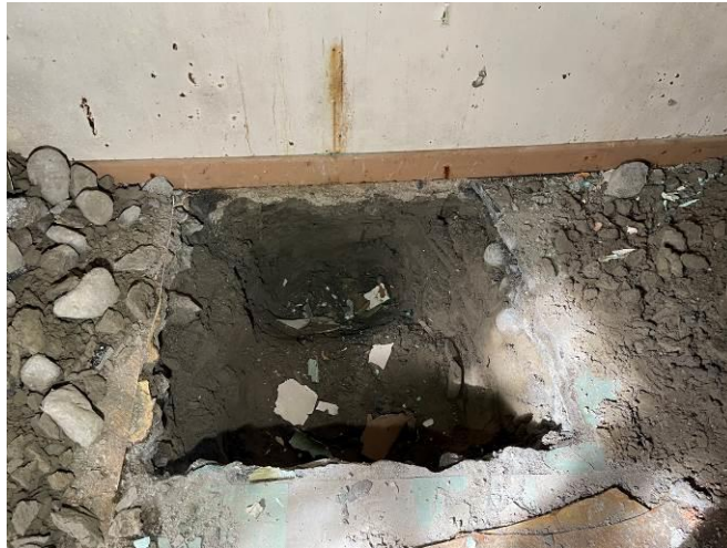
Photograph 6: Shallow depth of bearing stones under external / party walls of residential property adjacent to the Public House. Formation at 600mm below FFL
