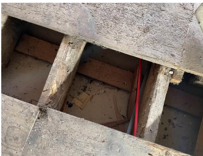
Photograph 34: Woodworm attack noted in the floor joists at the location above
