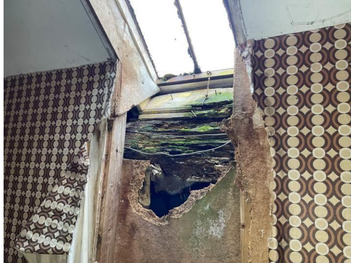
Photograph 45: Dilapidated and water damaged timber purlins in the residential property adjacent to the public house, left side
