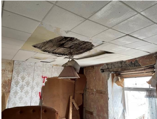
Photograph 27: Dilapidated nature of the walls and ceilings within the public house area
