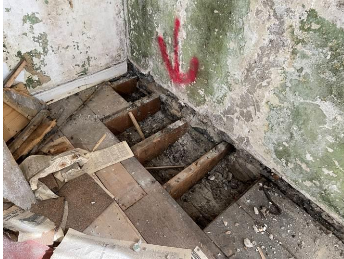
Photograph 38: Good condition of the timber second floor joists in the public house area
