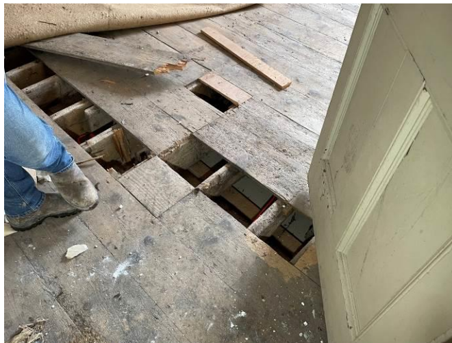
Photograph 33: Brittle condition of the floorboards and floor joists in the property adjacent to the archway
