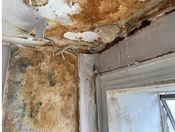
Photograph 29: Dilapidated nature of the walls and ceilings within the public house area
