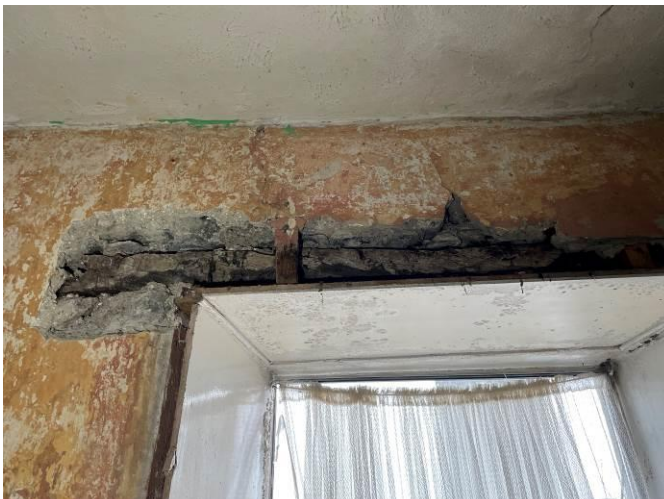
Photograph 15: Typical example of the dilapidated nature of the timber lintels
