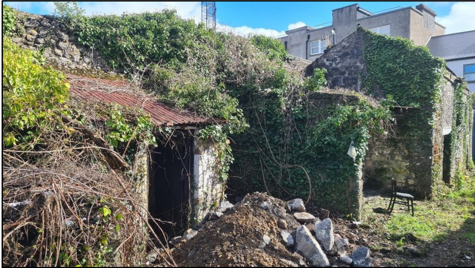
Plate 7 Facing E showing outbuildings abutting N boundary wall
