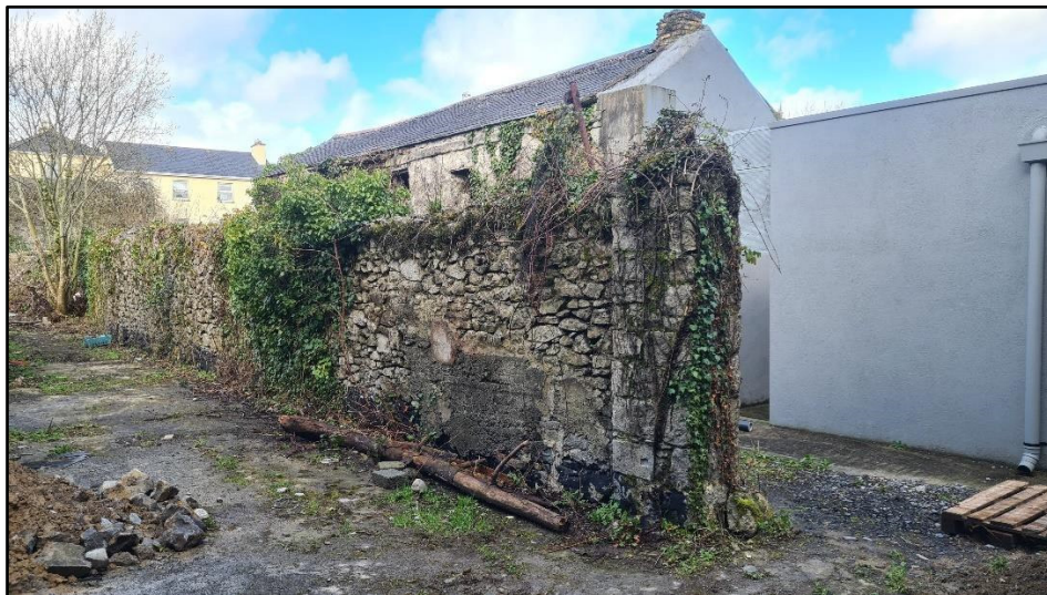
Plate 5 Facing NW showing gate pillar at east extent of internal boundary wall
