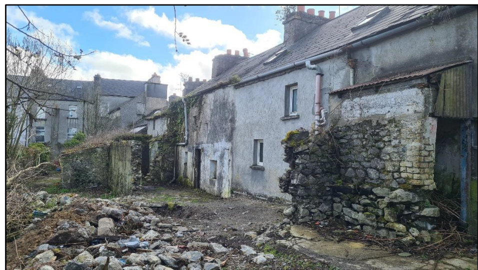
Plate 12 Facing E showing rear of terraced dwellings
