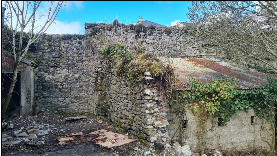
Plate 10 Facing W showing outbuilding abutting W boundary wall
