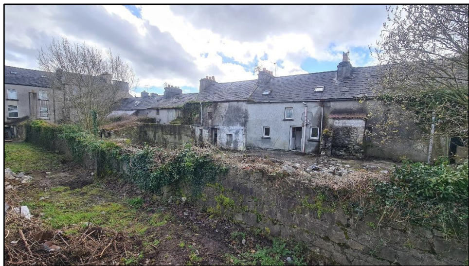
Plate 3 Facing SE showing west part of internal boundary wall (and rear of terraced houses)
