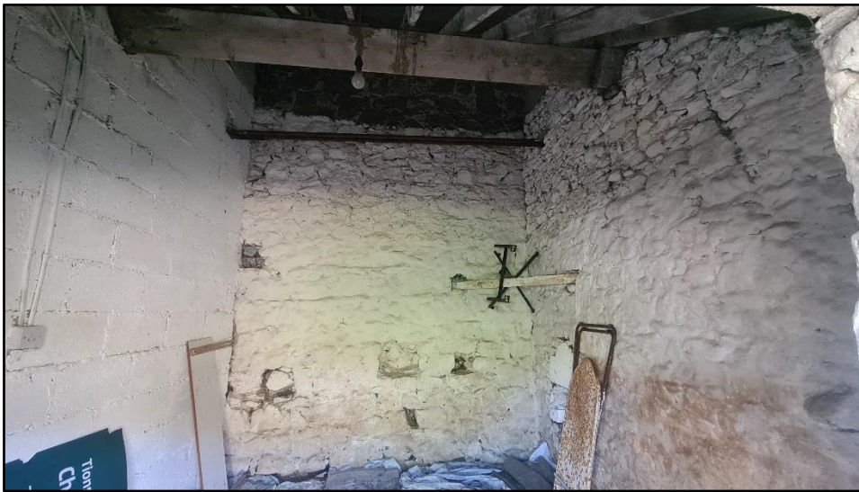
Plate 14 Interior of whitewashed extension (see plate 13) abutting rear wall of dwelling
