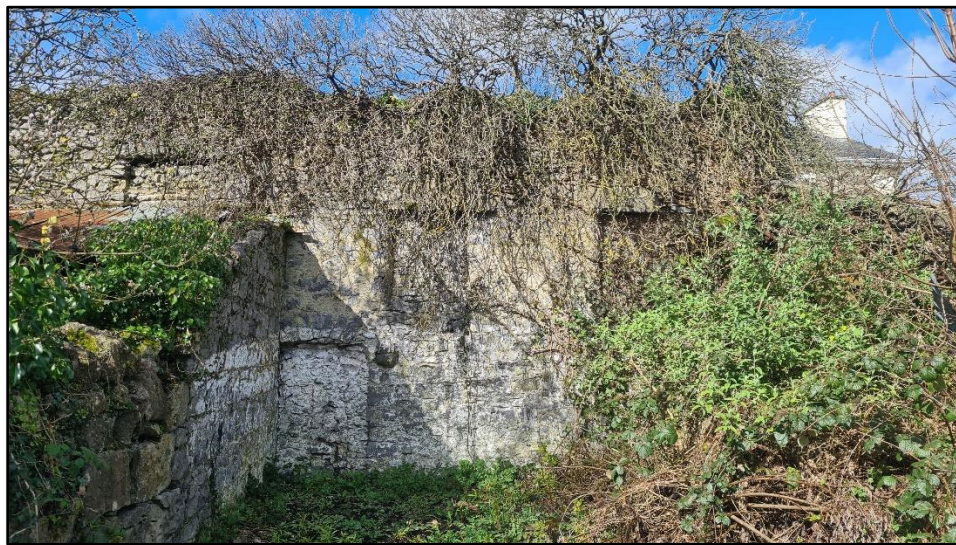
Plate 11 Facing W showing blocked opes in W boundary wall
