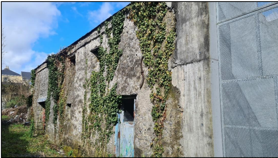
Plate 8 Facing W showing outbuildings abutting N boundary wall
