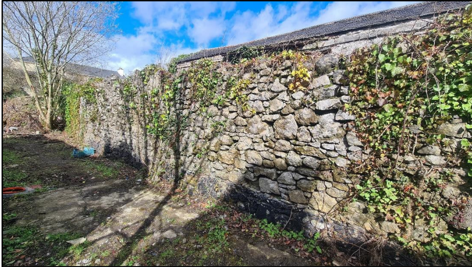
Plate 4 Facing NW showing E part of internal boundary wall
