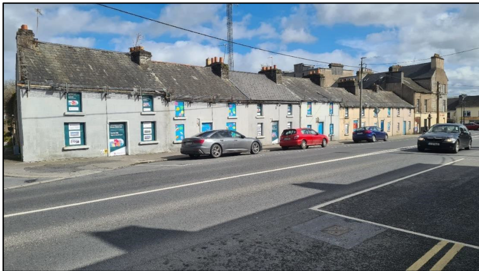
Plate 2 Facing NE showing site façade at Dunlo Hill
