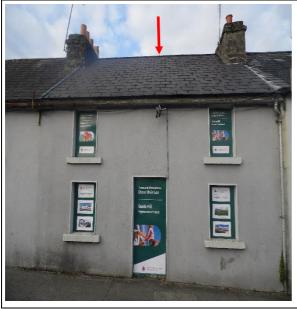
Slates to Roof of Terraced House #5 are strongly presumed ACM's
