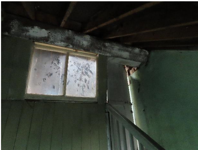
Photo 58 – stairs to attic space
