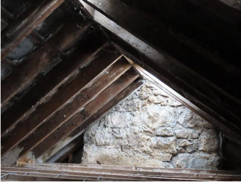
Photo 22 - Attic space of Property 1
