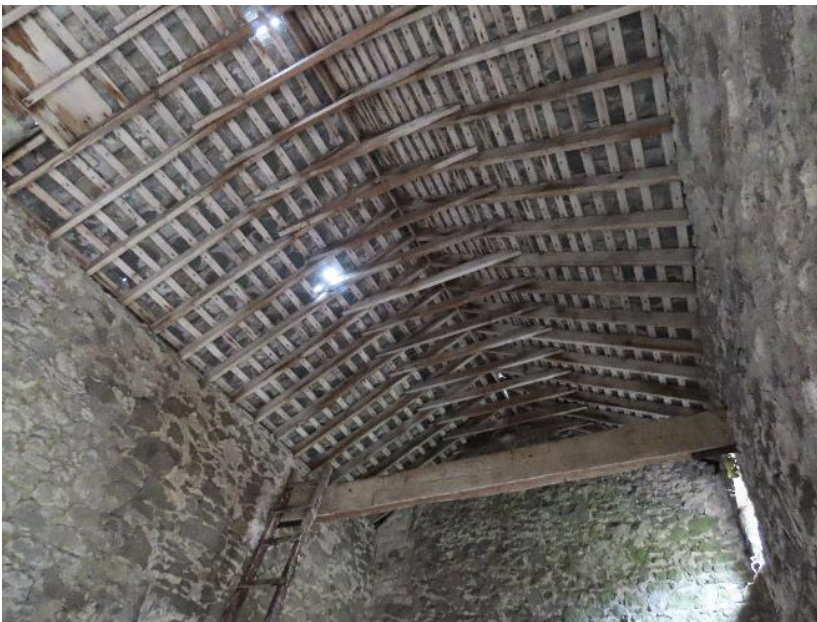
Photo 62 – exposed roof timbers in outbuilding
