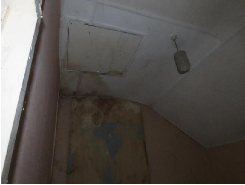
Photo 37 – trap door to attic of Property 6
