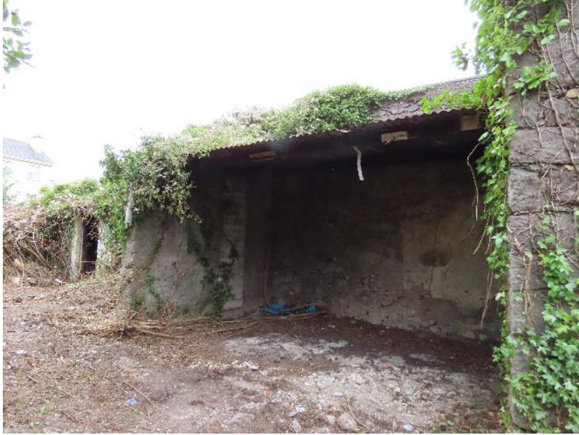
Photo 63 – lean-to building attached to stone outbuilding
