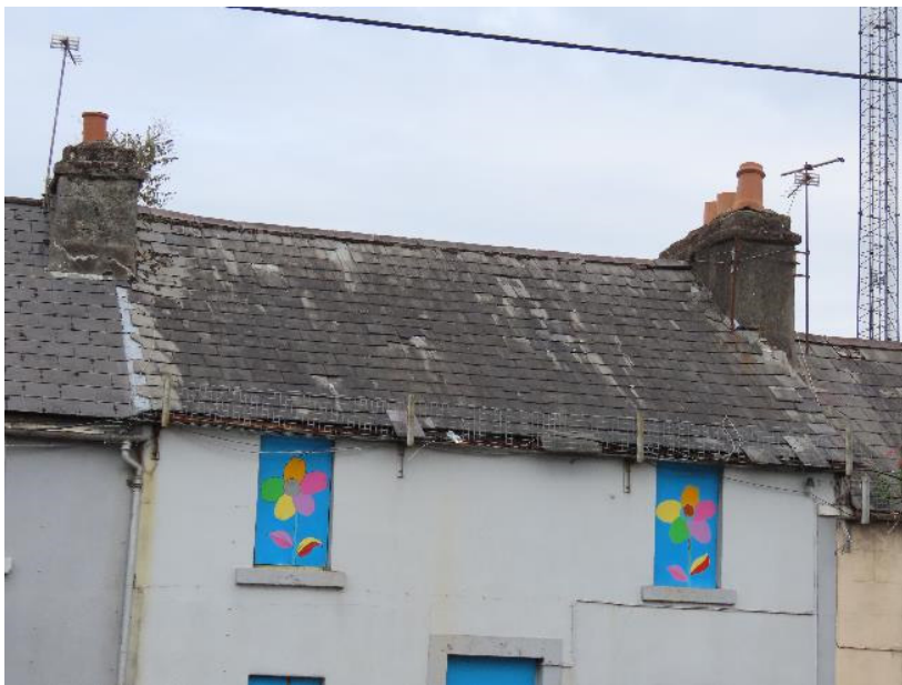
Photo 4 - Property 4 – showing poor condition of roof. Wire slate guard in place to catch falling slates
