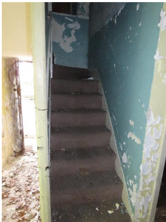
Photo 31 – stairs in Property 4
