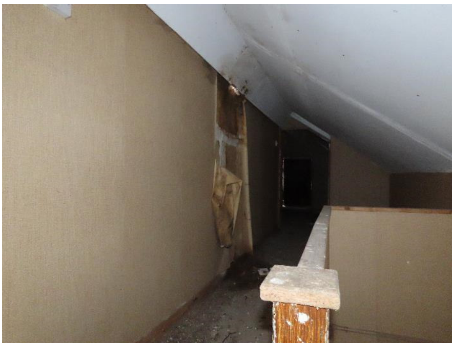
Photo 46 – upstairs landing of rear section of building
