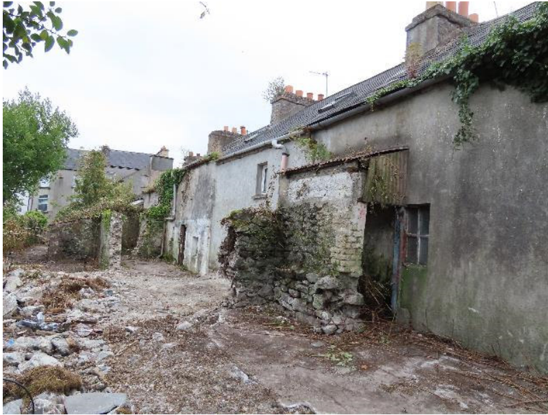
Photo 16 - Rear of Dunlo Terrace looking east
