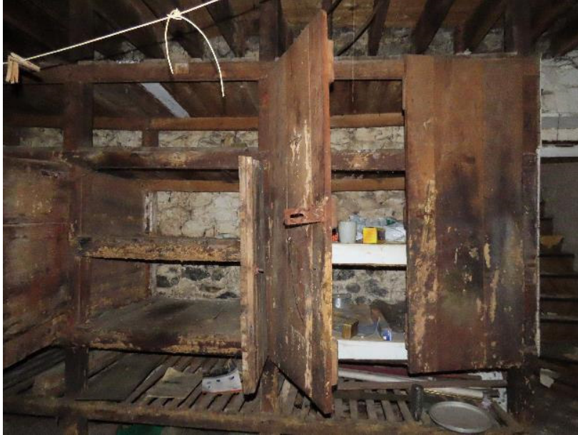
Photo 53 – basement in P.Dooley's
