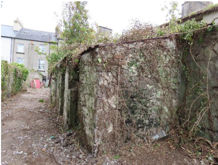
Photo 42 - Sheds to rear of Property 5, 6 & 7
