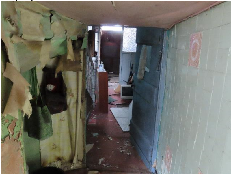
Photo 55 – hallway of Property 9
