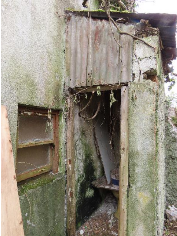
Photo 39 - Outdoor toilet outside property 6
