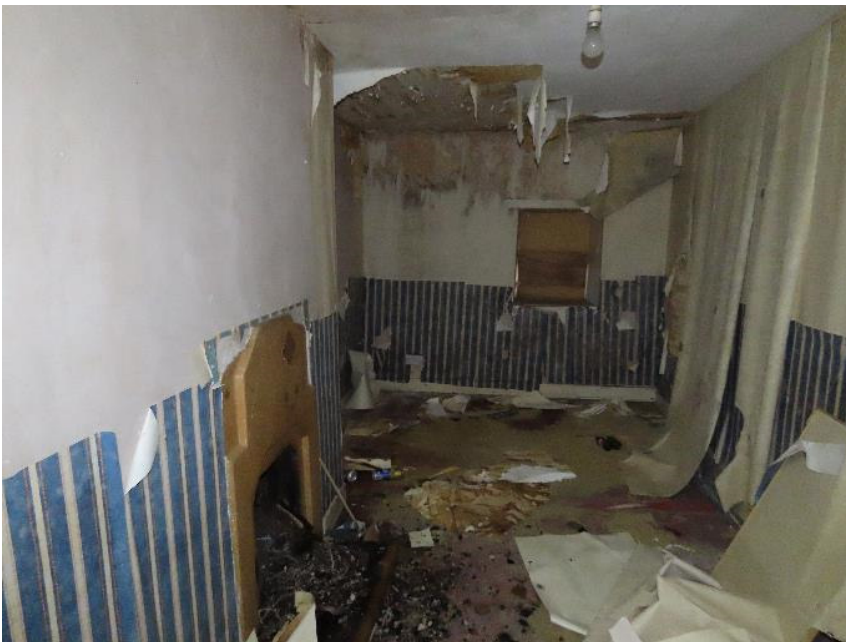
Photo 40 – sitting room of Property 7
