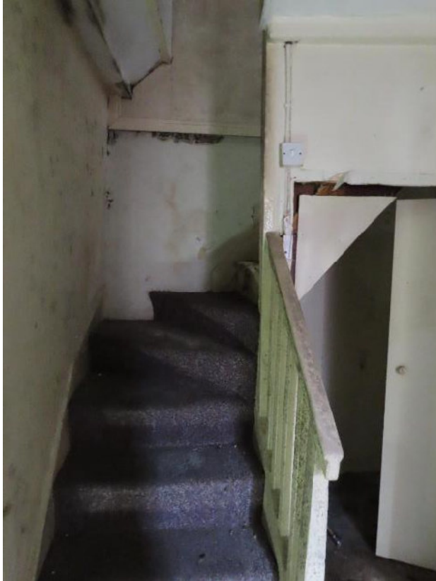
Photo 35 – stairs in Property No 6
