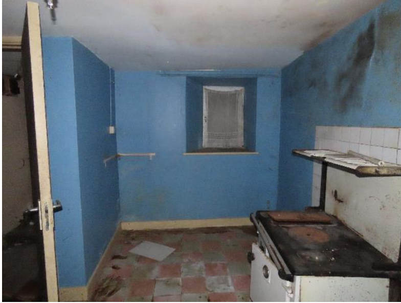
Photo 24 - Kitchen of Property 2 on Dunlo Hill terrace
