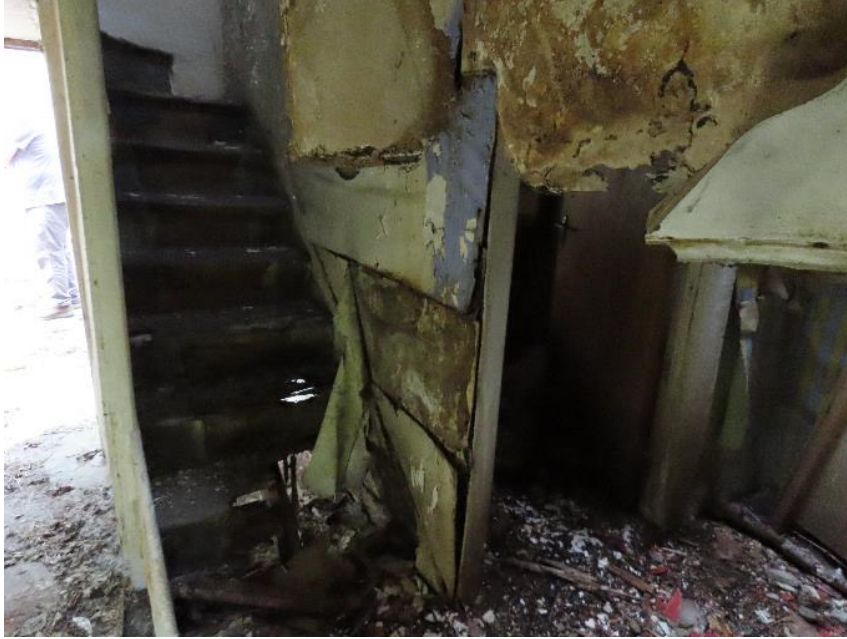
Photo 41 - Stairs in Property 7
