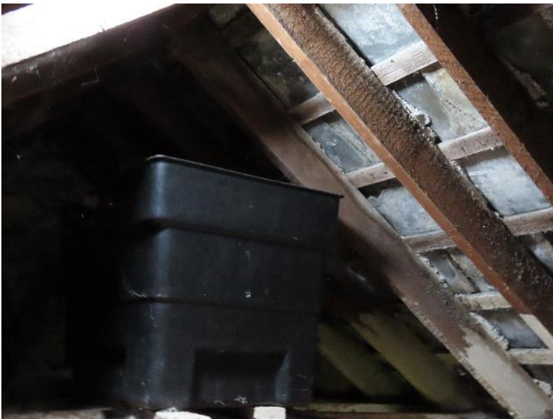
Photo 23 - Attic space of Property 1 showing original slates
