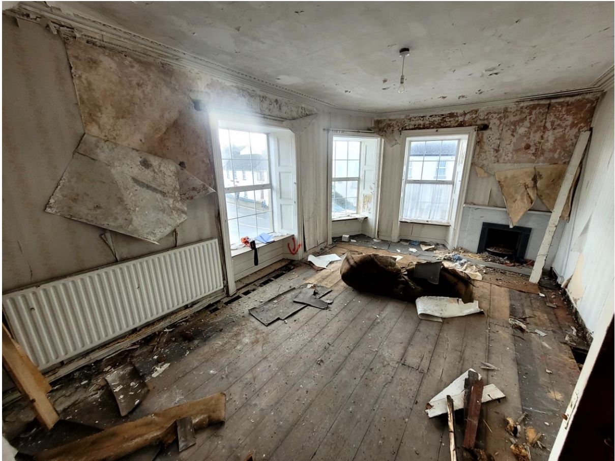
Figure 13. Shows a broad view of the first-floor front room.
