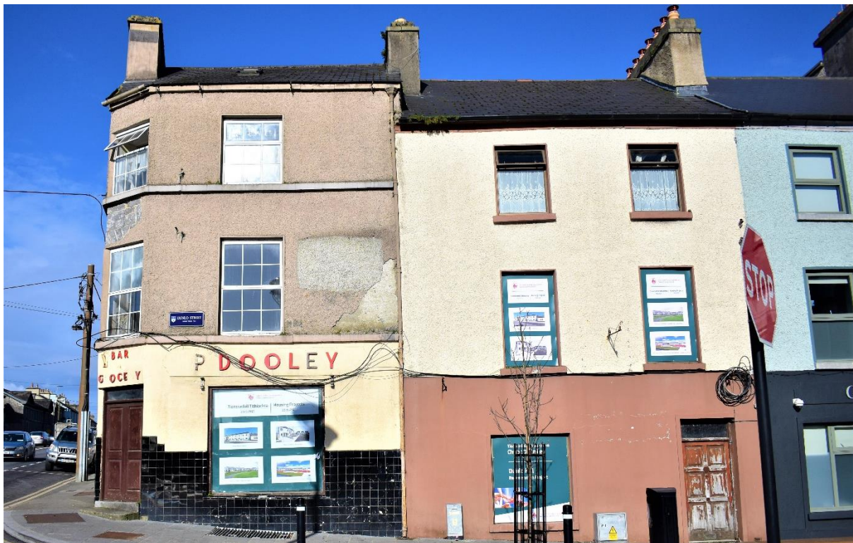
Figure 1. Shows the elevation facing Dunlo Street.
