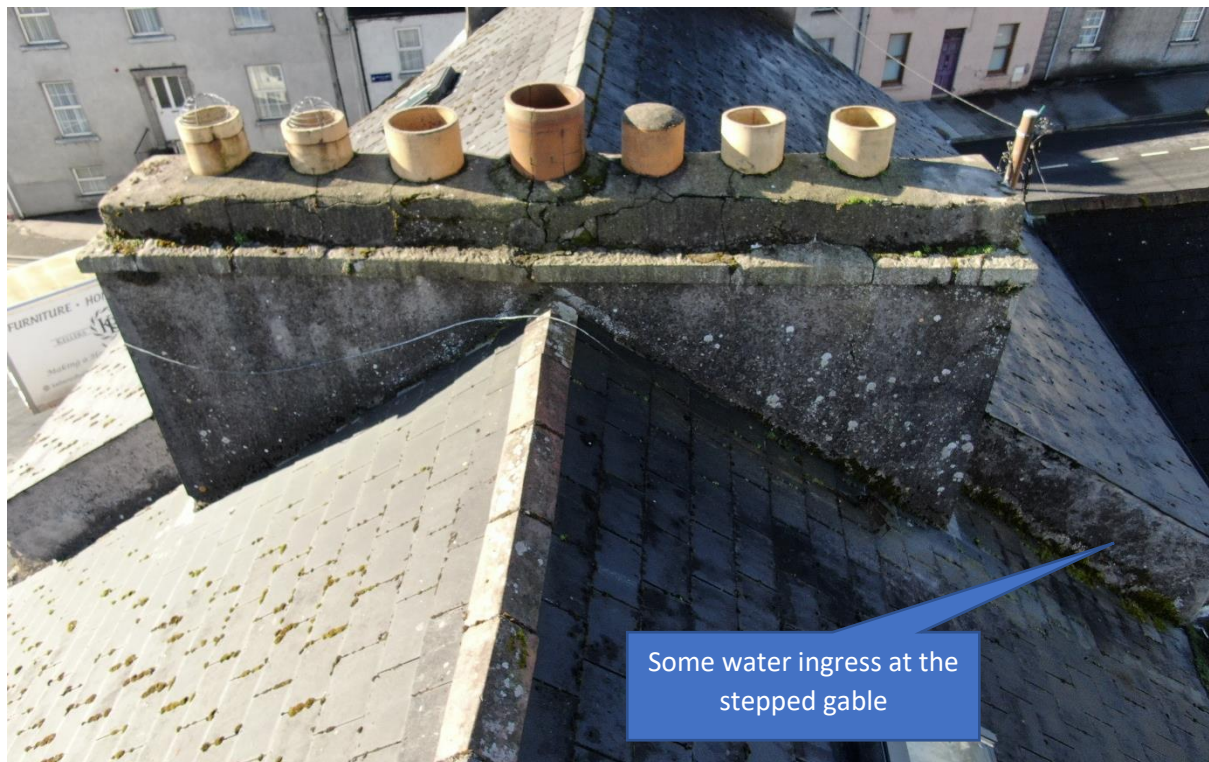
Figure 7. Shows an aerial view of the shared chimney.
