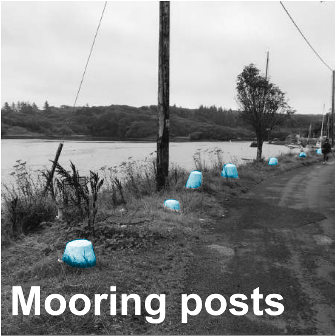
Painted granite bollards that are set back from quay, and some modern concrete bollards, are currently being used as mooring posts. The ropes across the grass bank introduce a tripping hazard for pedestrians.
