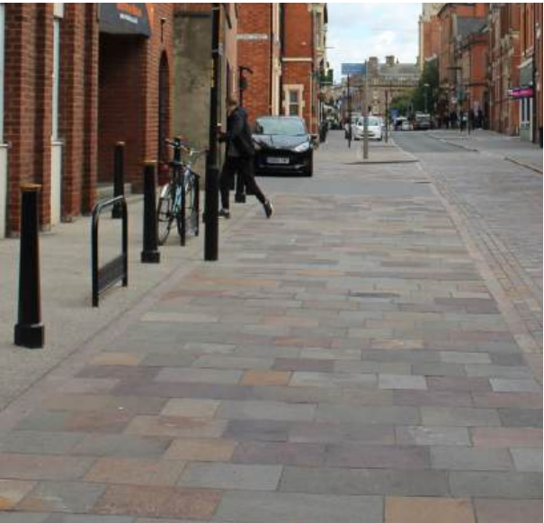
Natural stone paving to footway
