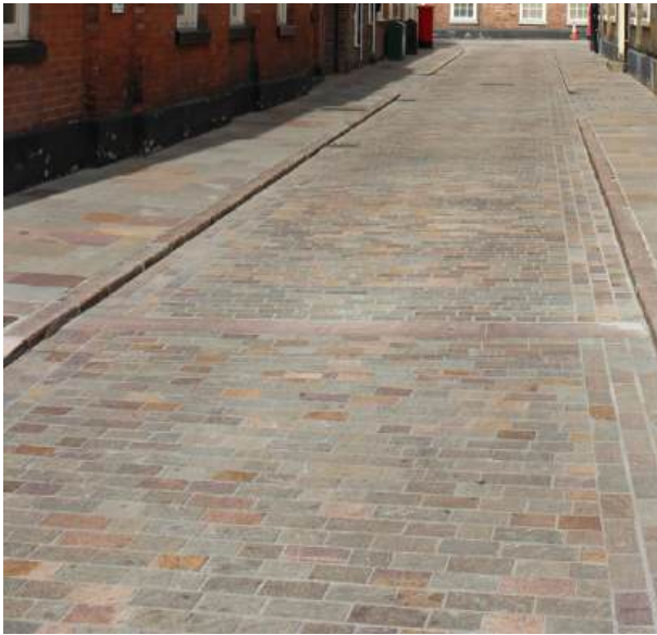
Natural stone setts to carriageway
