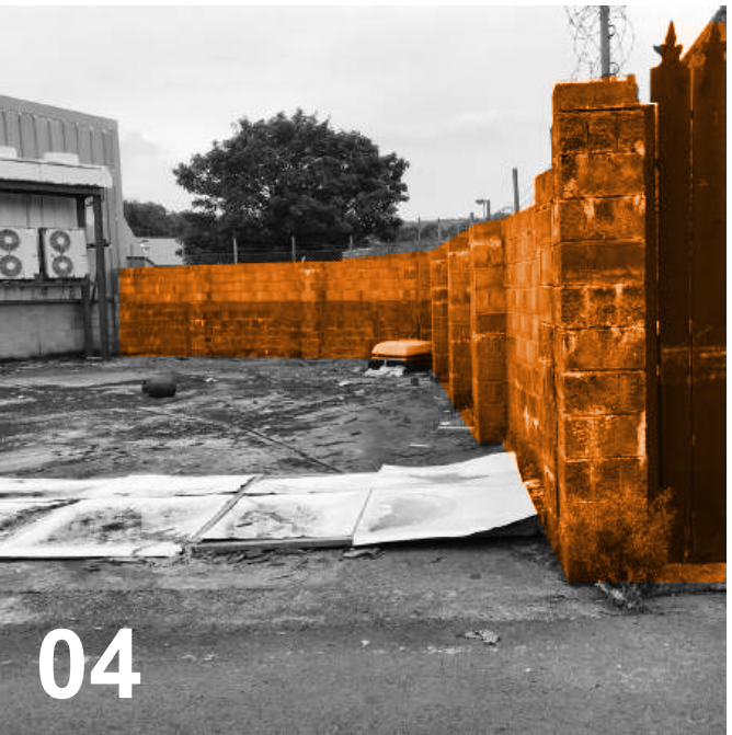
High walled boundaries between building plots create barrier to movement in various locations across the Town Centre.
