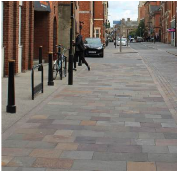
Natural stone paving to footway
