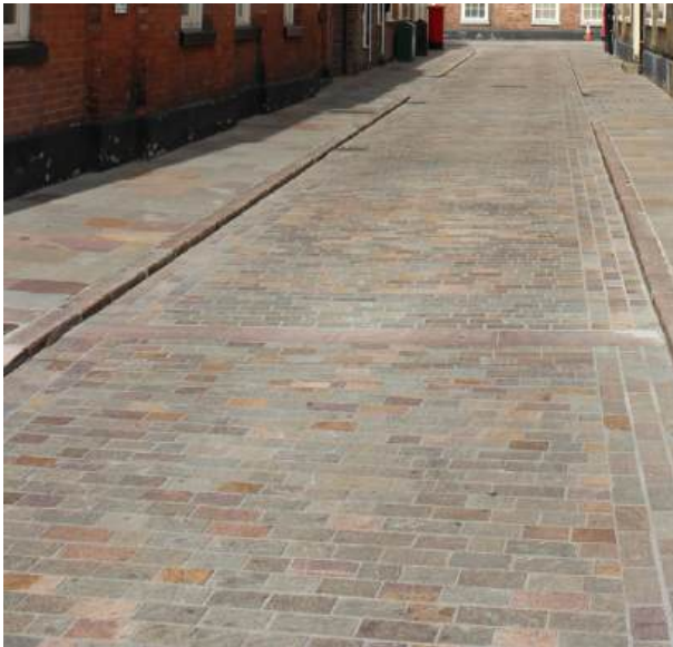
Natural stone setts to carriageway
