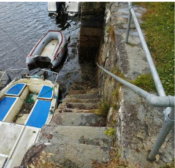
Existing Stone Wall retained
