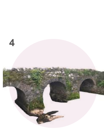
Ardber Old Bridge
