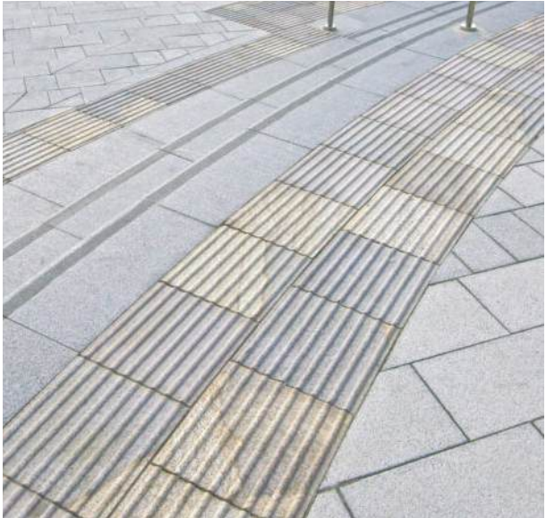
Natural Stone corduroy paving
