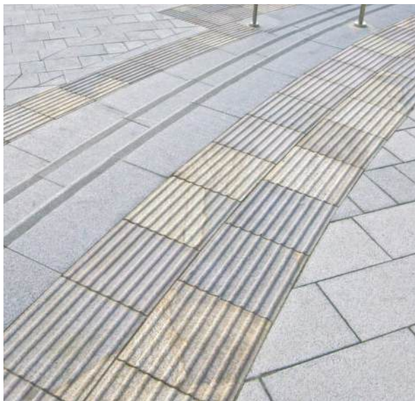
Natural stone corduroy paving
