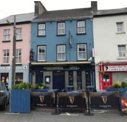
Existing active frontages along Main Street
