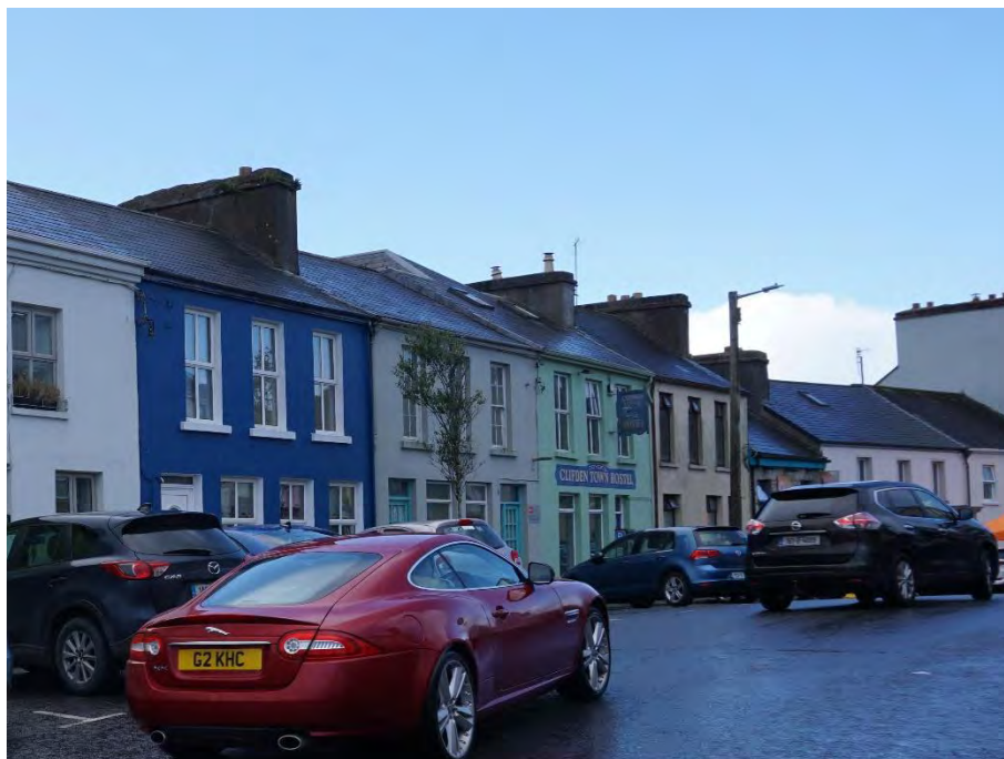
Photograph 23 - Terrace of Four Houses, Market Street
