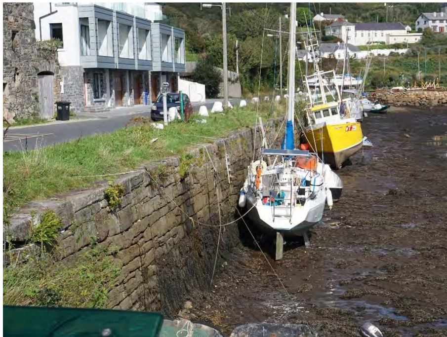
Photograph 7 - Quay/Wharf, Beach Road
