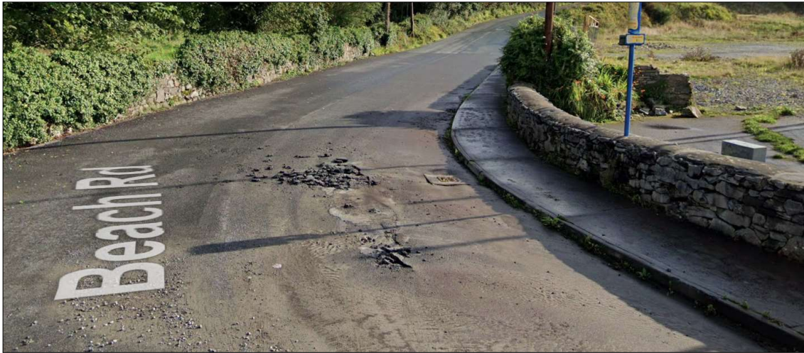
Figure 3-8 Beach Road culvert crossing
