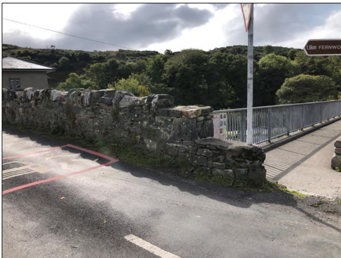
Plate 5-15 A small section of mapped Article 17 Annex I habitat [4010] Wet Heath overlaps with a section of the proposed works site, along Doonen Road to the southeast corner. The habitats recorded in this area includes Buildings and Artificial Surfaces. As such, this area does not conform to this Annex I habitat type [4010] Wet Heath
