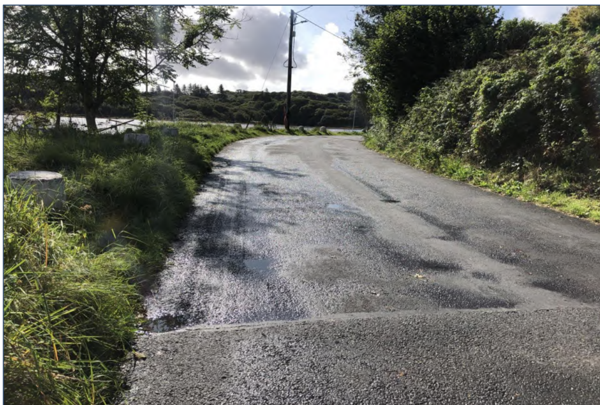
Plate 5-11 Hedgerow (WL1) recorded to the eastern boundary of Beach Road Quay, outside of the proposed works boundary.
