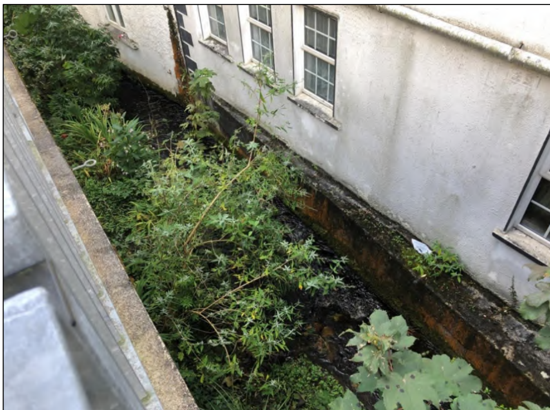
Plate 5-8 An artificially canalised section of an unmapped EPA watercourse, classified as an Eroding Upland River (FW1) runs culverted under Main Street in Clifden Town Centre to the northeast parcel of the proposed works site. This artificially canalised watercourse continues to flow adjacent to the eastern margin of the proposed works site, in a southerly direction before discharging into the Owenglin River after approx 280m, which at this point is designated as part of the Twelve Bens/Garraun Complex SAC.
