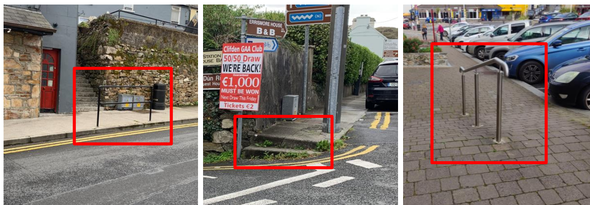
Figure 2-8: Existing Obstructed Regulatory Sign
