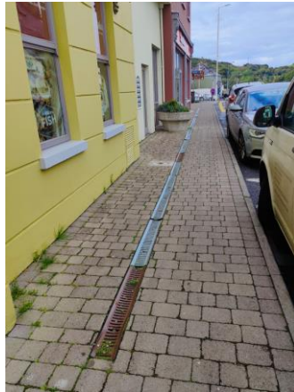
Figure 3-2 Existing Aco Drain
