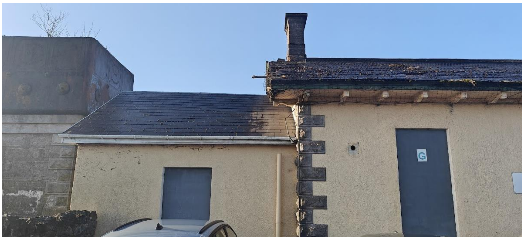
Plate 3-4: Netting covering fascia and roof.
