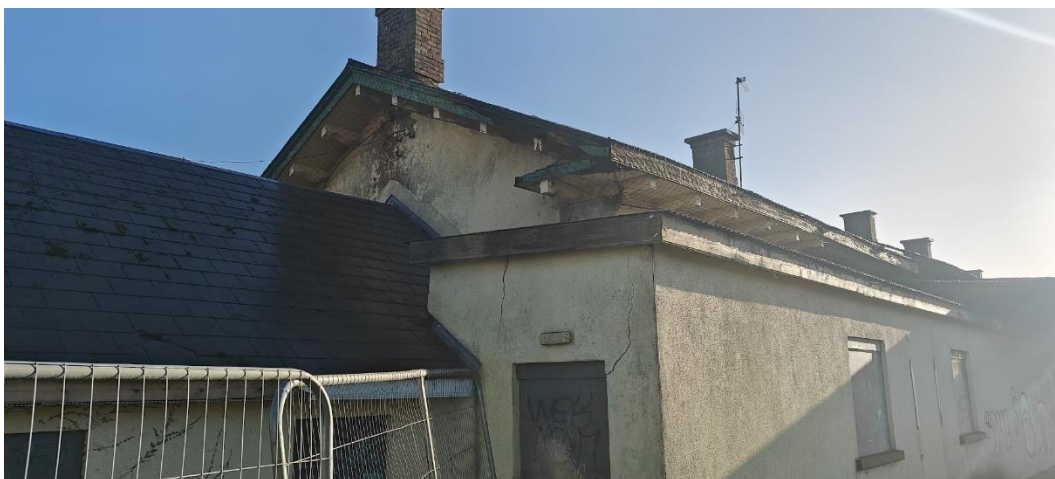
Plate 3-5: Rear gable with multiple potential access points
