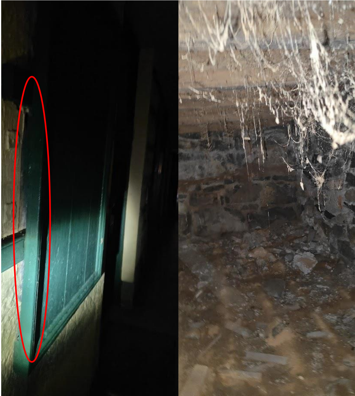
Plate 3-9 rear hallway with shutters. room
