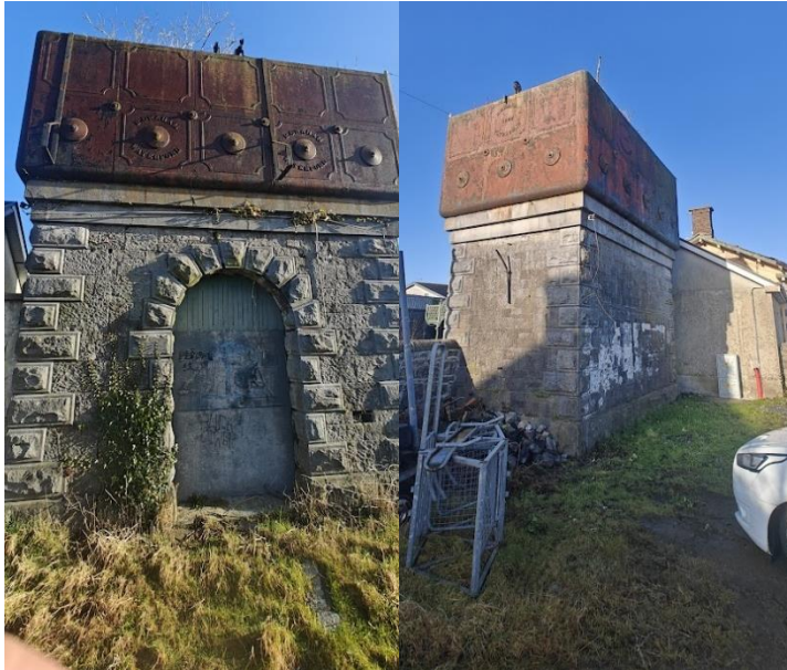
Plate 3-6 & Plate 3-7: Old water tower
