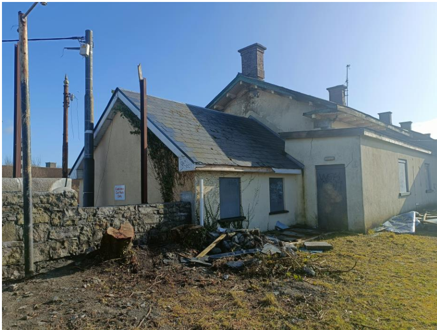
Plate 4: modern extension proposed for demolition
