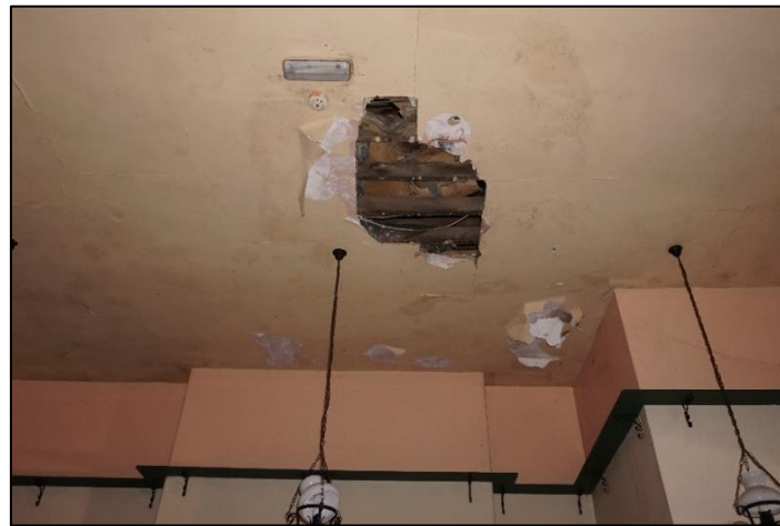
Photograph 9: View of modern plasterboard ceiling in the entrance hall
