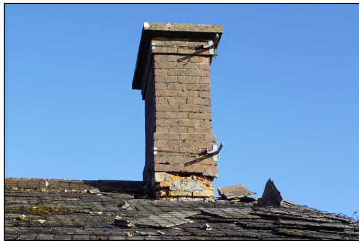
Photograph 1: View of the southern-most stack
