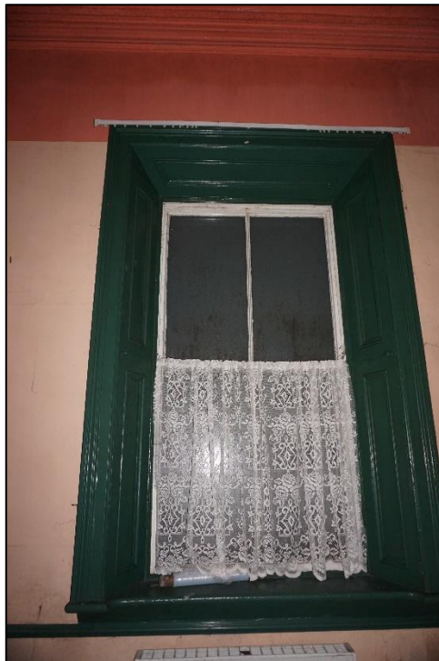
Photograph 7: View of an original timber sliding sash window assembly
