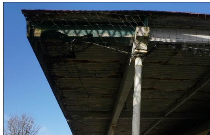
Photograph 4: View of lean-to structure
