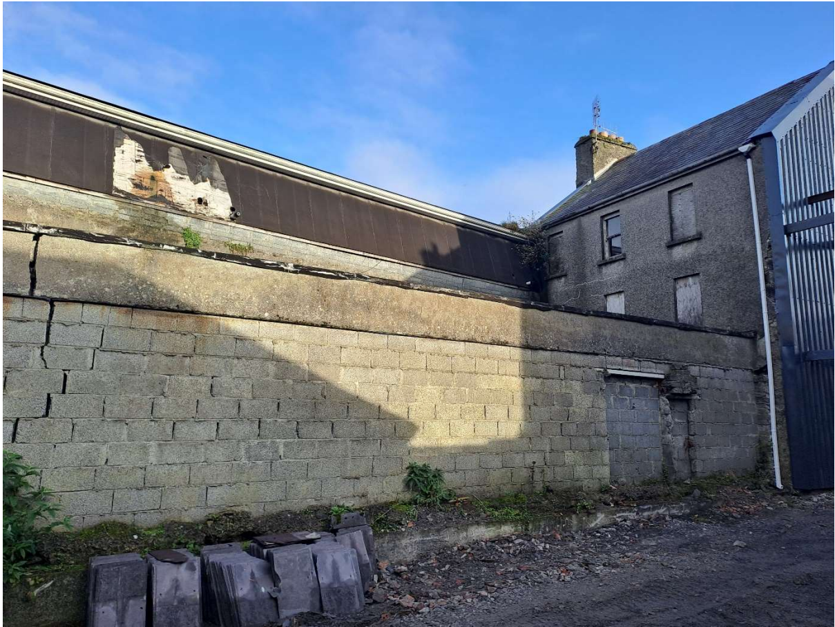
Figure 8- Single storey extension to rear to be demolished.
