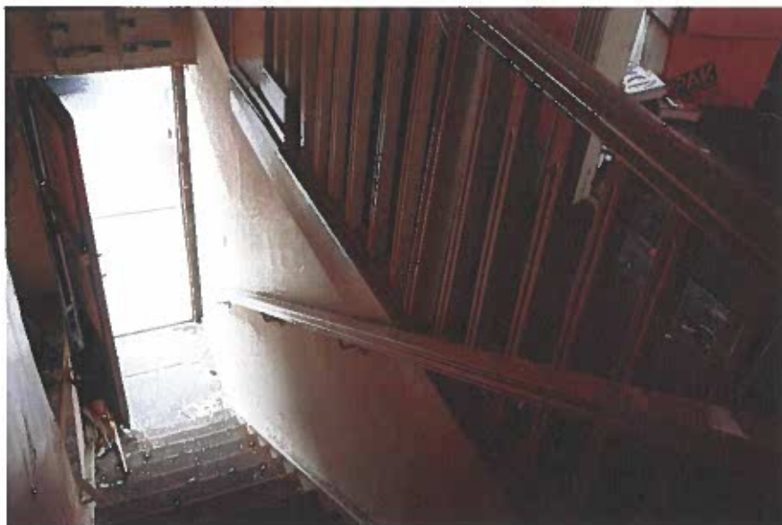
Photograph 26 View down the stair flight to the entrance door.
