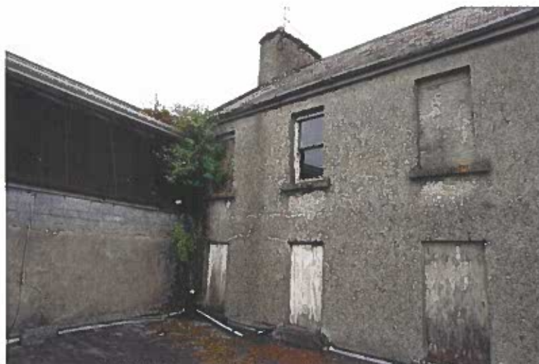
Photograph 24 Rear fenestration of building “B”.
