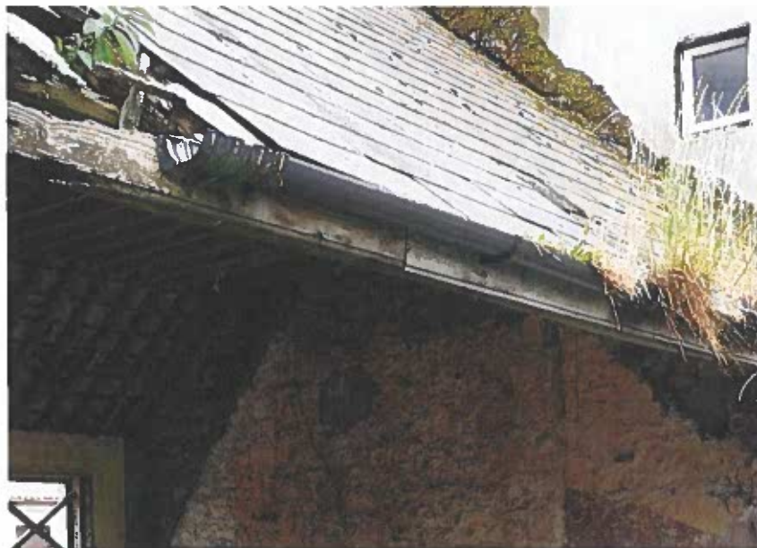
Photograph 9 Plastic guttering to rear roof eaves.
