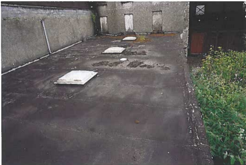
Photograph 18 Modern flat roof to the ground floor extension of the shop.
