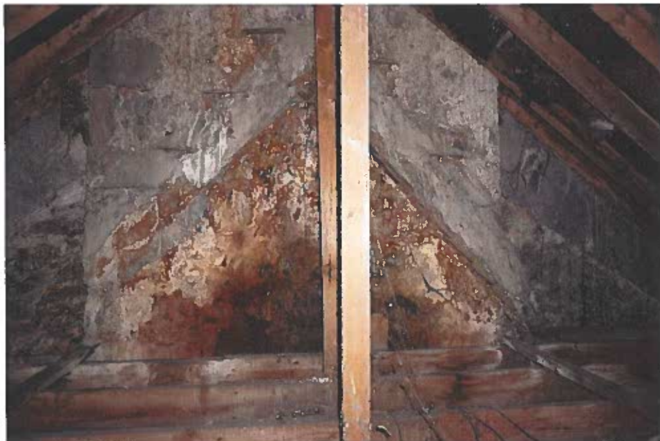
Photograph 13 View chimney system within the roof space.
