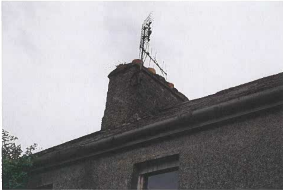
Photograph 19 View to eaves, rear of building "B" showing the gutters.
