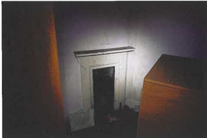
Photograph 15 Fireplace within first floor bedroom.
