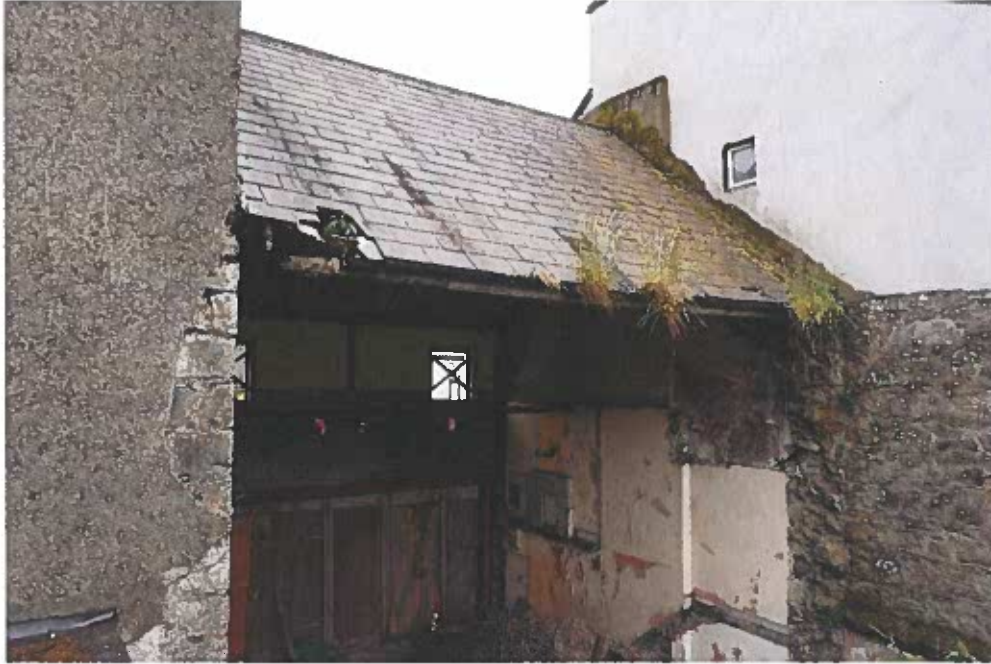
Photograph 10 General view into Building "A" with the structural walls on view.
