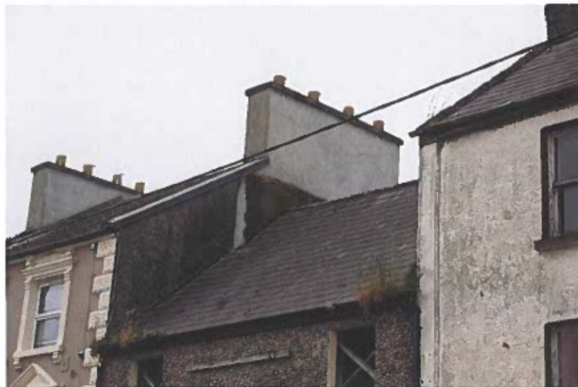
Photograph 4 Smooth Rendered Stack of the “Connaught Arms” serving Building “A”
