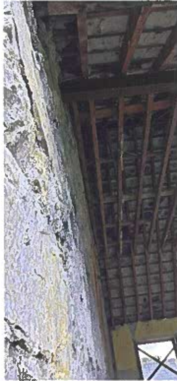
Photograph 8 View up to the roof structure of Building “A”. Note surviving lime parging.
