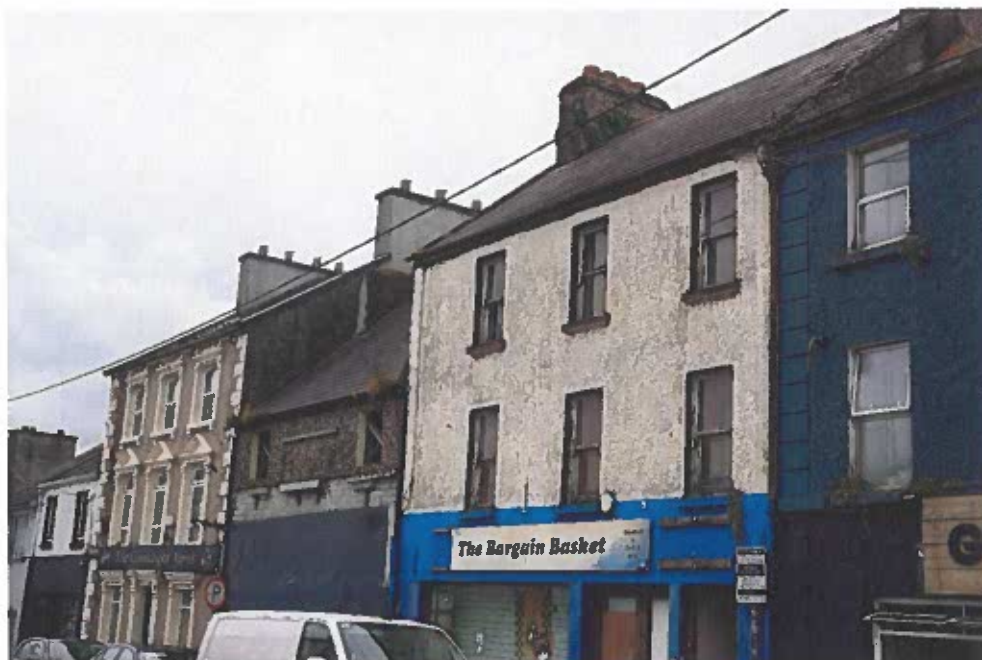
Photograph 1 - View of Subject Structures, Building A to Left, Building B (The Bargain Basket) to Right
