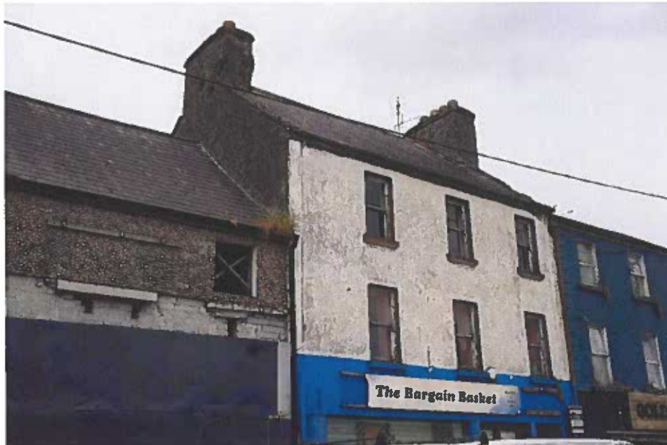
Photograph 12 General view up to the chimney stacks from the street.
