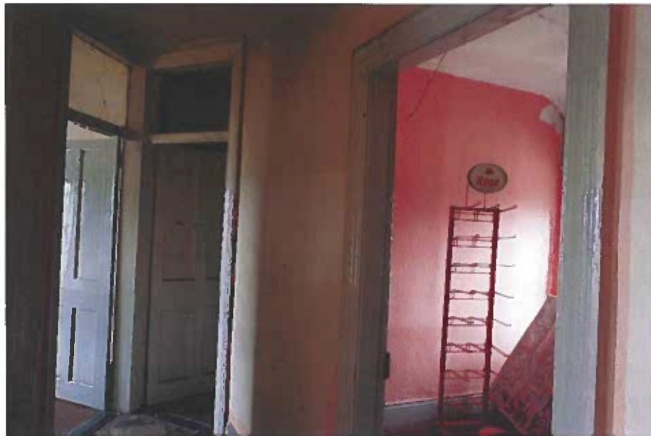
Photograph 21 First floor hallway. Partition walls to the bedrooms.
