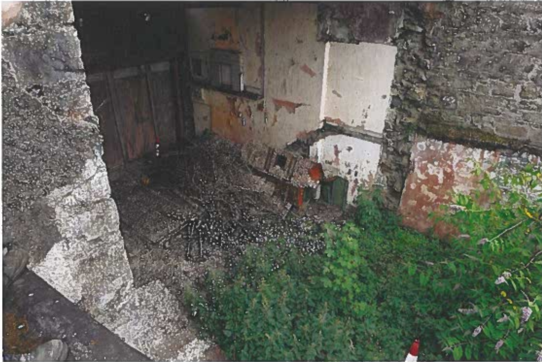
Photograph 11 View to the ground floor of Building “A”.
