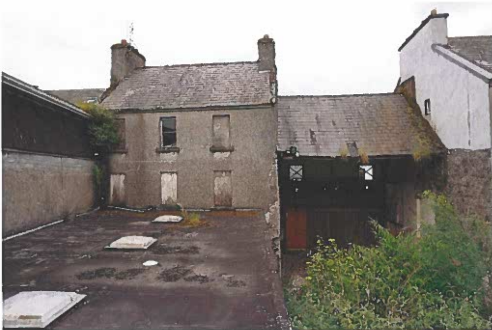
Photograph 2 - Rear Elevation of Building B (Left) and Building A (Right)
