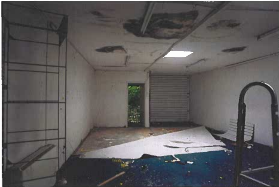
Photograph 25 View to the rear of the ground floor of building "B", with the floor finish pulled back revealing the concrete floor.
