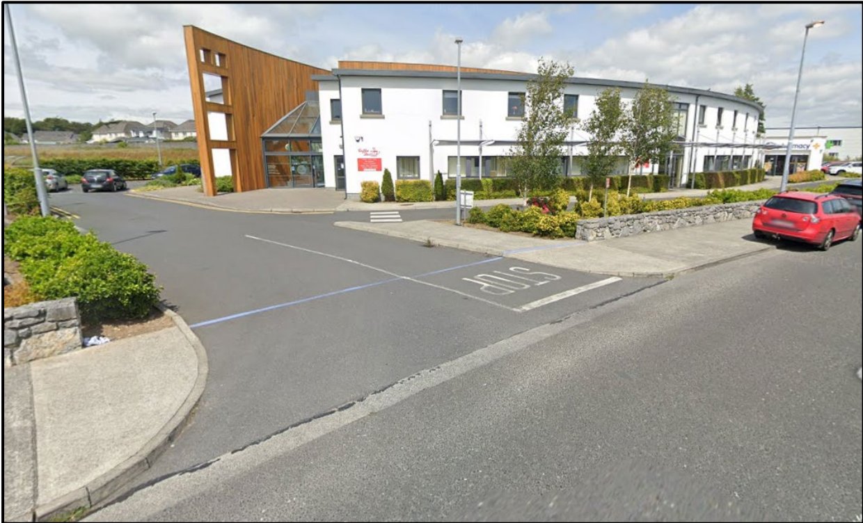
Figure 3.9: Pedestrian infrastructure at the entrance to the Athenry Primary Care Centre and Pharmacy on the Gort Mhaolir Road. (Source: Google Earth, Street View).
