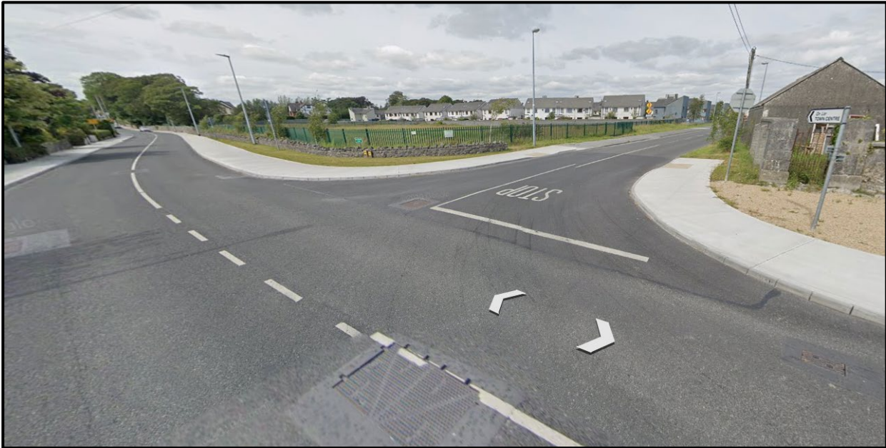
Figure 3.6: Gort Mhaolir Estate Road/L-3103 Junction. Approach from south (Source: Google Earth, July 2019)
