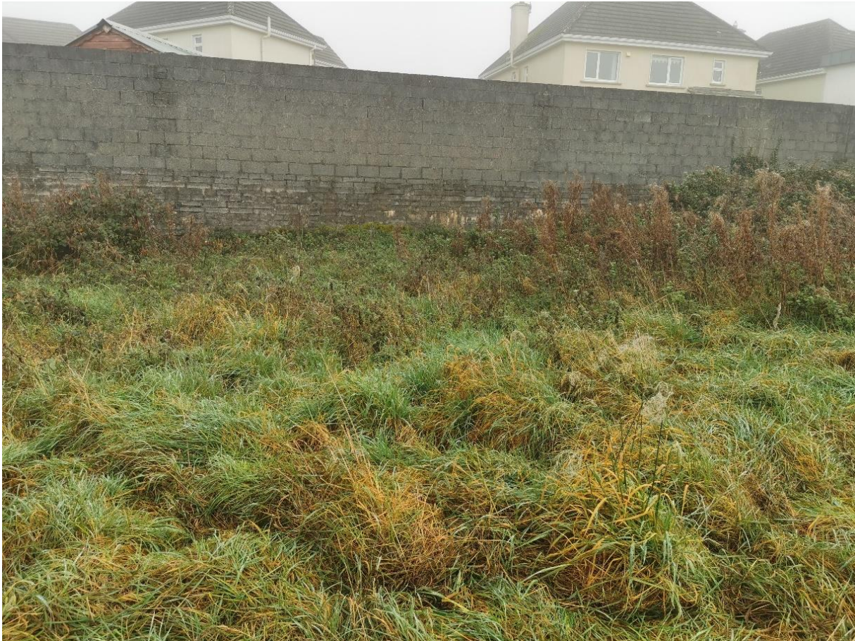
Figure 4-2: Example of brick wall bordering the site
