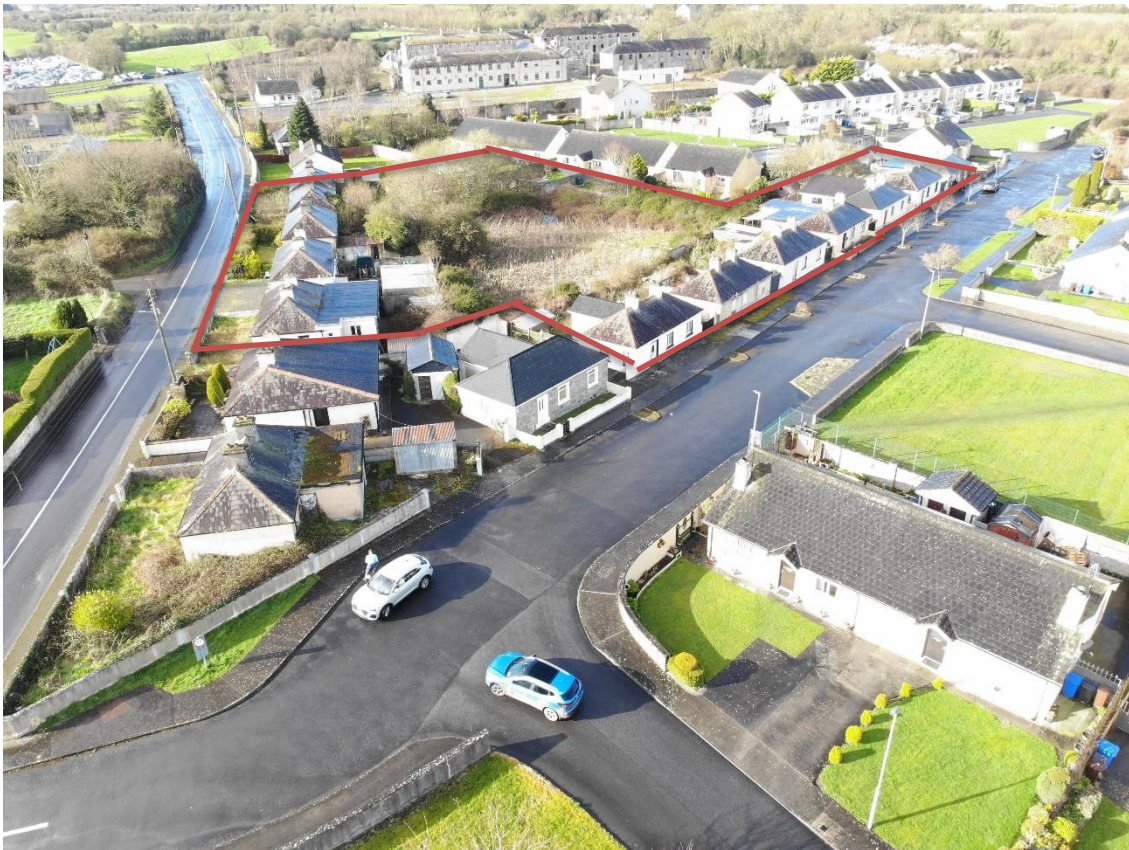
Photo of the Site
