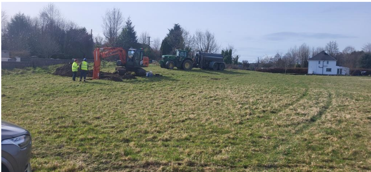
Plate 1-4 Site investigation trial holing being carried out in March 2025.
